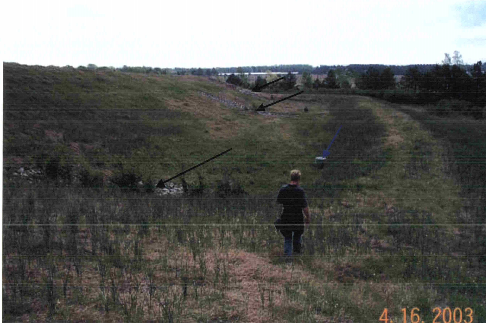
Photo 20: View of sedimentation basin at the south end of the OU1 landfill. View is to the east. Rock lined structures (black arrows) are letdown channels. Metal structure (blue arrow) is drainage pipe for the sedimentation basin.
