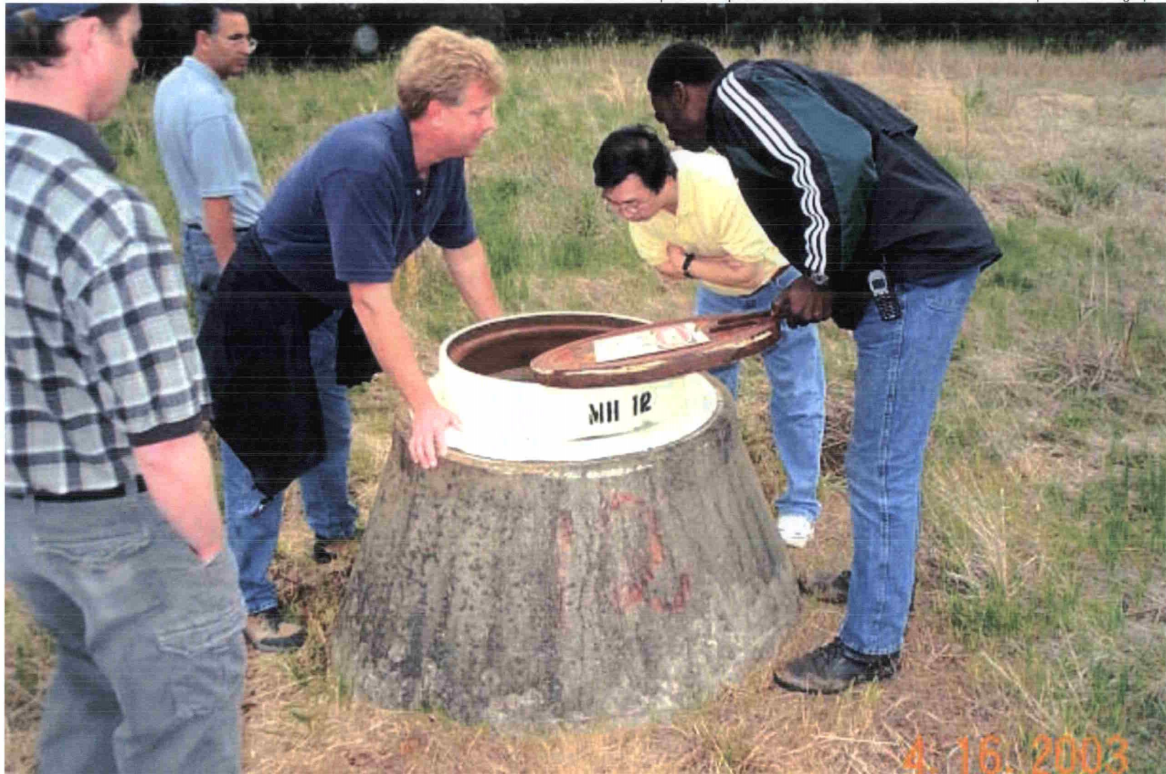
Photo 37: View of Manhole 12 of the french drain system. Manhole cover has been removed for inspection.
