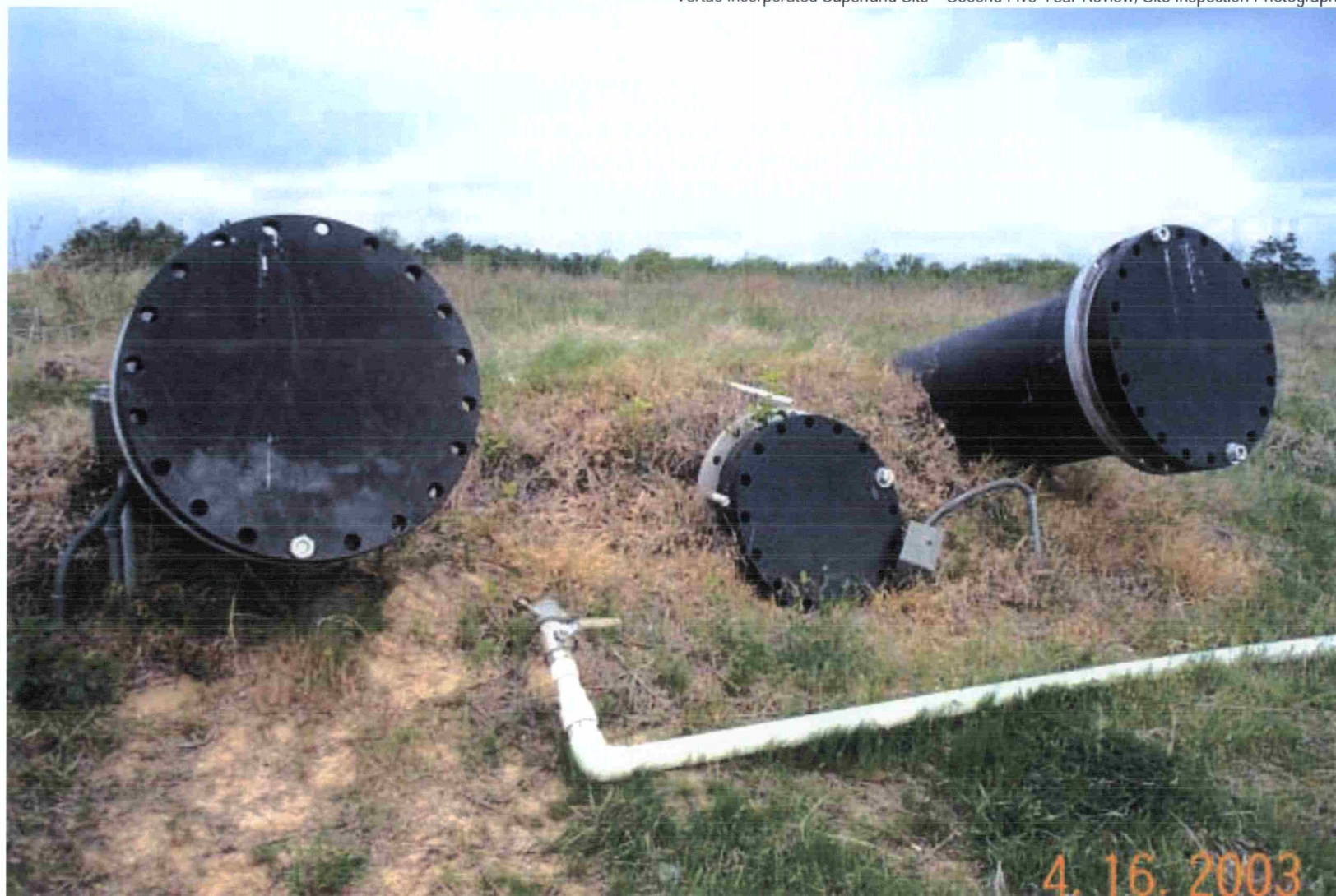
Photo 23: Access outlets for leachate collection and leachate detection sumps at the OU1 landfill.
