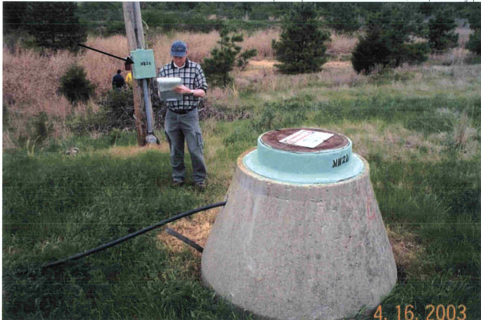
Photo 12: View of Manhole 2A of the french drain. The manhole contains a sump and pump to collect and remove leachate. The controller box for the pump and leachate level detector system is mounted on the pole in the background (at arrow).
