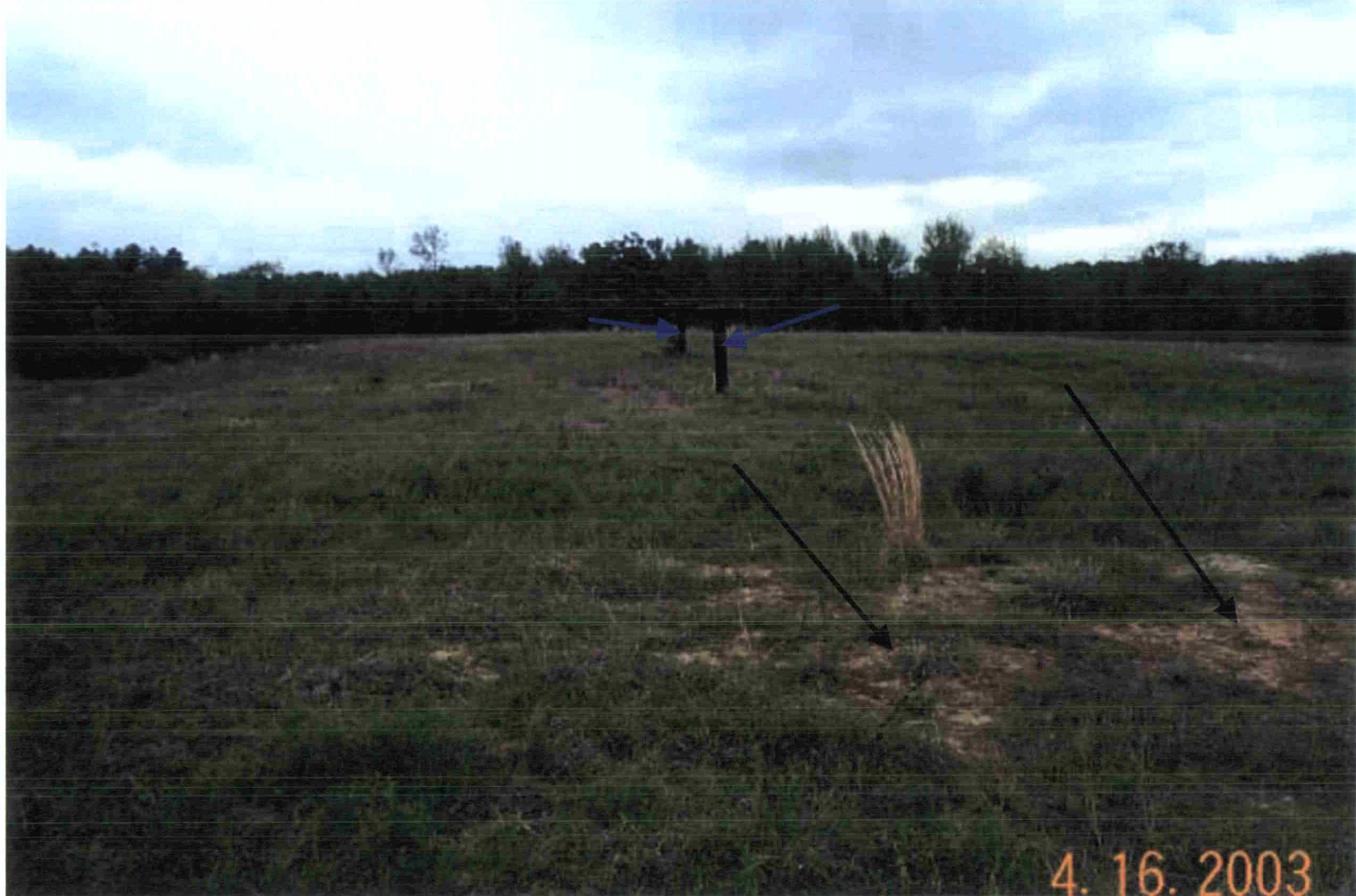
Photo 29: View of the top of the cap at the OU1 landfill. Note area of sparse vegetation (black arrow). Blue arrows are pointing to passive gas vents.
