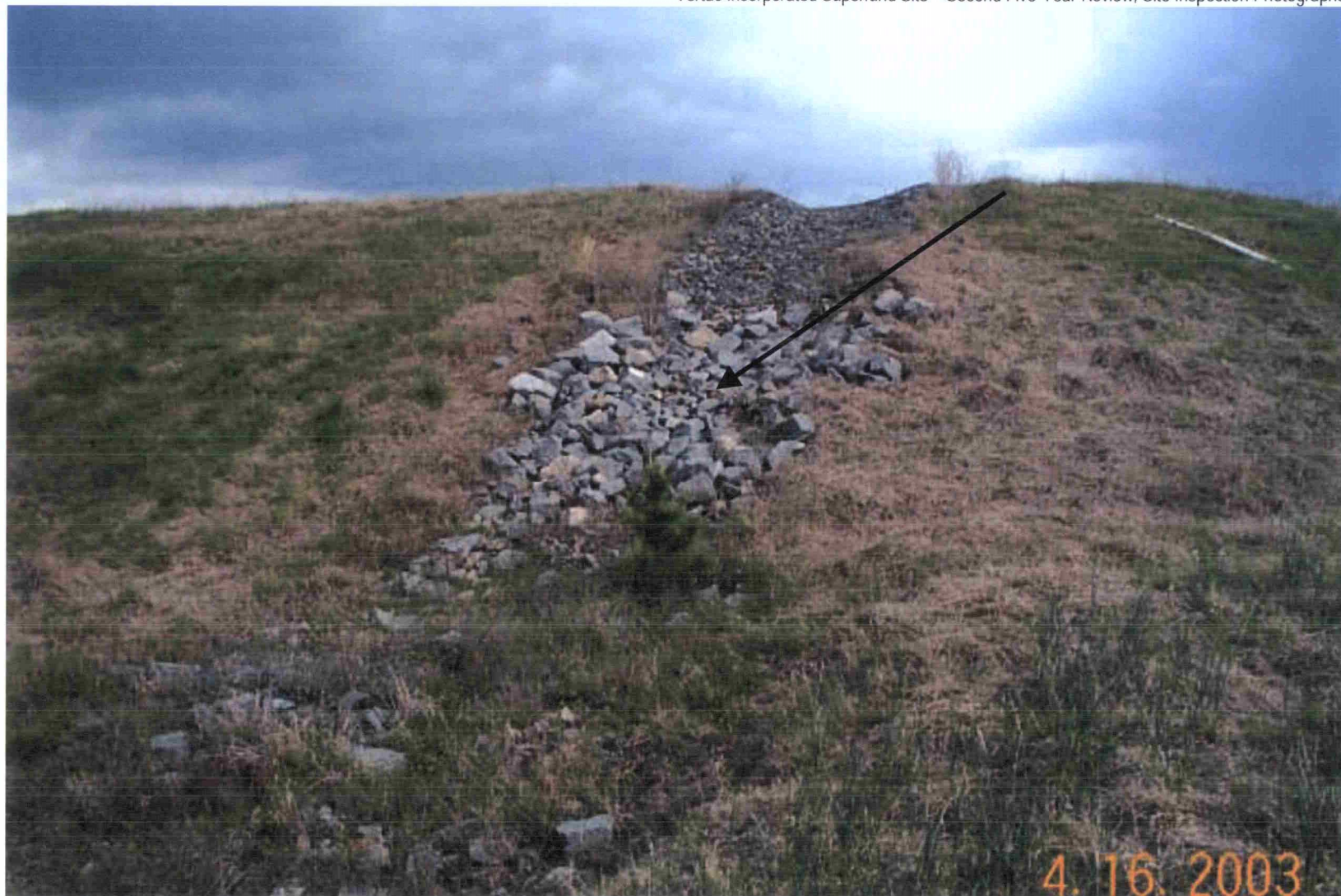
Photo 21: View of rock lined letdown channel (at arrow) at the OU1 landfill. These channels drain water from the top of the landfill cap. Note small tree growing along letdown channel in the center foreground.
