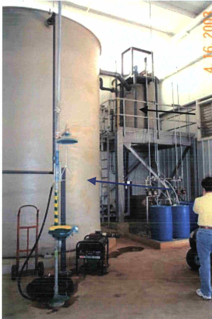
Photo 50: View inside Wastewater Treatment Plant. The large tank on top of the platform in the rear is the pH neutralization tank (black arrow). The tank to the left is the treated water tank (blue arrow).
