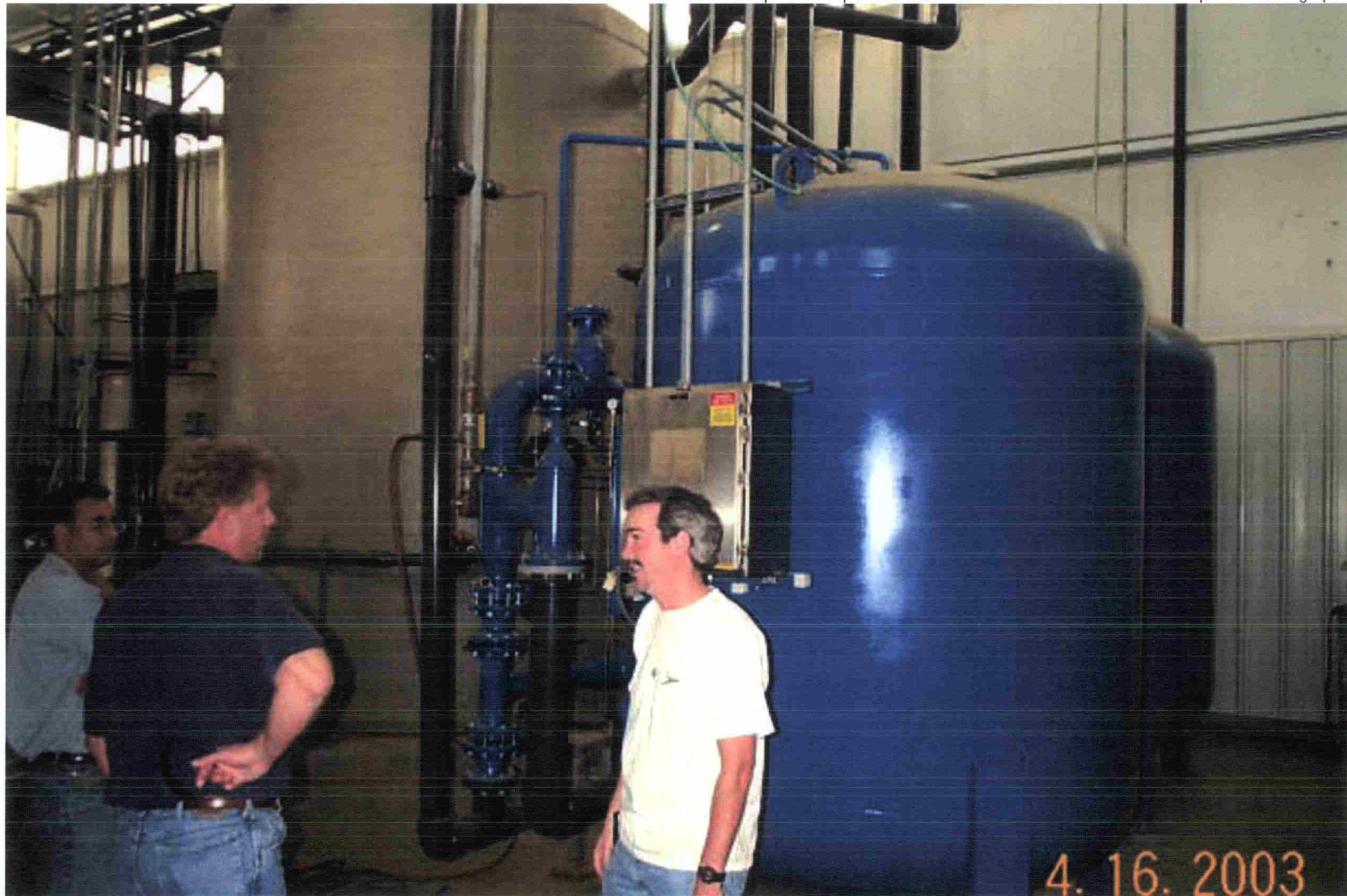
Photo 48: View inside Wastewater Treatment Plant. The two large blue tanks are the sand filters.
