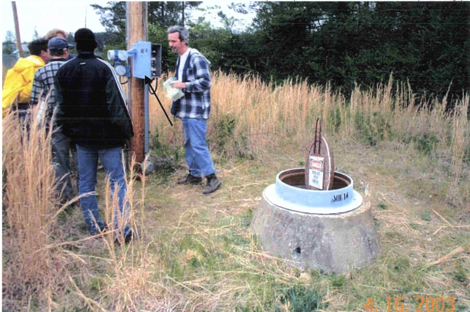
Photo 38: View of Manhole 14 of the french drain system. Manhole cover has been removed for inspection. The controller box for the pump and leachate level indicator are mounted on the pole at left (arrow).
