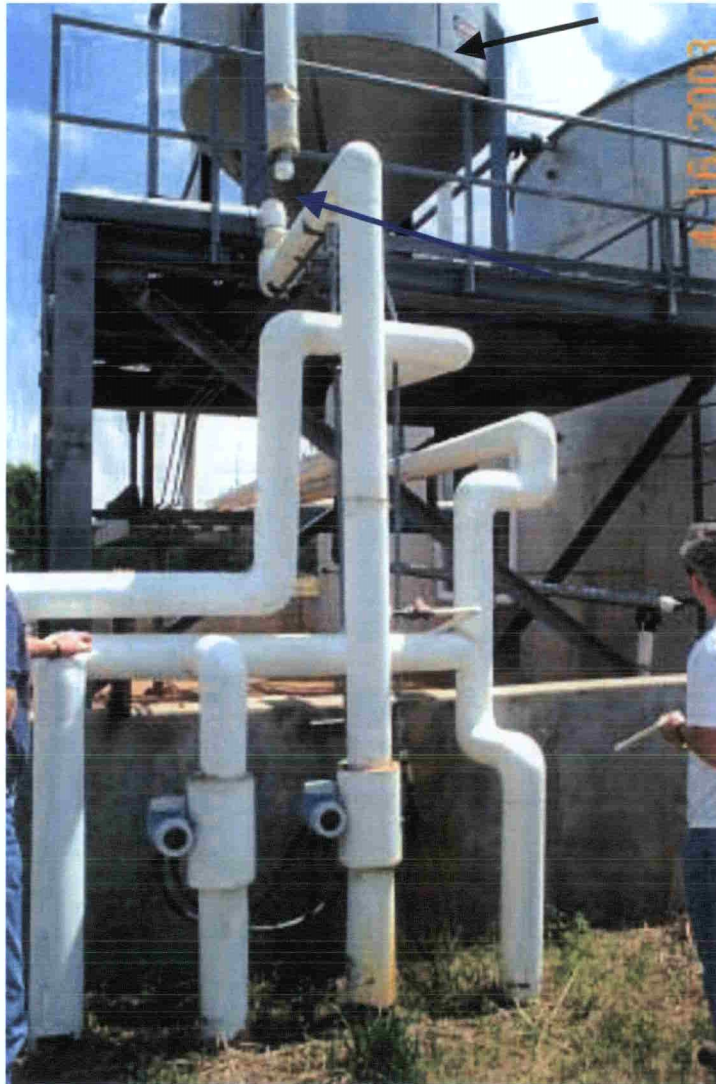
Photo 45: View of inlet pipes from french drain and ground water extraction systems at the waste Wastewater Treatment Plant. Tank at top of photo is the oil/water separator (black arrows). Note that the inlet pipes are no longer connected to the oil/water separator (blue arrow).
