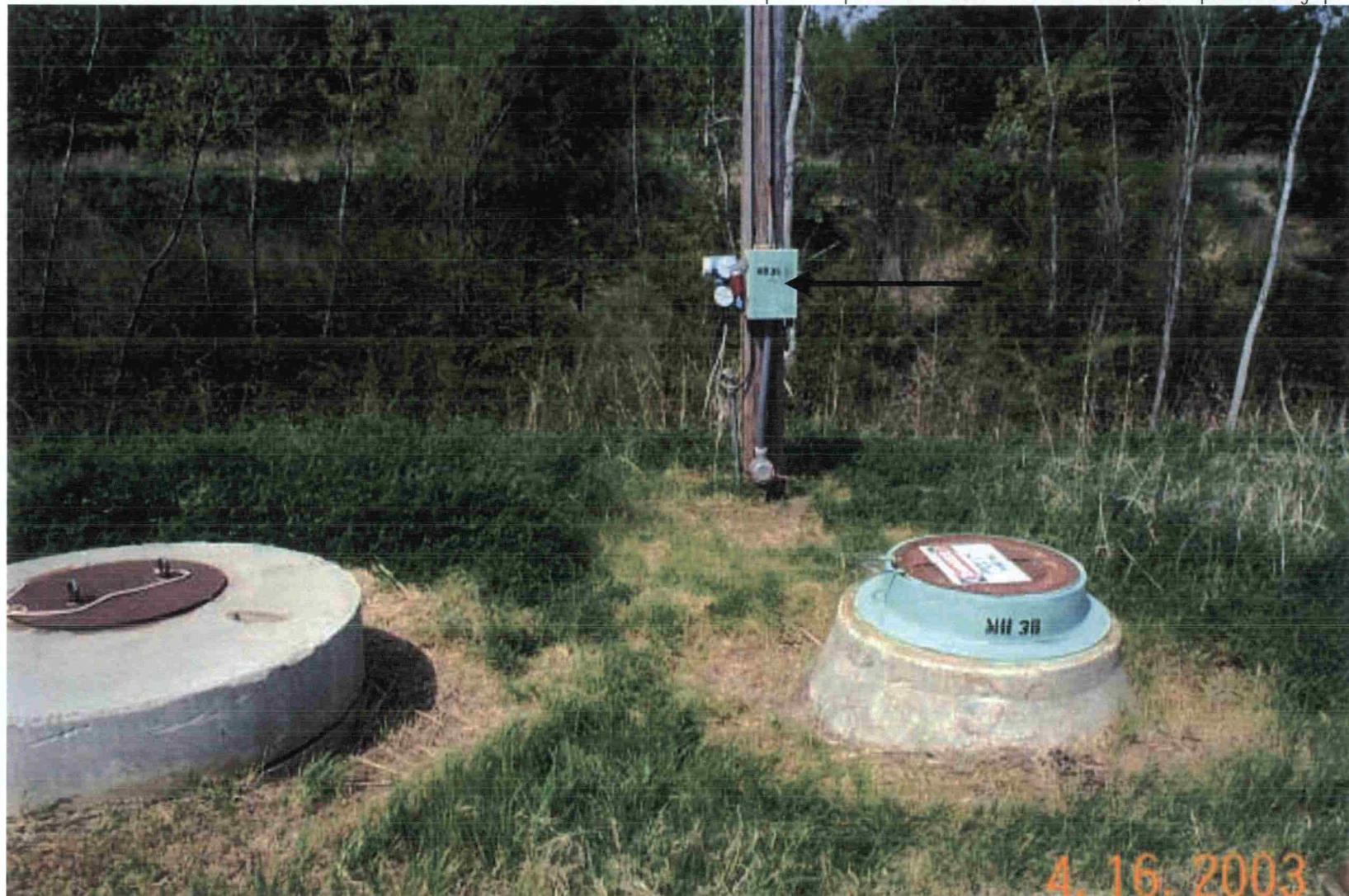
Photo 44: View of Manhole 3B of the french drain. The controller for the leachate level indicator and pump is on the pole behind the manhole (black arrow).
