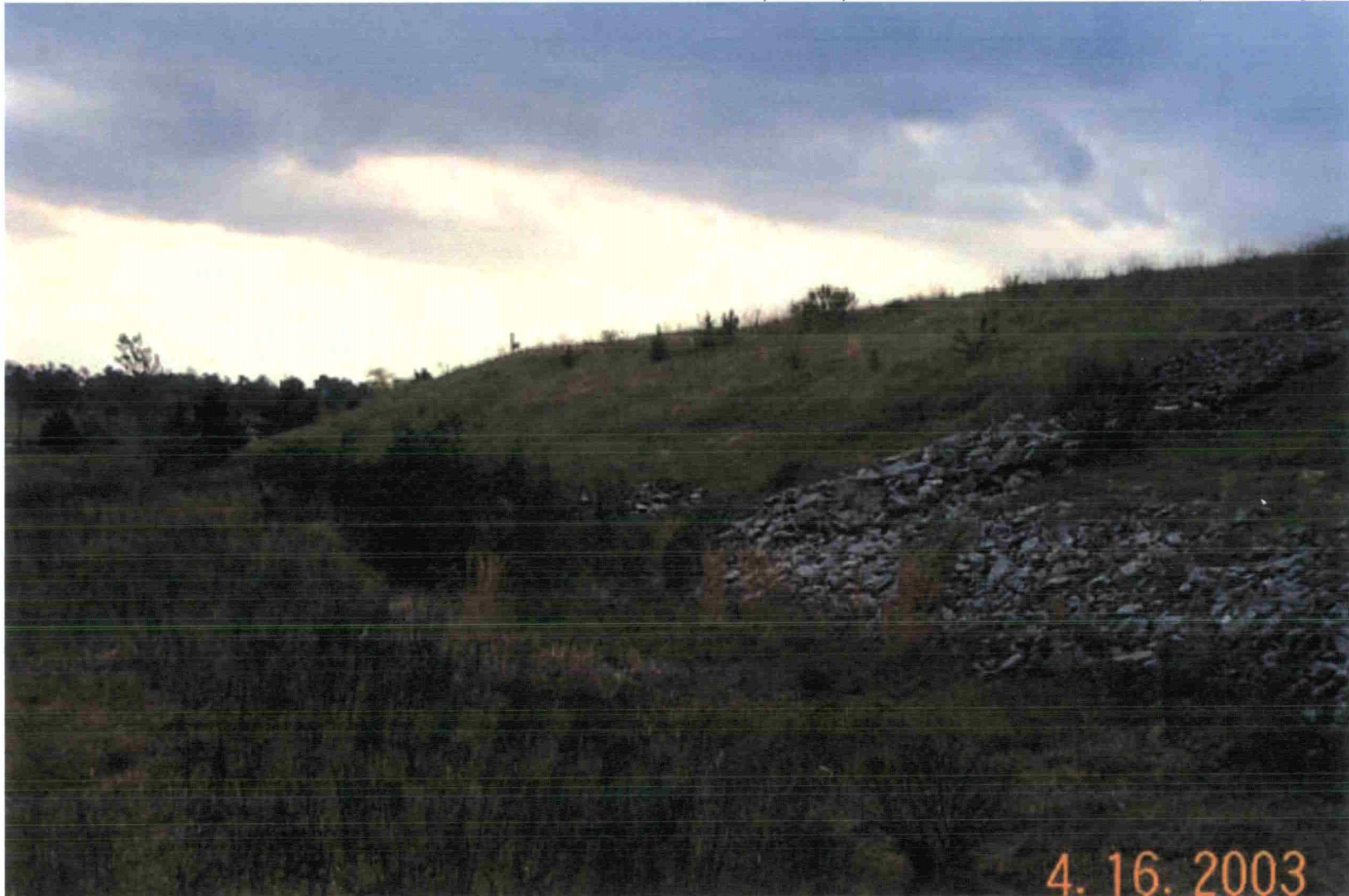
Photo 25: View of the east side of the OU1 landfill. View is facing south. Note small trees growing on the cap.
