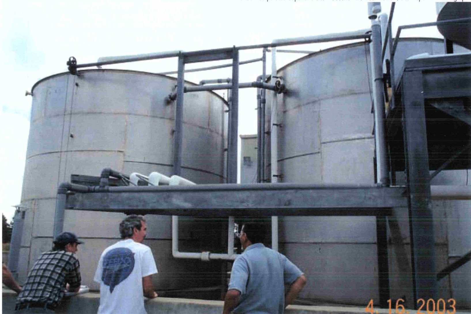
Photo 46: View of equalization tanks outside the Wastewater Treatment Plant. Tanks store contaminated water and leachate prior to treatment.
