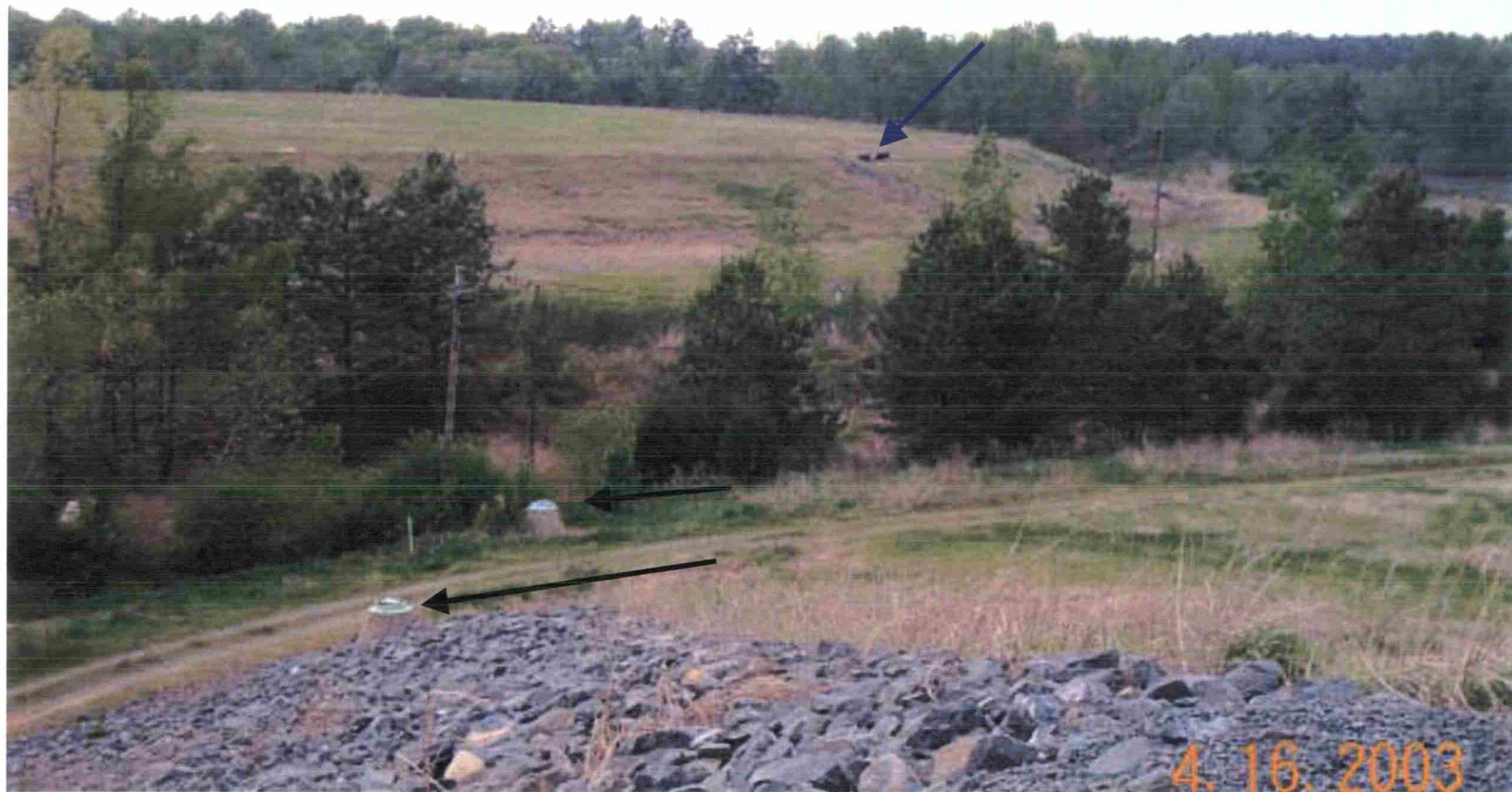
Photo 9: View of the OU1 landfill from Mt. Vertac. View is to the northwest. Two sumps for the french drain are visible in the foreground (black arrows). The leachate collection and detection system sumps are visible on the landfill (blue arrow).
