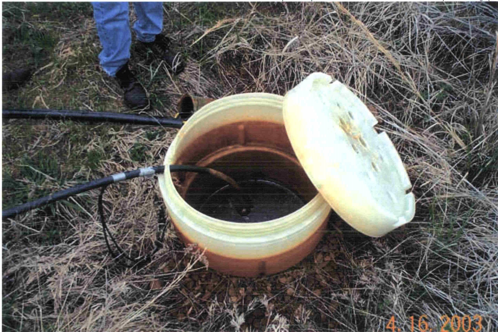
Photo 13: View of leachate sump installed in former cooling pond. This sump is located west of the french drain and east of the OU1 landfill.
