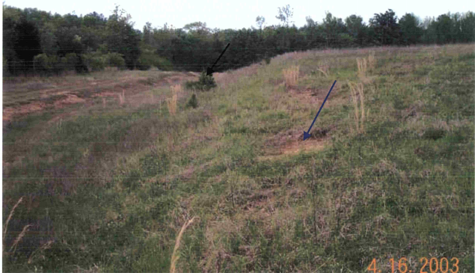
Photo 30: View of the west side of the OU1 landfill. View is facing north. Note small trees growing on the cap (black arrow) and area of sparse vegetation (blue arrow).
