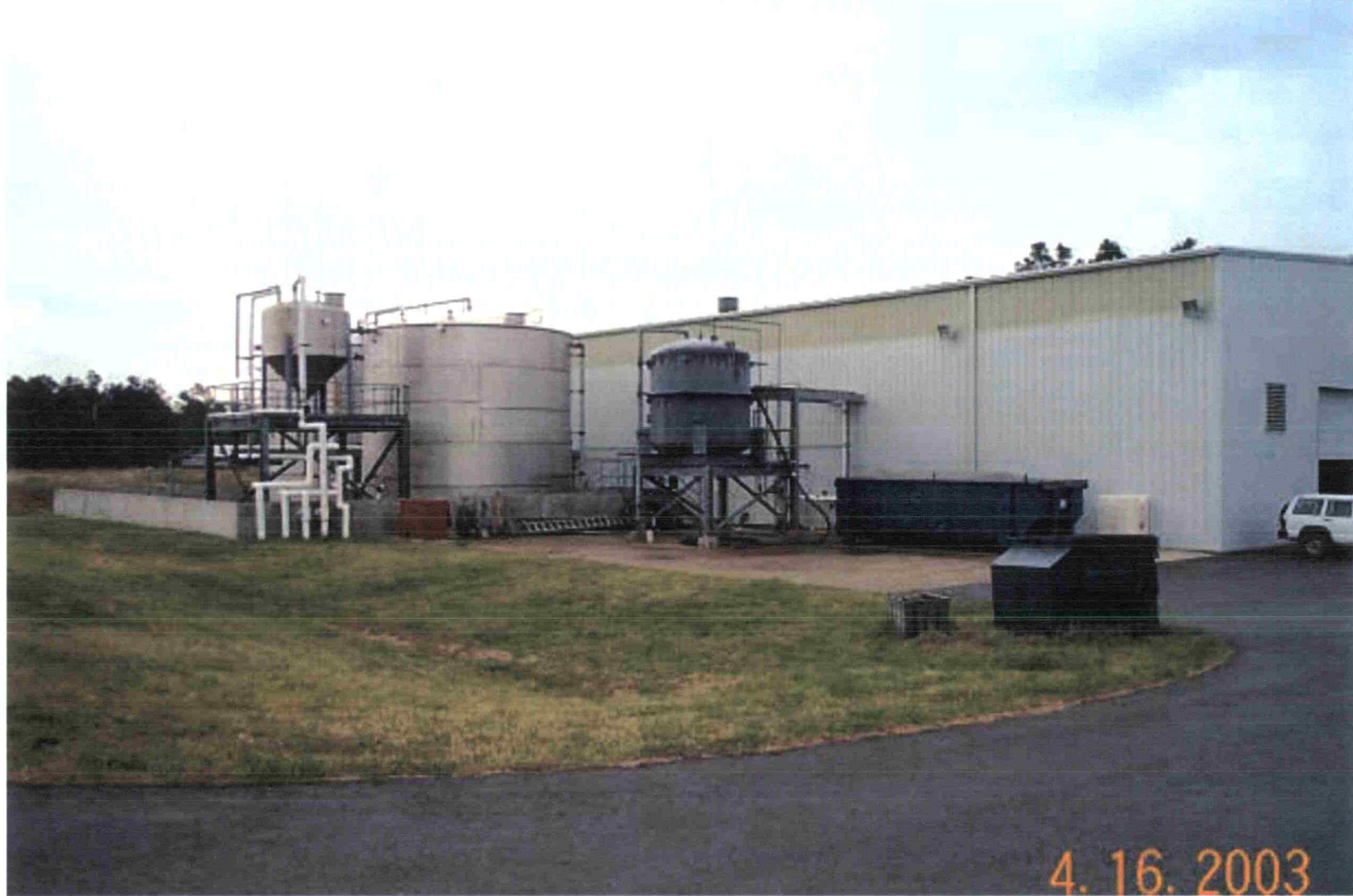
Photo 1: View of Wastewater Treatment Plant, facing southeast. Two large tanks contain untreated water from the french drain and ground water extraction systems.
