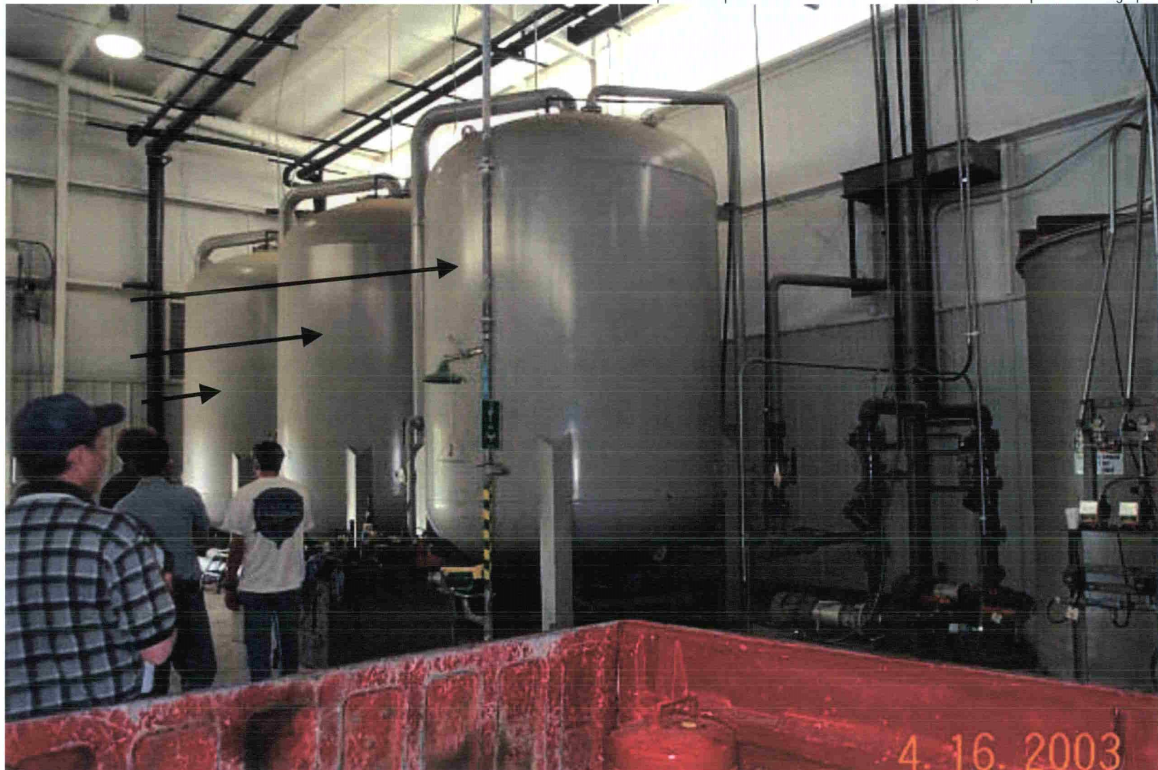
Photo 49: View inside Wastewater Treatment Plant. The three large tanks are the carbon treatment units (black arrows).
