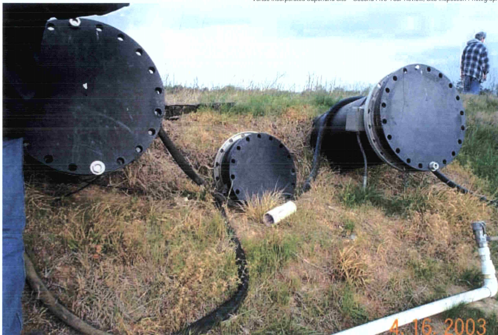
Photo 24: Access outlets for leachate collection and leachate detection sumps at the OU1 landfill.
