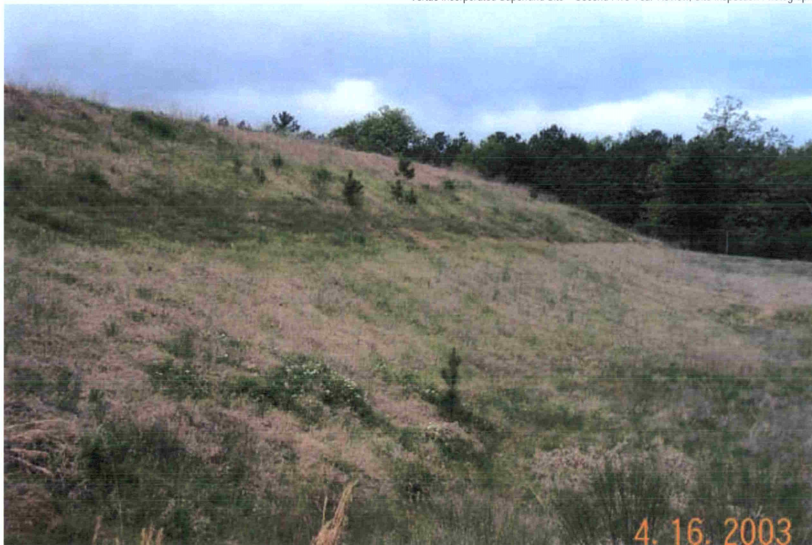
Photo 26: View of the north side of the OU1 landfill. View is facing west. Note small trees growing on the cap.
