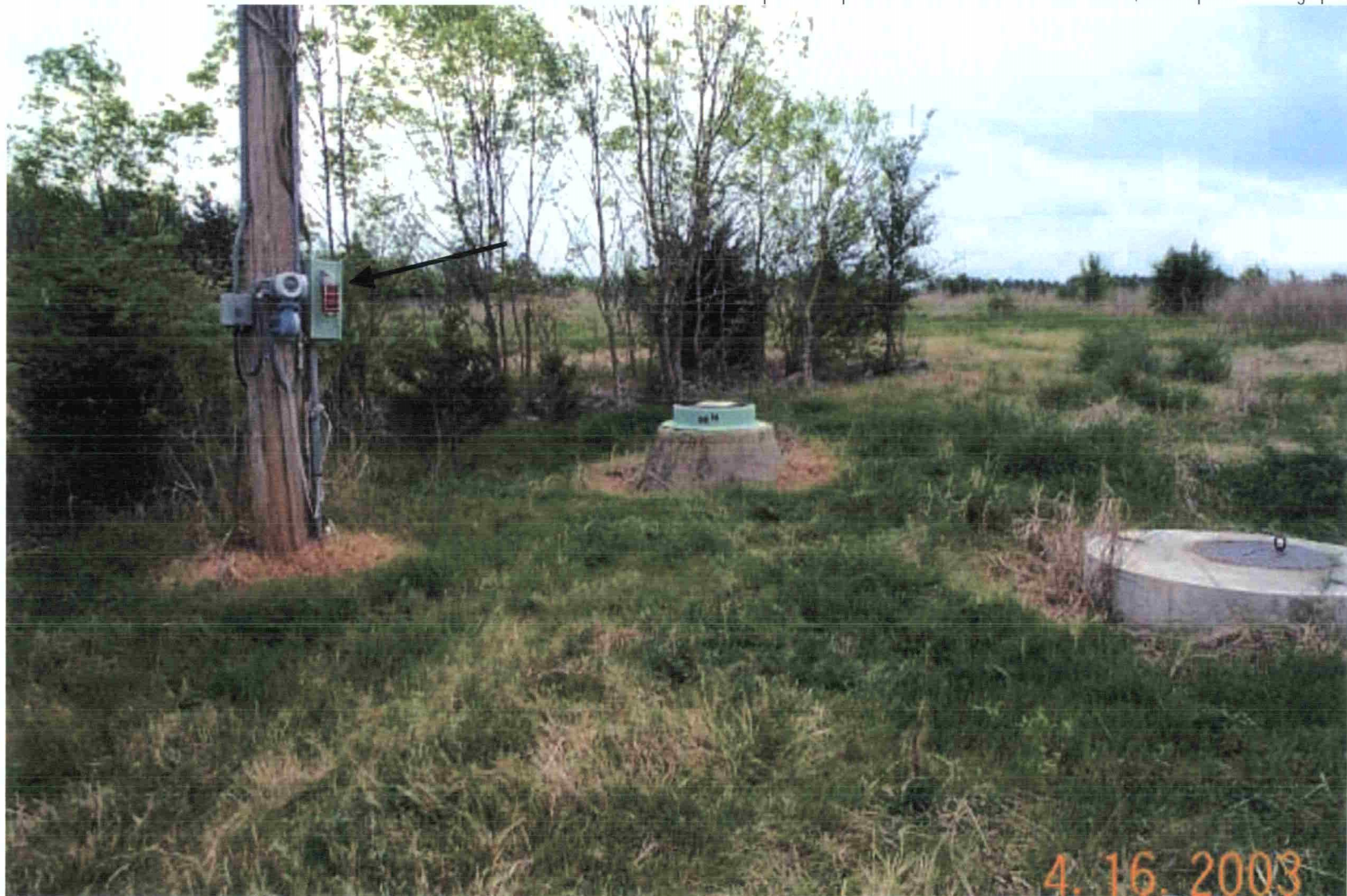
Photo 15: View of a french drain manhole. Controllers for pump and leachate level detectors are mounted on the pole to the left (arrow).
