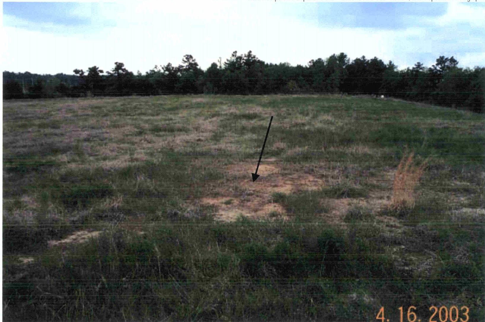
Photo 28: View of the top of the cap at the OU1 landfill. Note area of sparse vegetation (black arrow).
