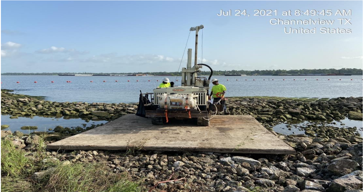
Photo 7 Drill crew collecting soil cores at boring location SJSB099.
