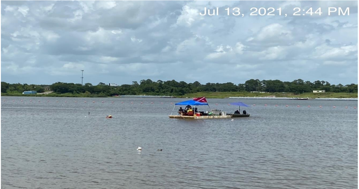
Photo 3 Dive crew clearing the rock cap at various boring locations prior to drilling activities.
