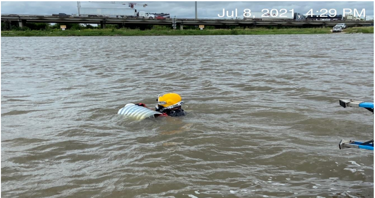
Photo 2 View from airboat. Diver installing a culvert pipe after clearing the rock cap at boring location SJSB104.
