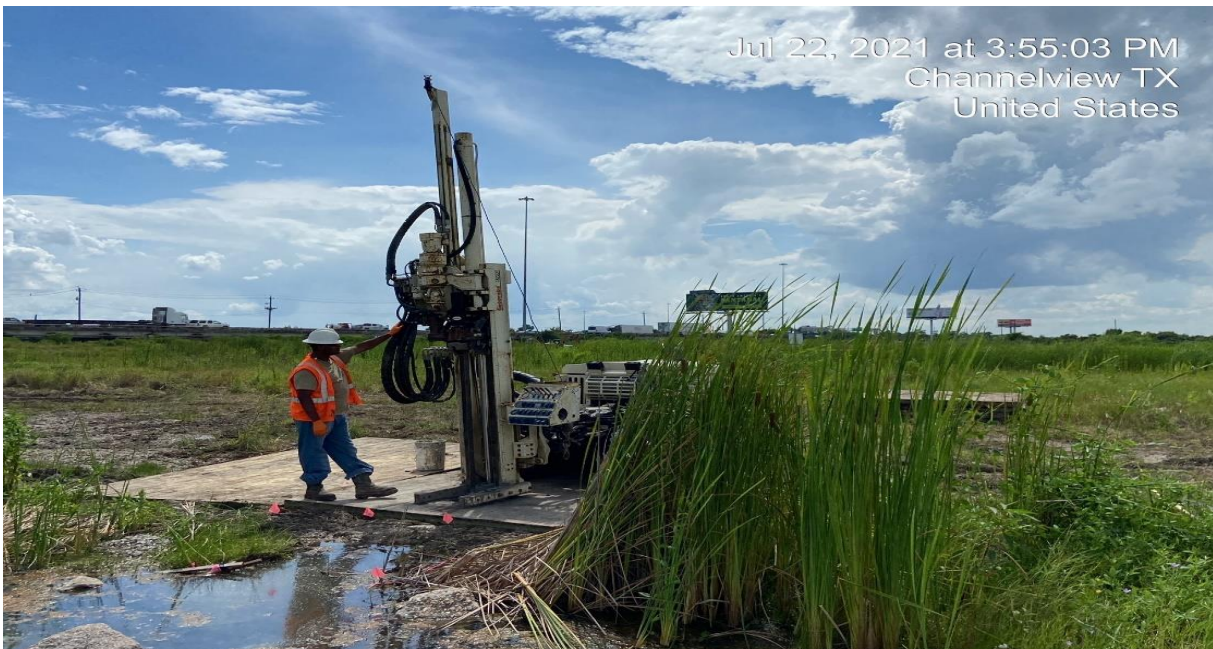
Photo 6 Drill crew positioning drill rig on Northern Impoundment at boring location SJSB076.
