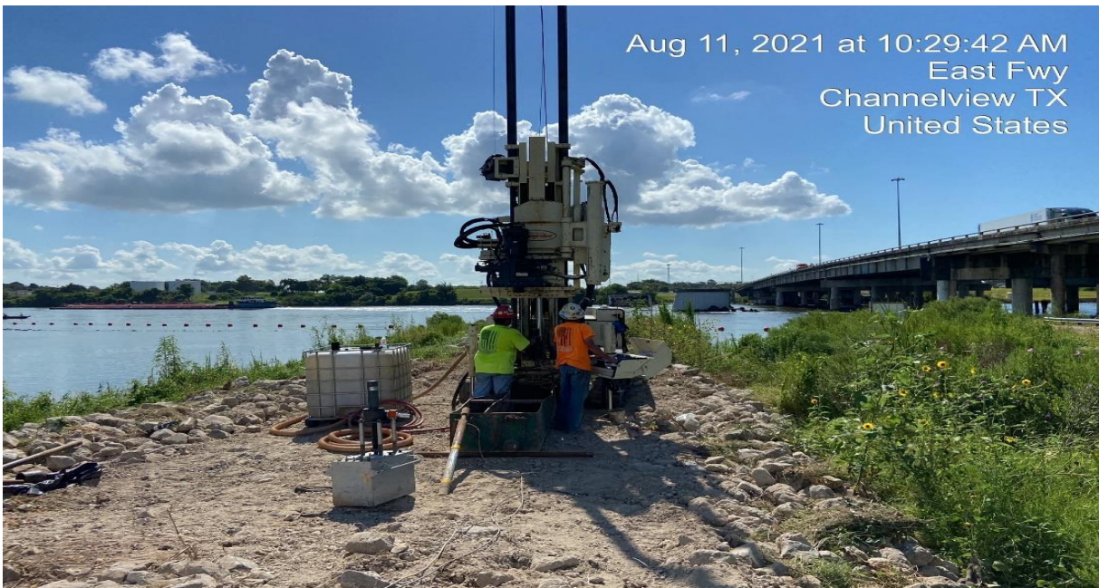
Photo 14 Drill crew installing piezometer SJMW-017.
