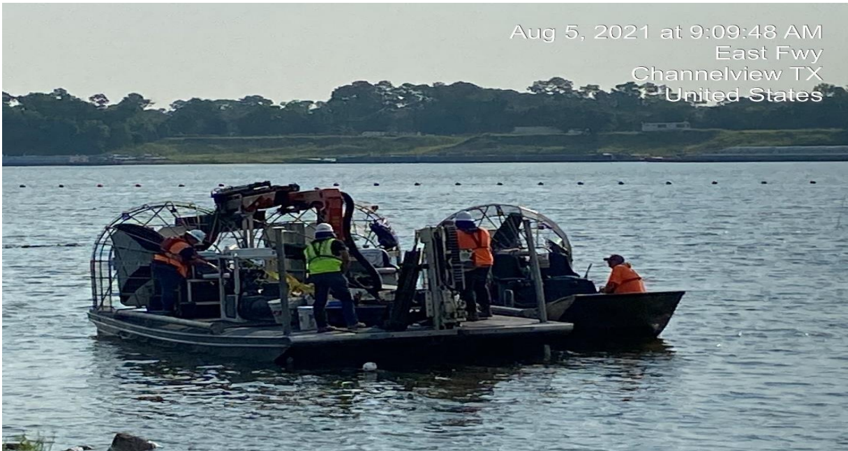
Photo 10 Drill crew collecting soil cores from boring location SJSB081.
