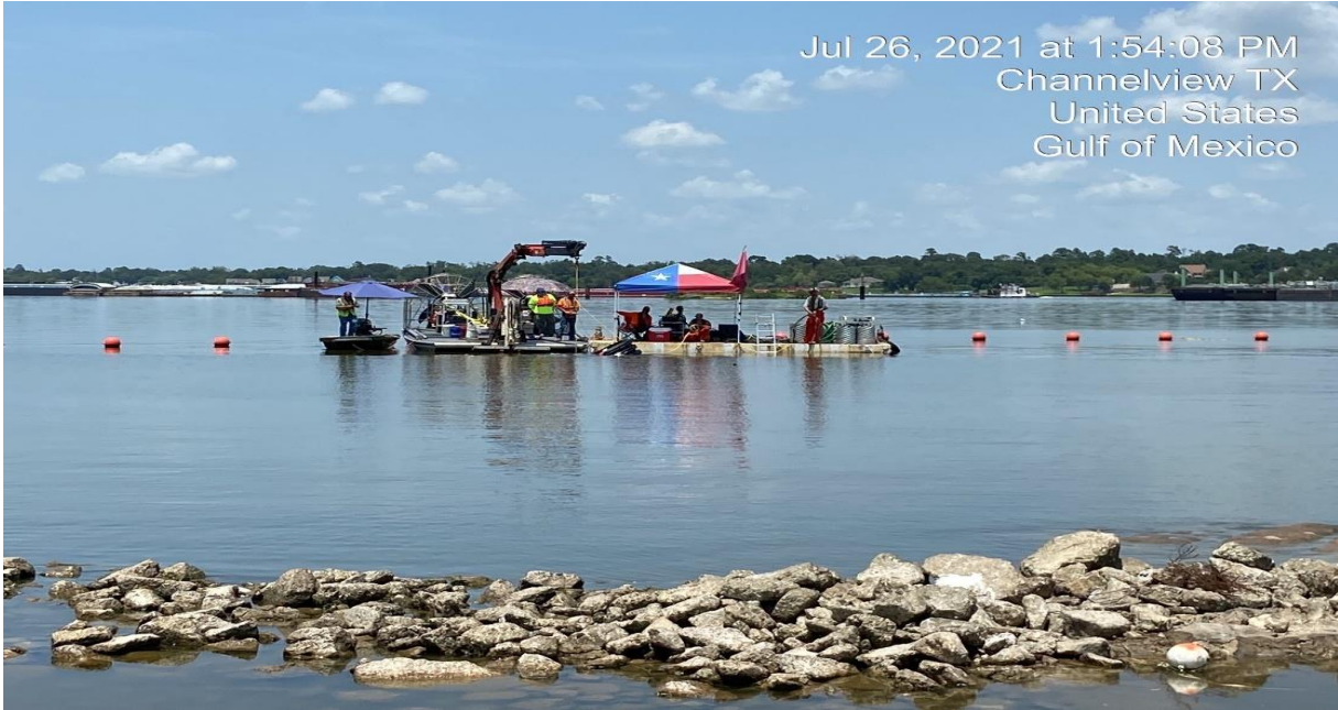
Photo 9 Airboat and dive crews installing a culvert at boring location SJSB097.
