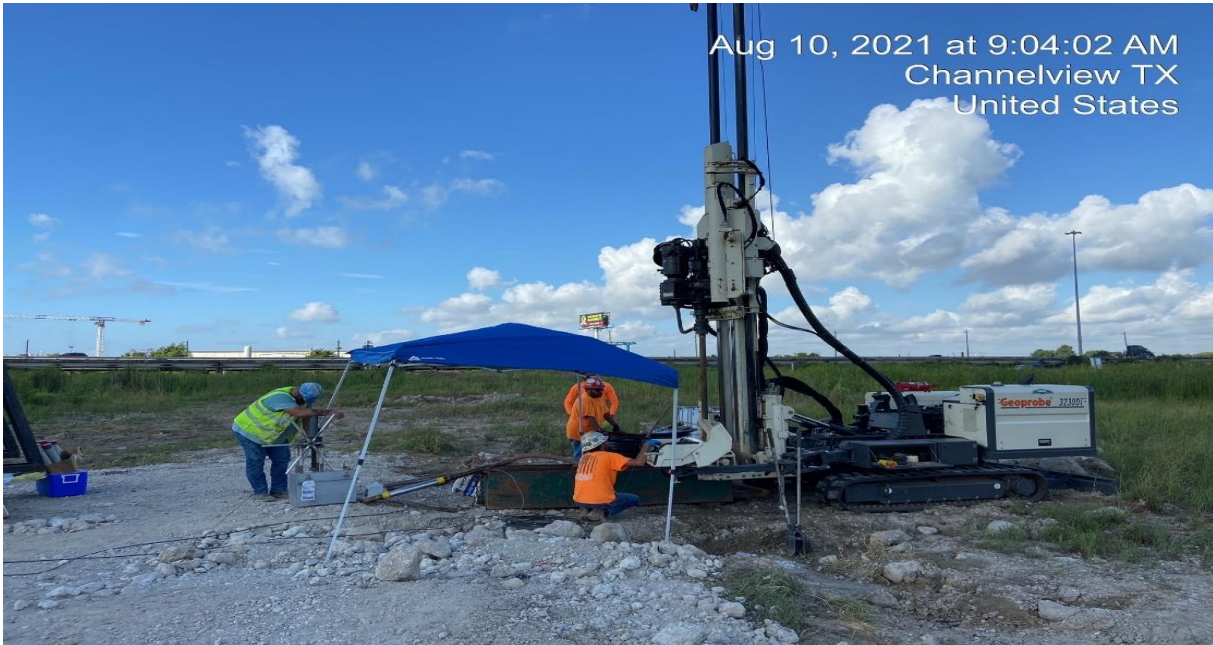
Photo 13 Subcontractor conducting pressure meter tests at piezometer location SJMW-016.
