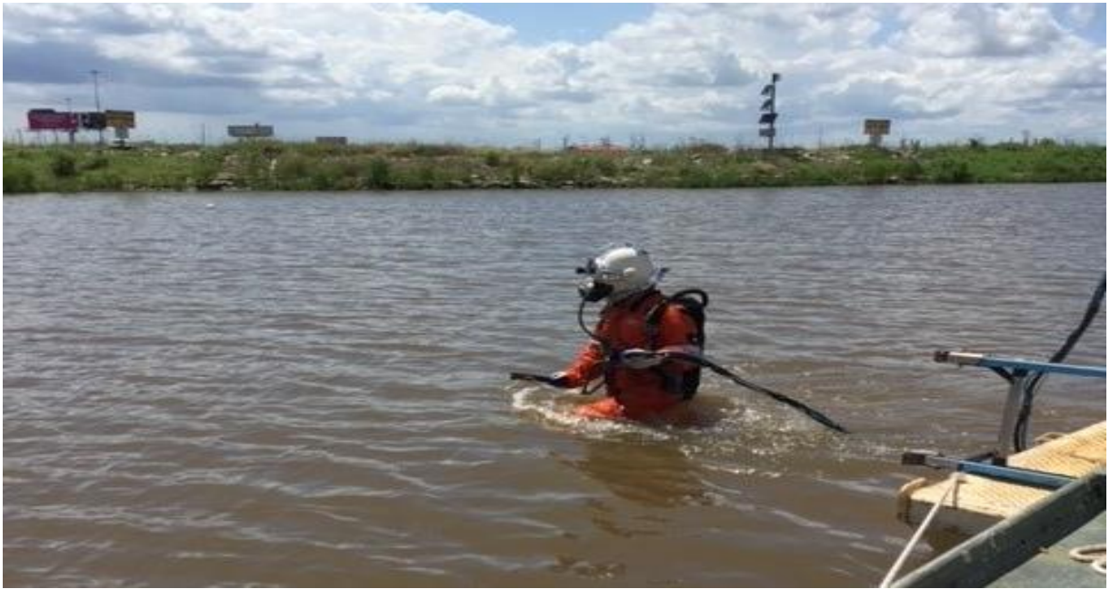
Photo 1 View from airboat. Diver preparing to clear rock cap at boring location SJSB086.
