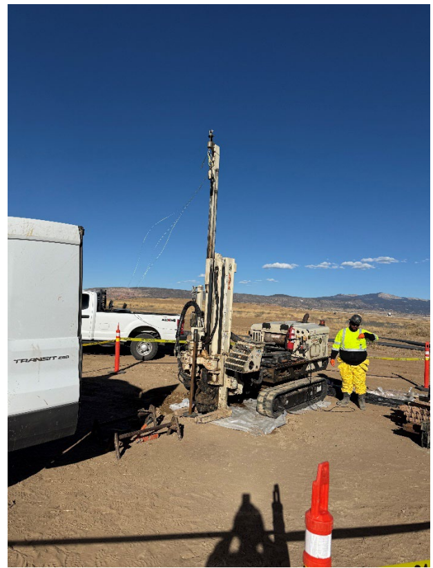
Photo 2: Drill Rig on top of Large Tailings Pile
