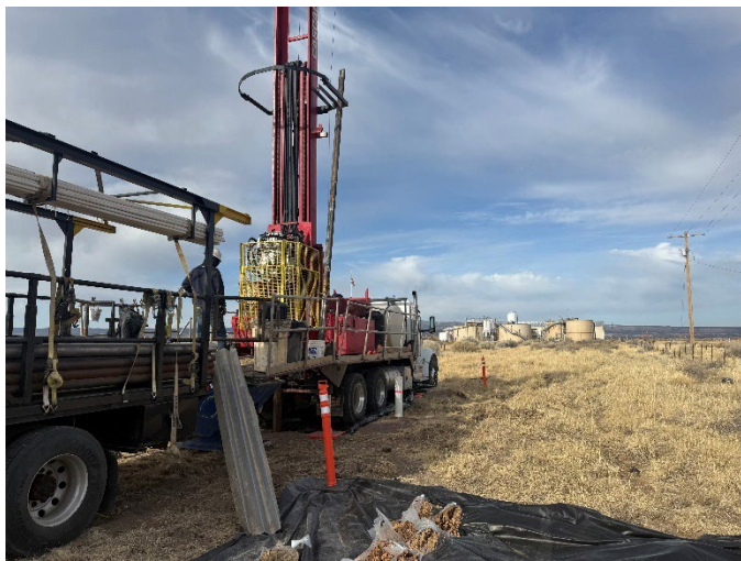
Photo 1: Drilling Rig in Operation at DT1 borehole location
