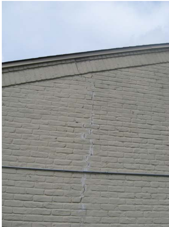
PHOTO 5: This photo shows the crack in the brick veneer on the northern side of the Veterinary Clinic.
