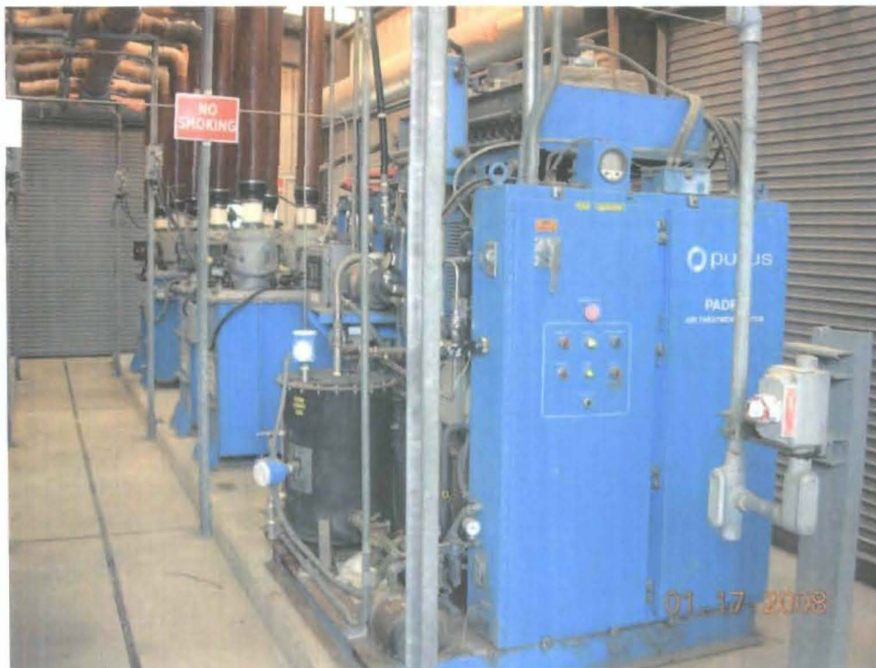
Photo 21. Post-stripper air treatment system. Units in background are solid resin bed adsorption units used to remove volatile contaminants removed by air stripper. Unit in foreground is vapor recovery system used for regeneration of resin beds.
