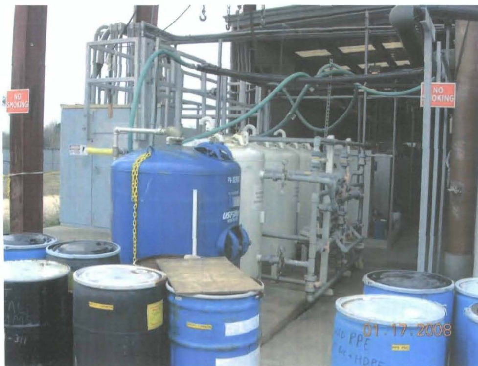
Photo 19. Looking into the treatment area. Blue tank is prefilter using carbon as filter material. Gray tank are carbon filters used to polish water after air stripper.
