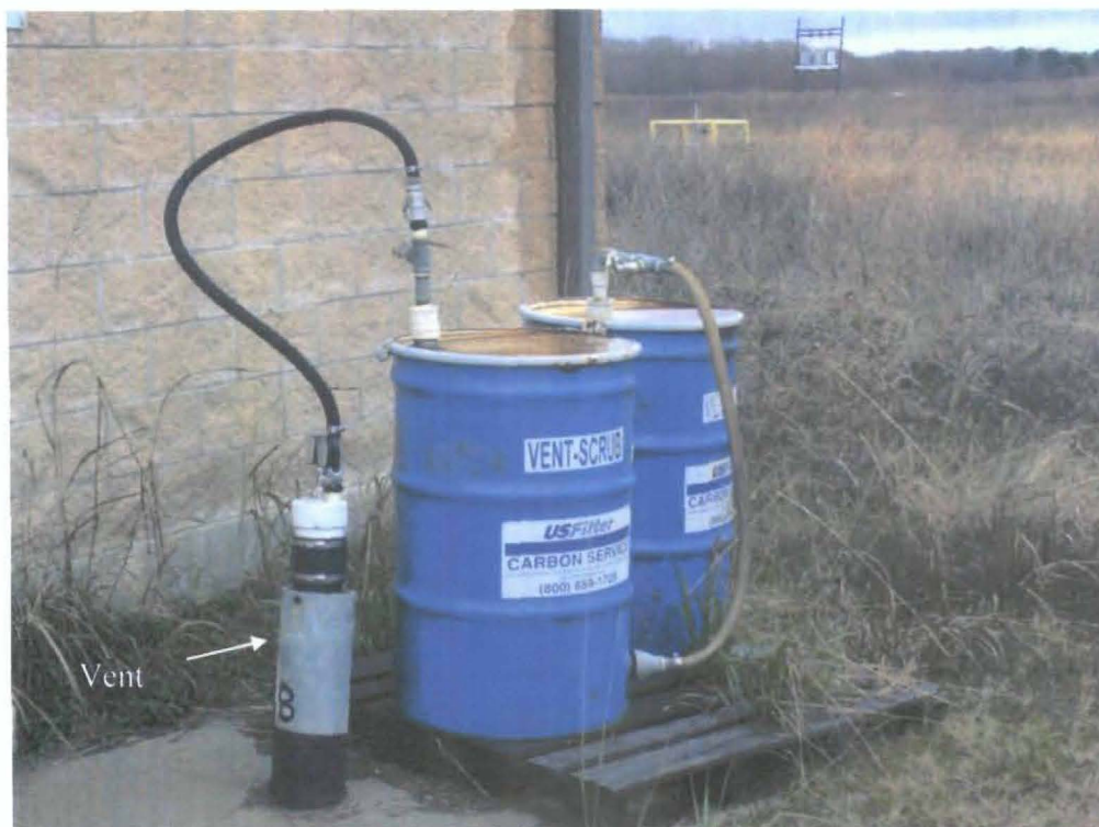
Photo 9. Gas Collection Vent on Compartment "B" located on southwest side of Hub Facility "B". Note the two carbon units used to scrub the vented gas.
