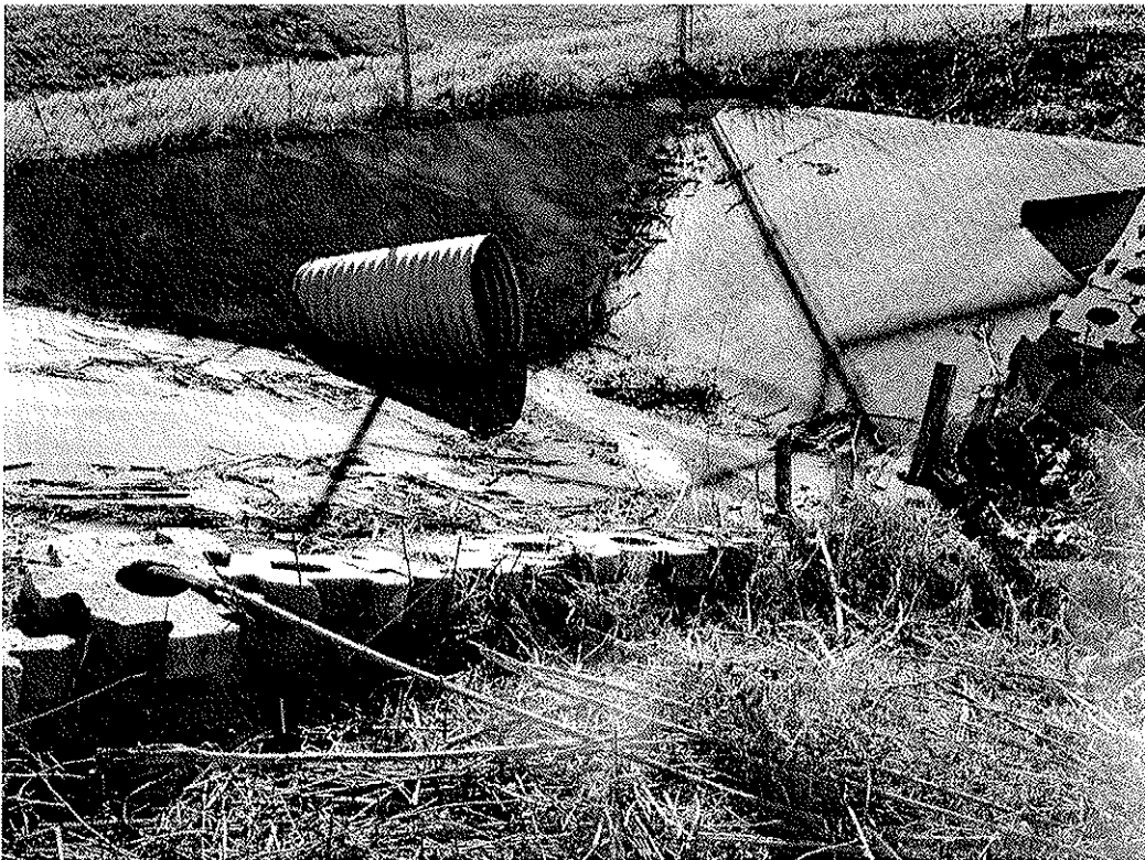
Surface Water Letdown Structure from Perimeter Ditch to Mud Gully
