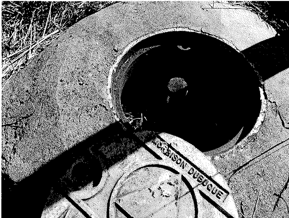
Typical Piezometer Surface Completion and Well Casing
