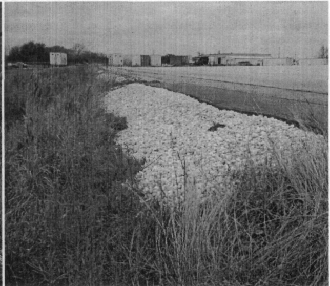
Photo 65. Rip rap and repaired cap along the southern edge of the CC.
