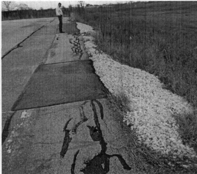
Photo 64. Rip rap and repaired cap along the southern edge of the CC.
