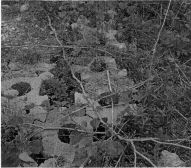
Photo 39. Instability and loss of continuity in the ACB at the toe of the LRB.
