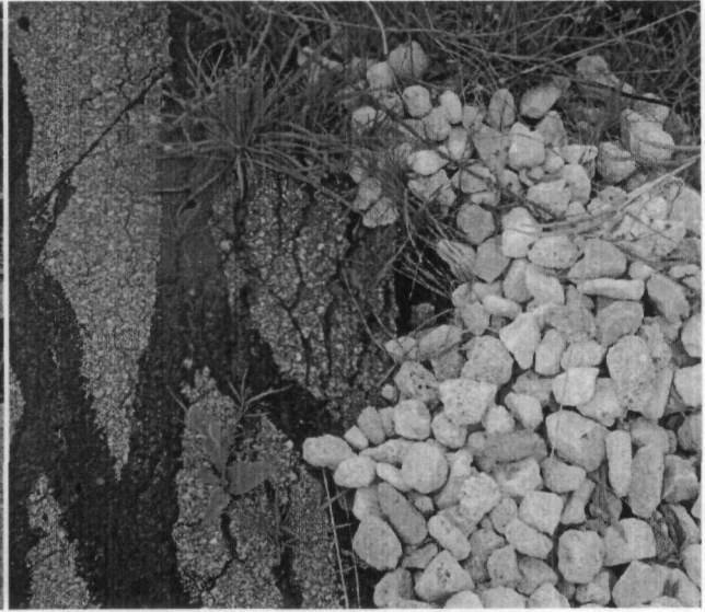
Photo 63. Rip rap along the southern edge of the CC. The hole in the rip rap indicates that erosion may still be occurring.
