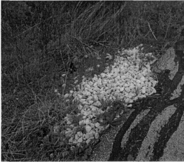
Photo 62. Rip rap along the southern edge of the CC.
