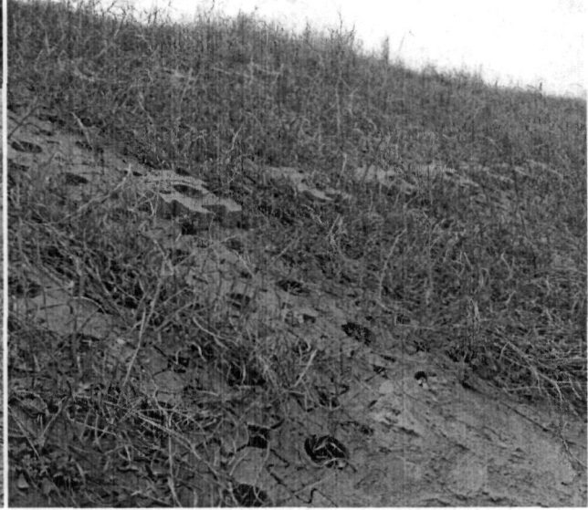
Photo 28. Looking west at ACB from the eastern edge. Note the raised concrete blocks.
