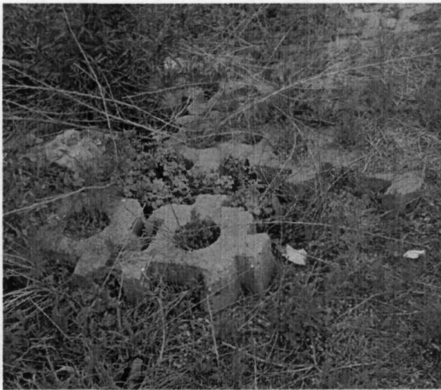
Photo 41. Instability and loss of continuity in the ACB at the toe of the LRB.
