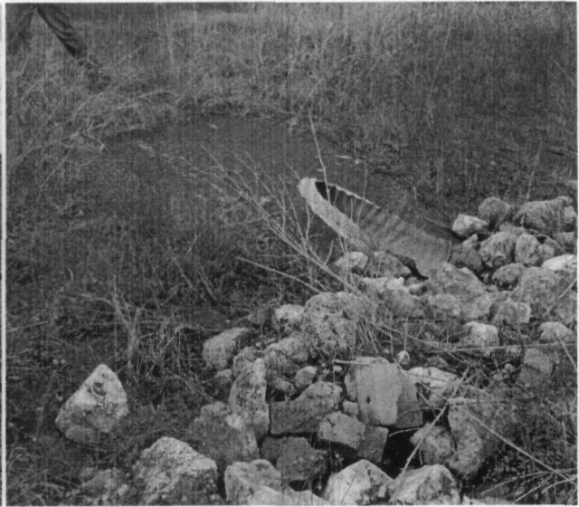
Photo 71. Detention basin outlet pipe.
