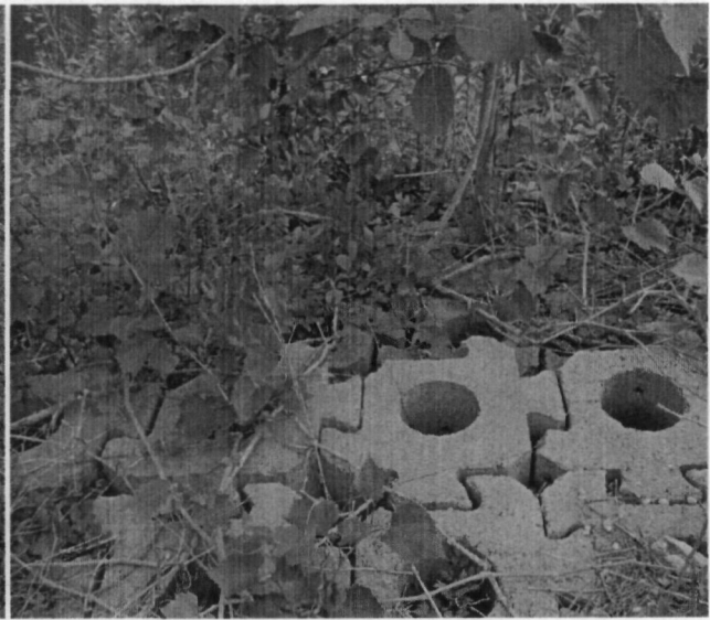
Photo 42. Instability and loss of continuity in the ACB at the toe of the LRB.
