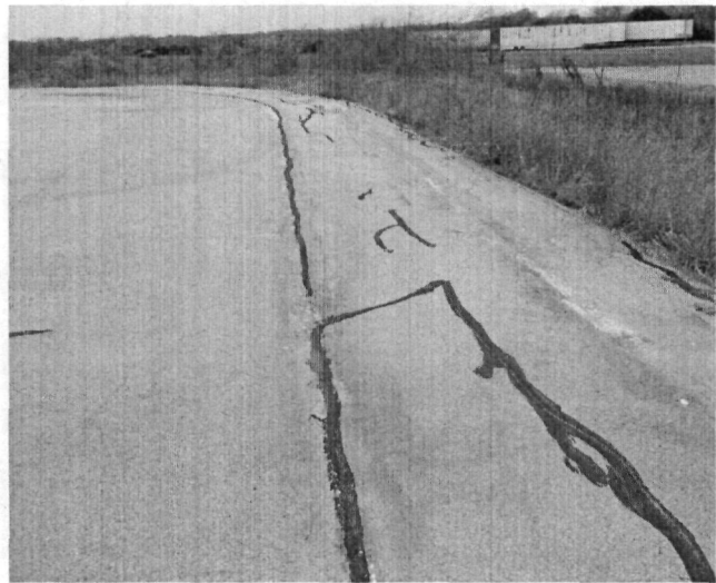
Photo 59. Patched cracks and asphalt repair area.
