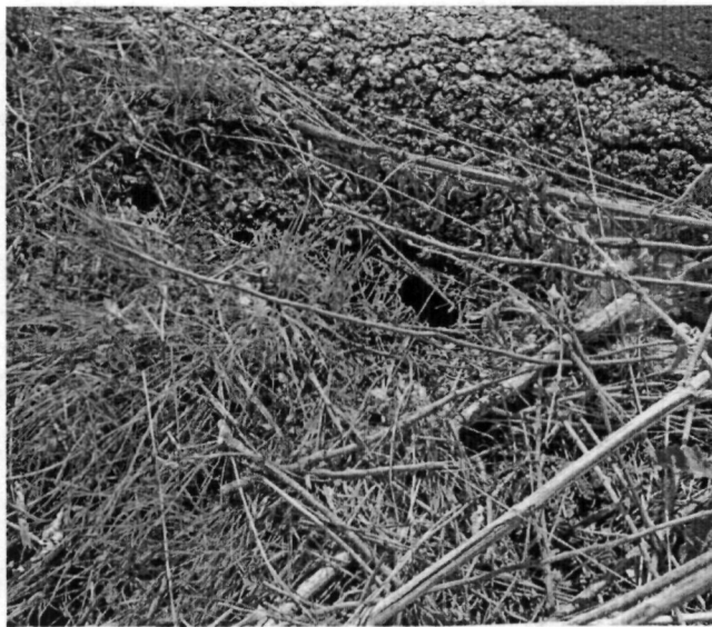
Photo 68. Possible minor erosion at the southern edge of the CC cap.
