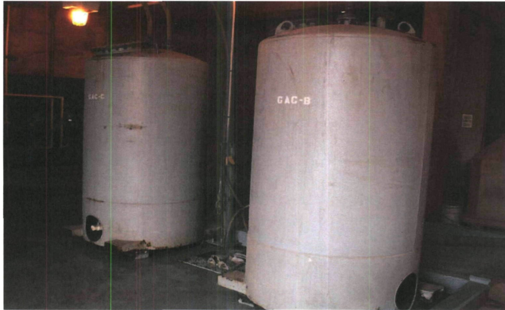
Granulated Activated Carbon Unit at CAPA
