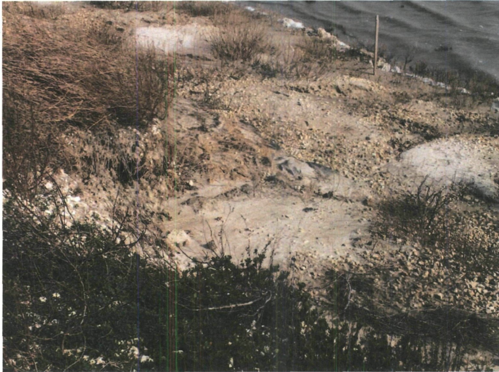
Erosion on Inside Bank of Confined Disposal Facility on Dredge Island
