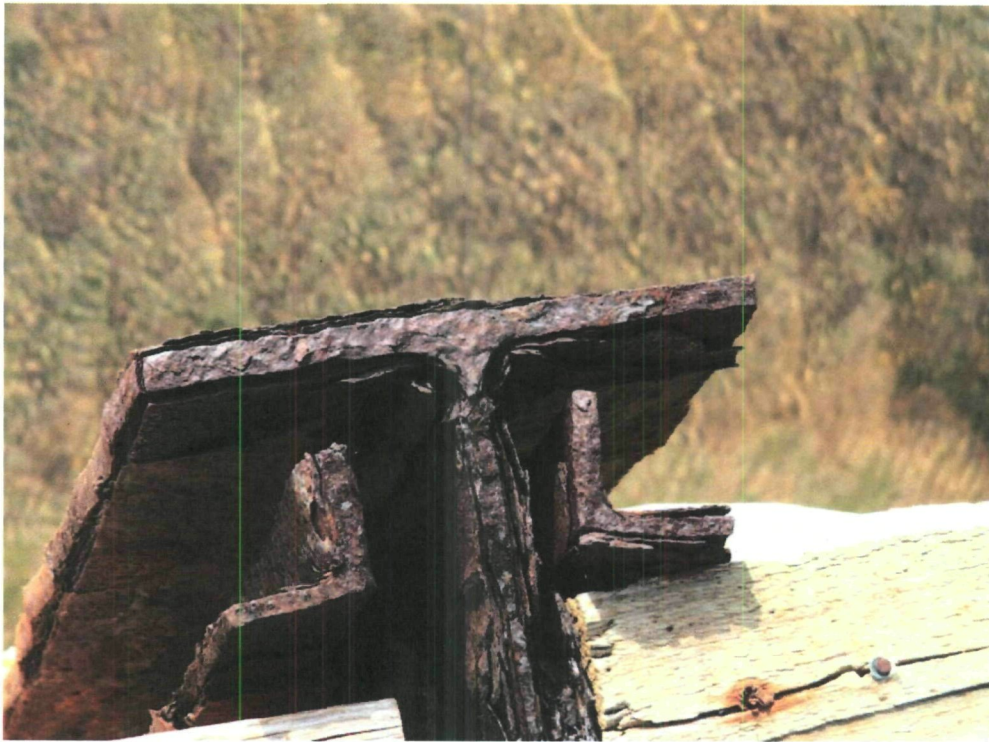
Erosion on Decant Structure on Dredge Island
