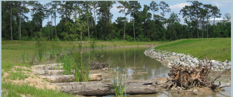
Bioswale with logs repurposed as weirs to provide aquatic habitat and control erosion. Gradual slope on left side of the bioswale allows water to spread out and slow down during periods of high water.
