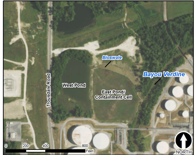
Aerial view of the revitalized west pond connected to Bayou Verdine by the bioswale constructed along the northern edge of the site’s containment cell.
