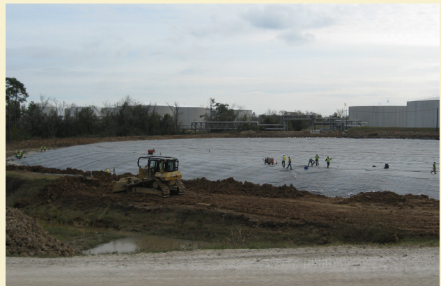
Installation of the containment cell's top liner in December 2014.
