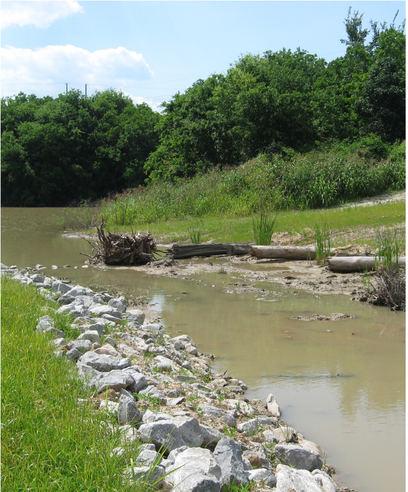
The Bayou Verdine cleanup included various ecological revitalization aspects, including a bioswale (above), which improves the west pond ecosystem by connecting it to Bayou Verdine.
