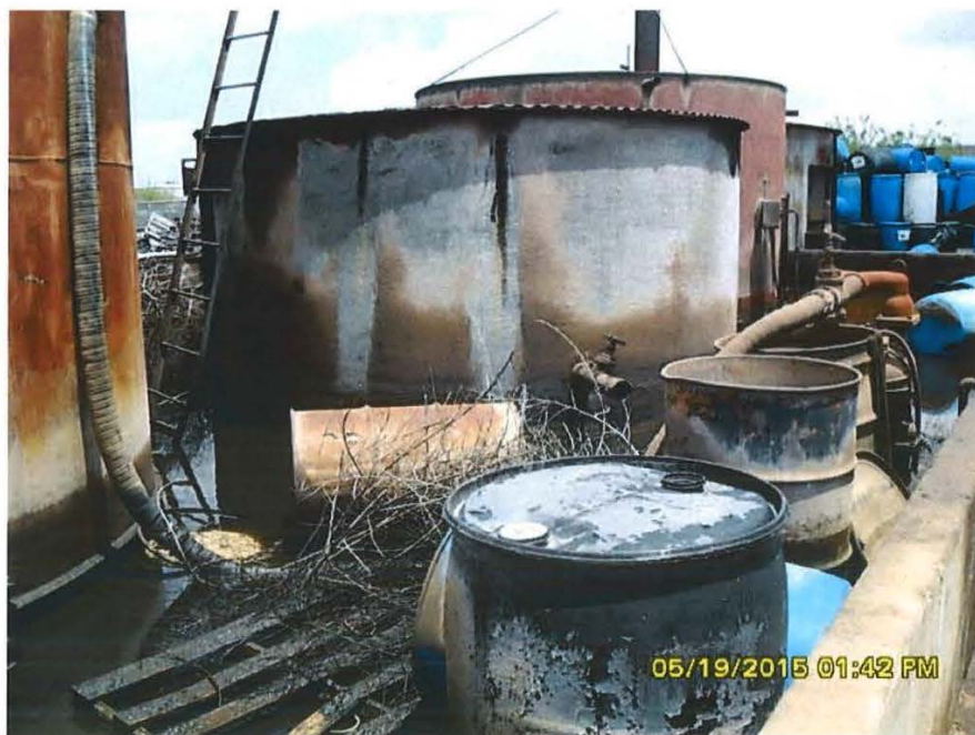
Figure 4 - Secondary containment with three AST's, unknown oily liquid and several opened drums.
