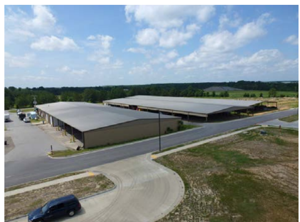
Figure 4: Drive-through recycling center and storage sheds
