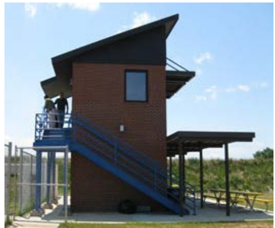
Figure 9: Firing range control room
