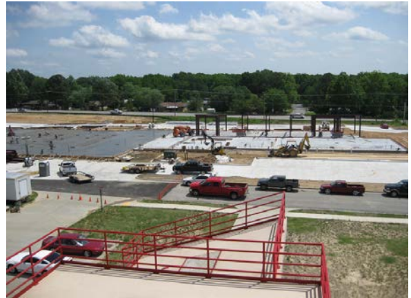
Figure 13: Public safety building under construction
