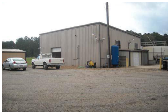
Figure 6. On-site ground water treatment plant facility.
