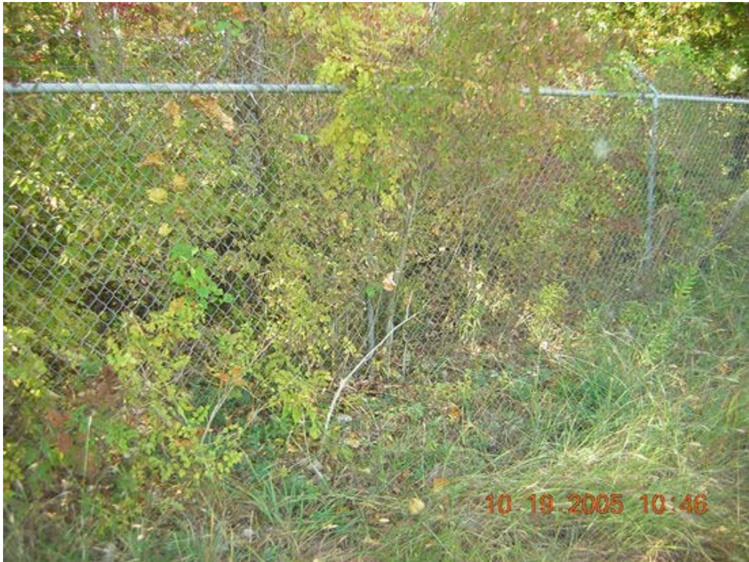
Photo 20: Trees growing through perimeter fence on south side.
