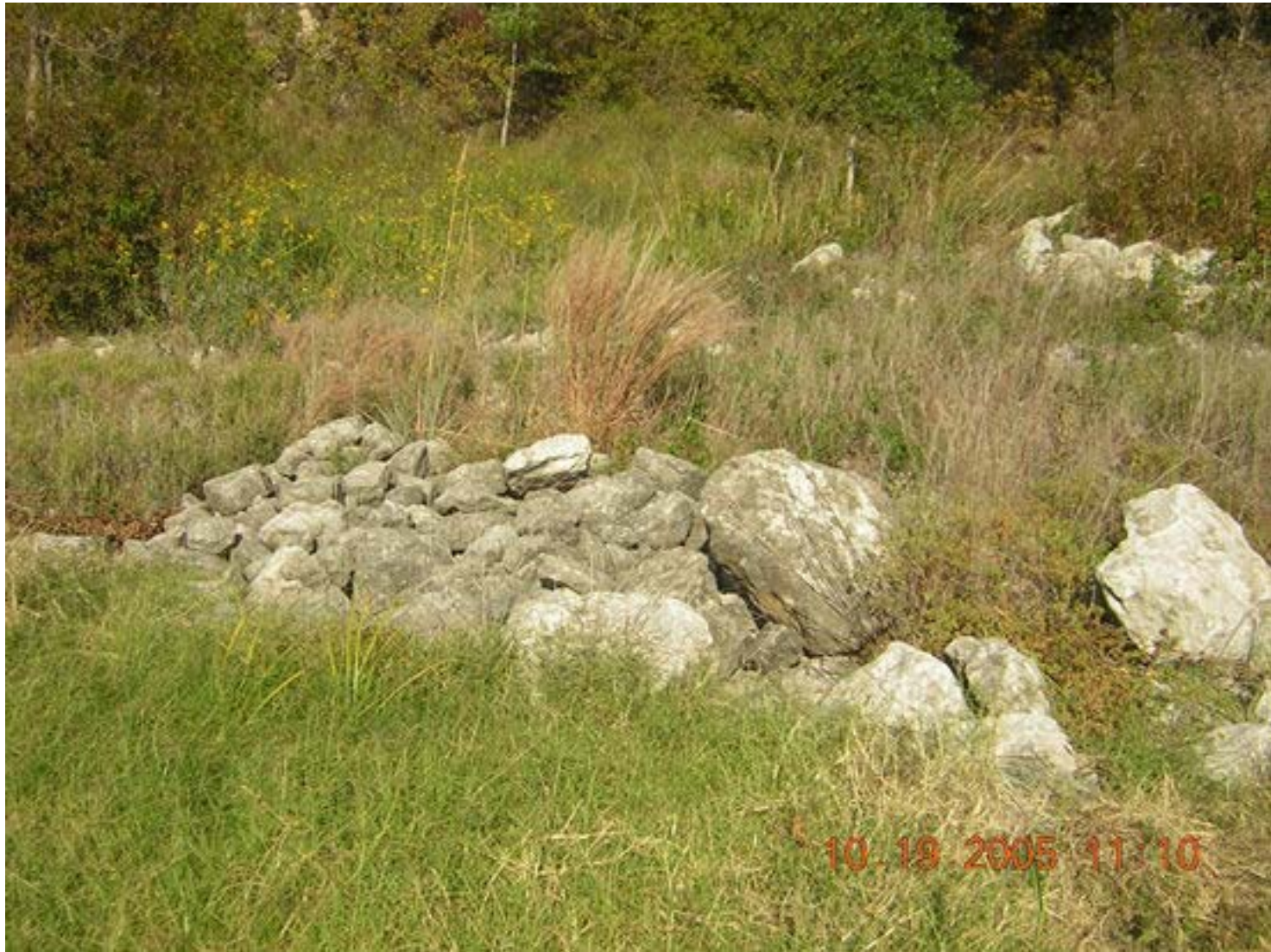
Photo 31: Riprap to prevent erosion along western edge of landfill.
