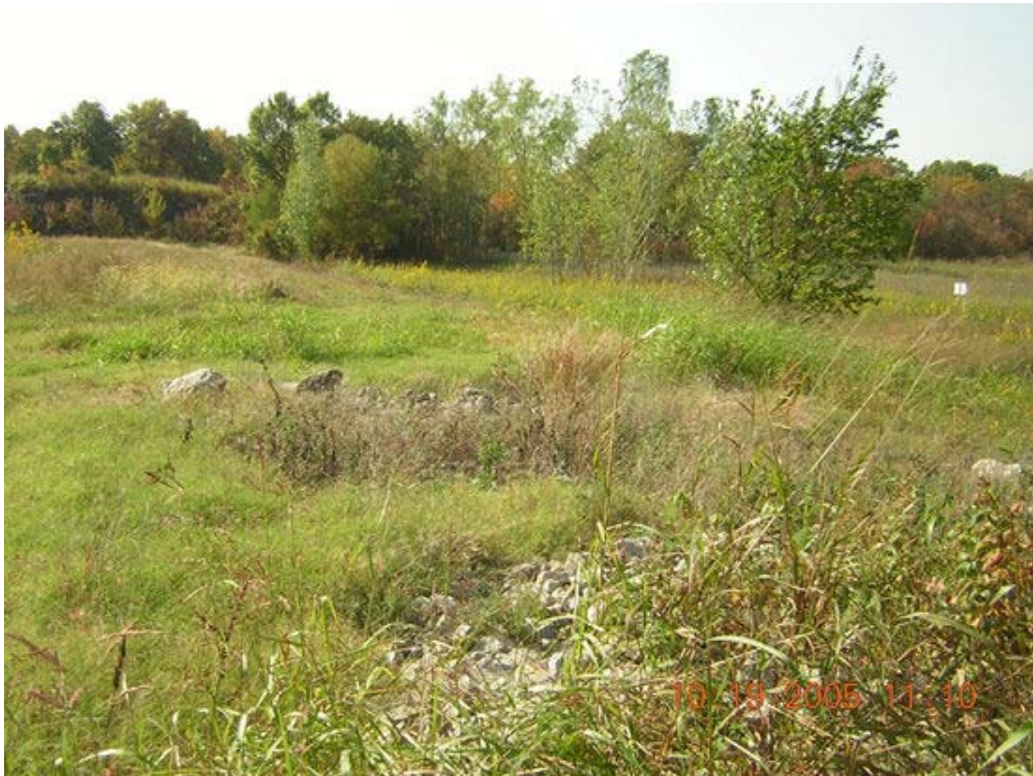
Photo 32: Western edge of landfill. Note riprap to prevent erosion.
