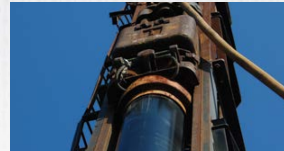
Vulcan 01 Impact Hammer Driving 16" Diameter SUPERPILE®
