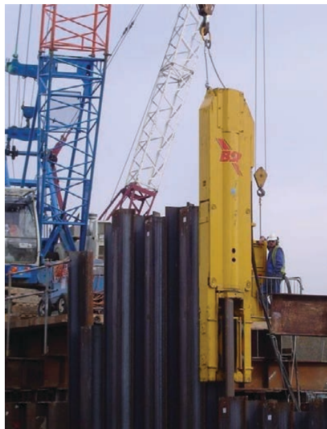
Crane suspended hammer
