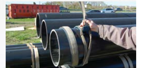
Lift-It® Sling Double Wrapped Around SUPERPILE®
