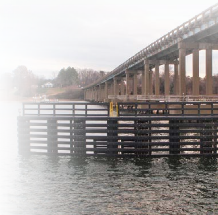
Fender Rehabilitation Route 3 Over Piankatank River, Virginia
