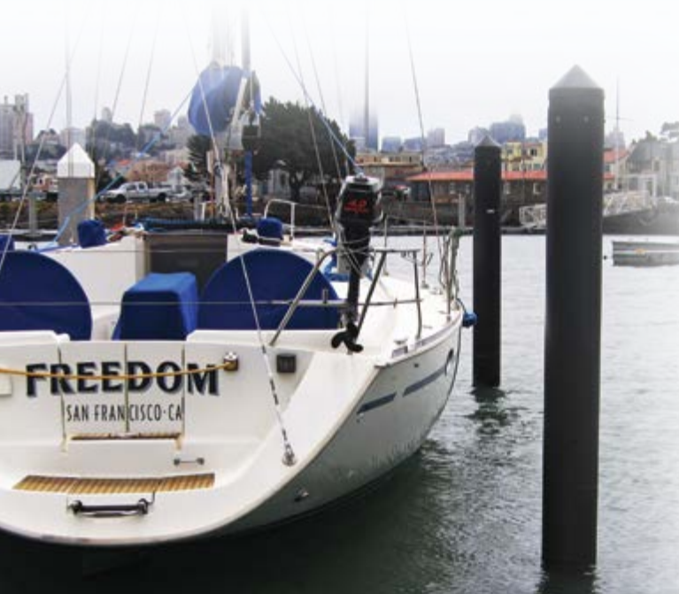
San Francisco West Harbor Renovation Project December 2011 (Phase 1), San Francisco, California
