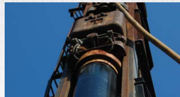
Vulcan 01 Impact Hammer Driving 16" Diameter SUPERPILE®
