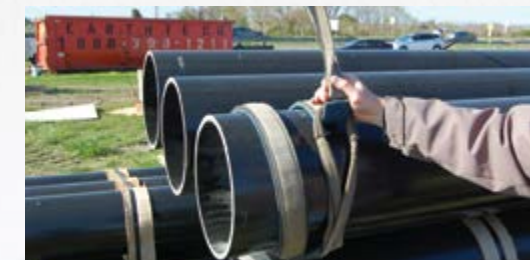
Lift-It® Sling Double Wrapped Around SUPERPILE®
