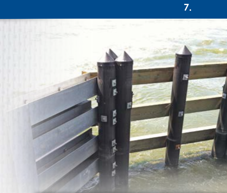
Margate Bridge Installation, Margate New Jersey
