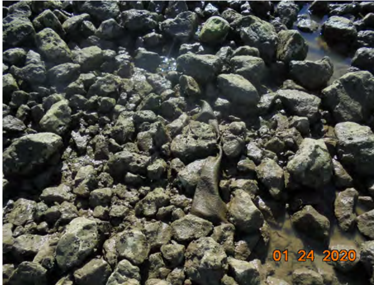
Photograph 5: Example of visible geotextile edge in the eastern cell, prior to maintenance, on January 24, 2020
