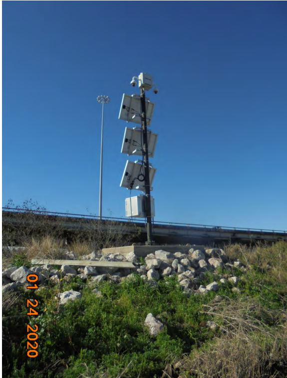
Photograph 21: View of security camera apparatus on southern berm (eastern cell) (view southwest)
