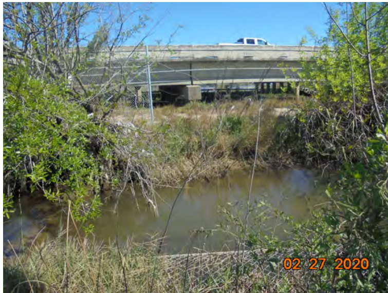
Photograph 11: View of eastern fence termination and ditch south of I-10 on west bank, prior to installation of fence extension, on February 27, 2020 (view northeast)
