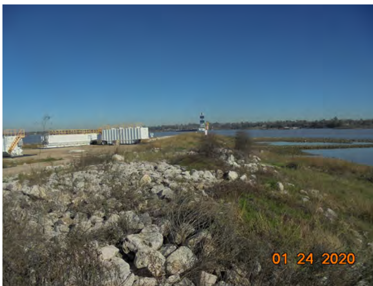
Photograph 3: View from the top of the central berm (view north)
