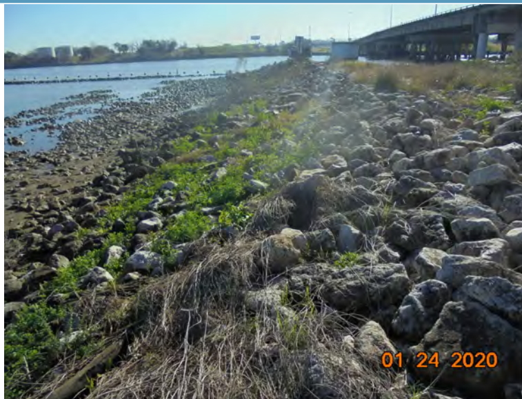
Photograph 1: View along the southern berm (view east)
