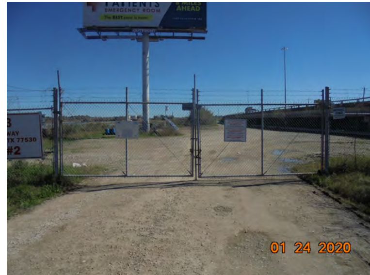
Photograph 8: View of perimeter fence at access gate north of I-10 (view east)
