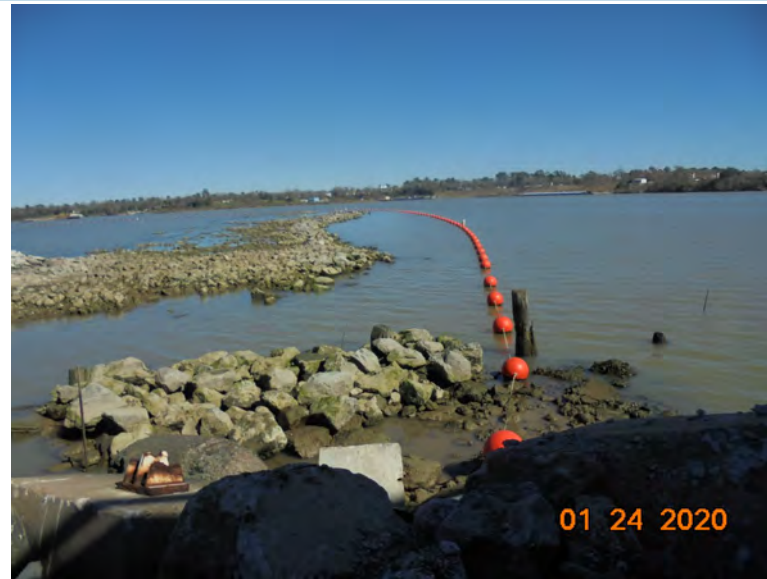
Photograph 18: View of buoys along eastern cell boundary (view northeast)
