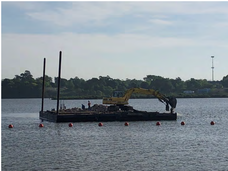
Photograph 2 – Rock being placed at Placement Area 2 with Dynamic Excavator.
