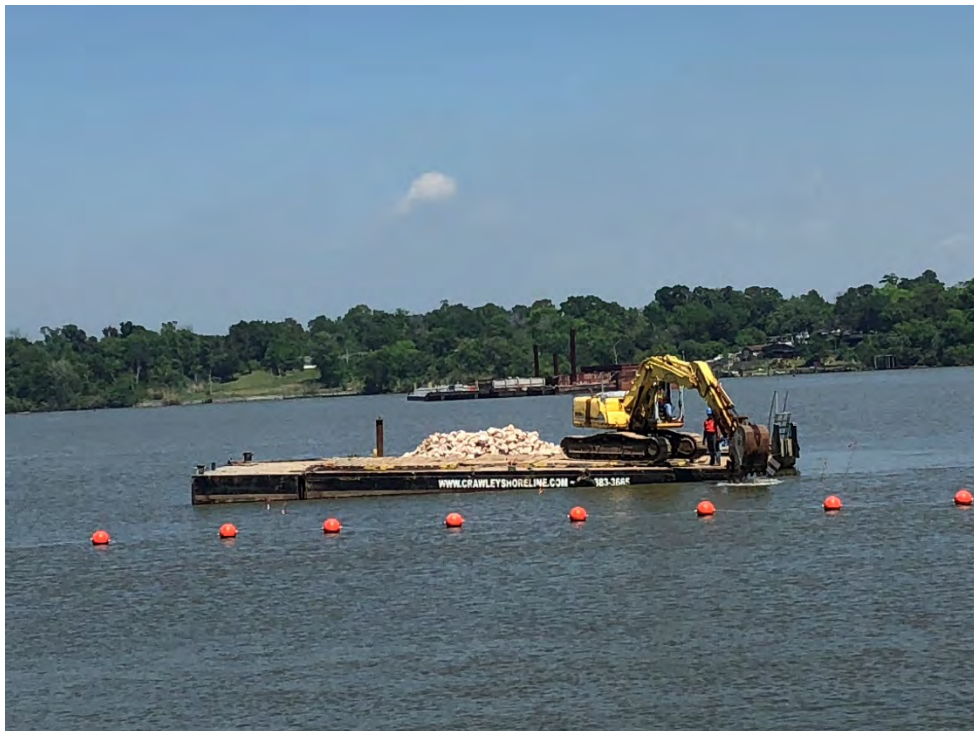
Photograph 4 – Rock being placed at Placement Area 1 with Dynamic Excavator.
