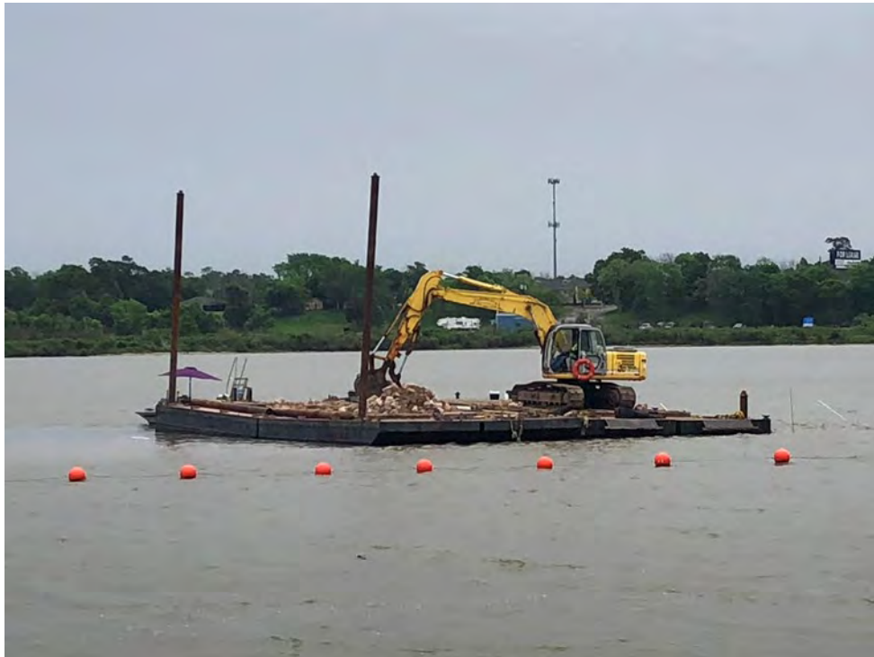
Photograph 1 – Rock being placed at Placement Area 2 with Dynamic Excavator.
