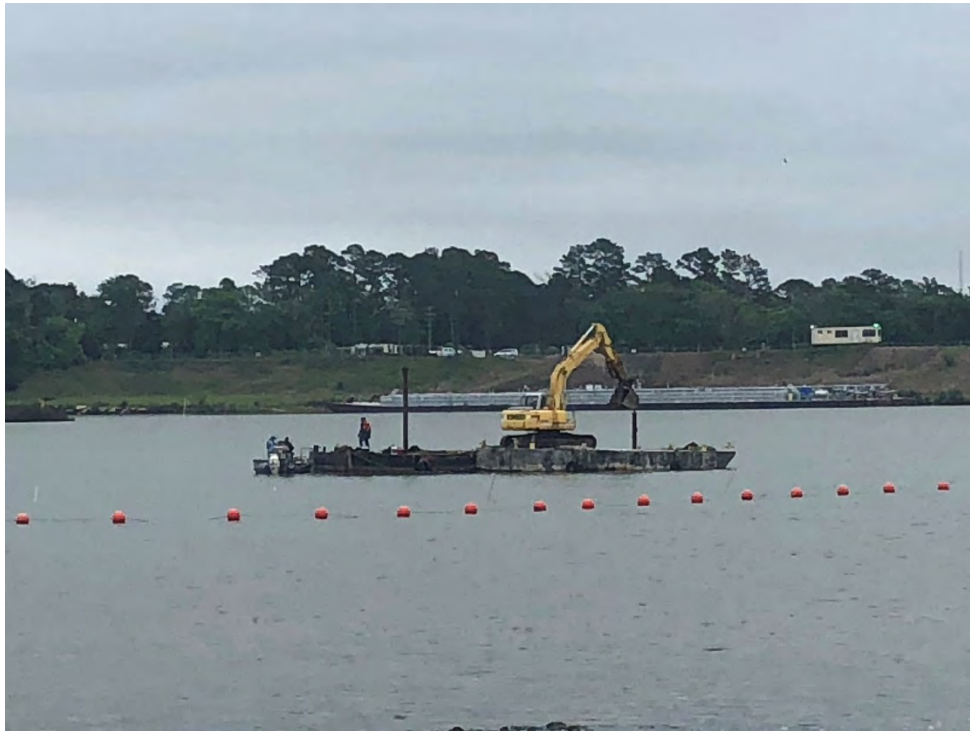
Photograph 1 – Bathymetric survey and rock placement corrections being conducted at Placement Areas 2 and 3.
