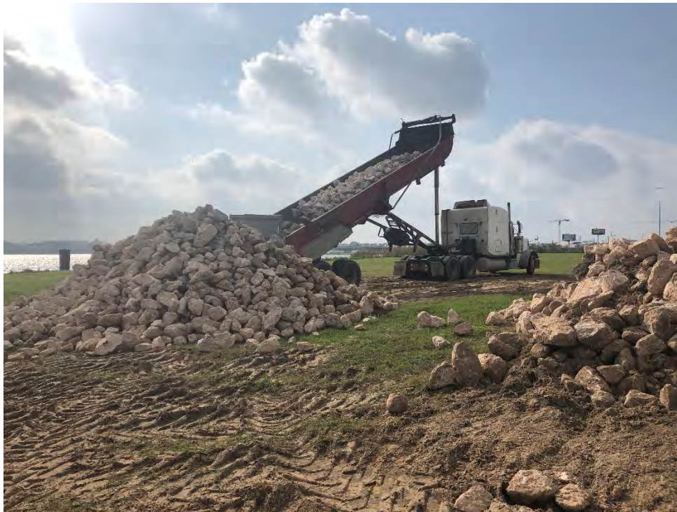
Photograph 1 – Rock delivered to stockpile at San Jacinto River Fleet property.
