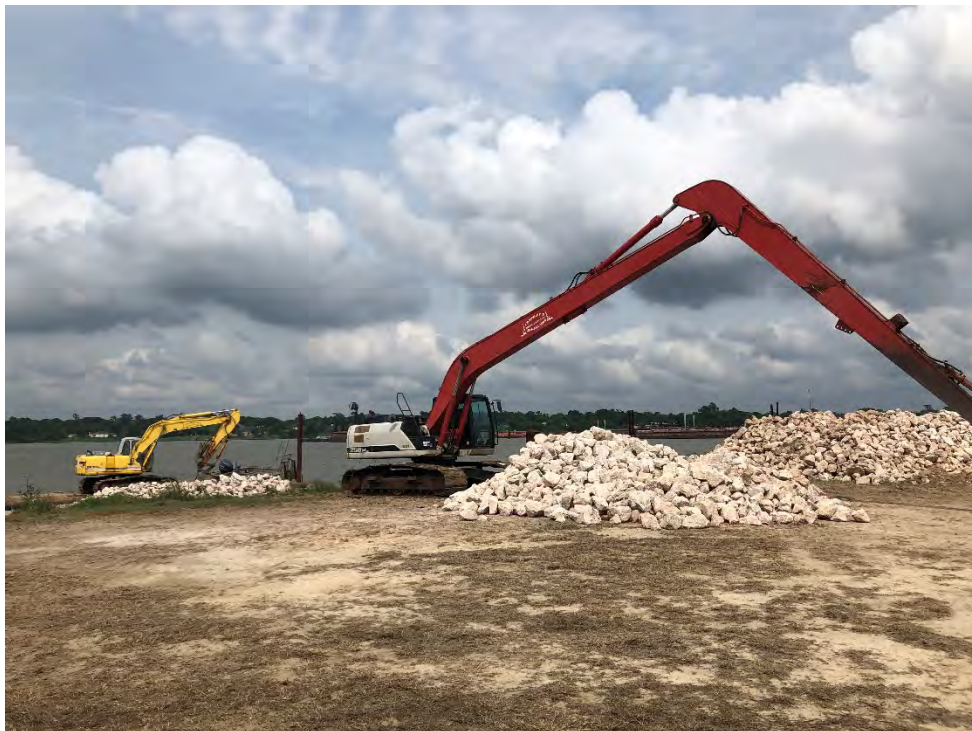
Photograph 4 – Equipment and stockpiled rock at San Jacinto River Fleet property.
