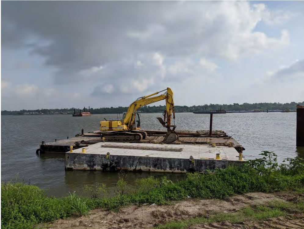
Photograph 2 – Crawley barges and excavator at San Jacinto River Fleet property.
