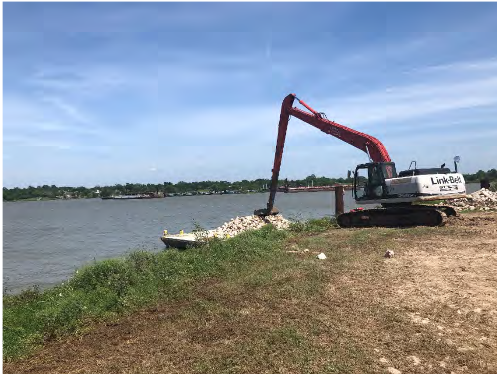
Photograph 1 – Barge loaded with rock at San Jacinto River Fleet property.
