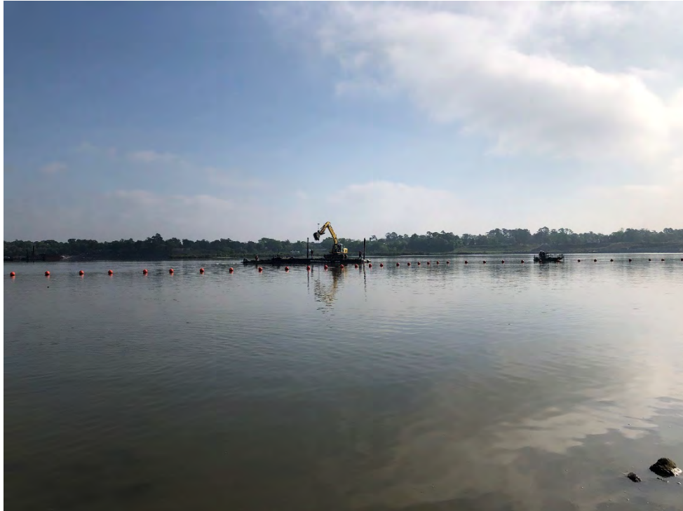
Photograph 3 – Staking and bathymetric survey being conducted at Placement Areas.
