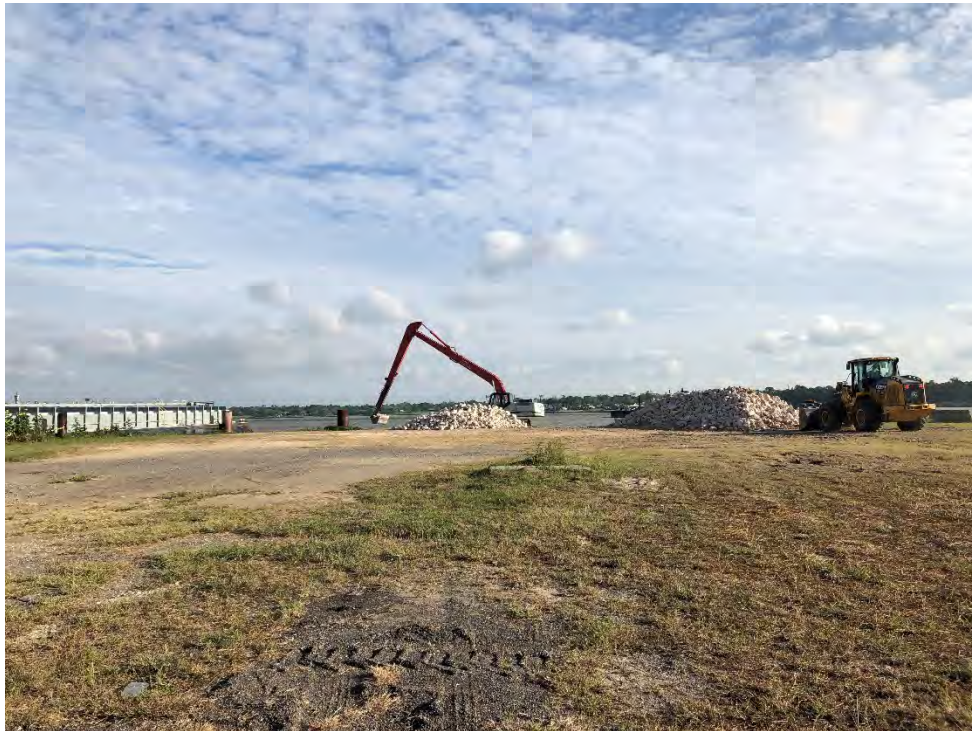
Photograph 1 – Rock being loaded onto barges at San Jacinto River Fleet property.
