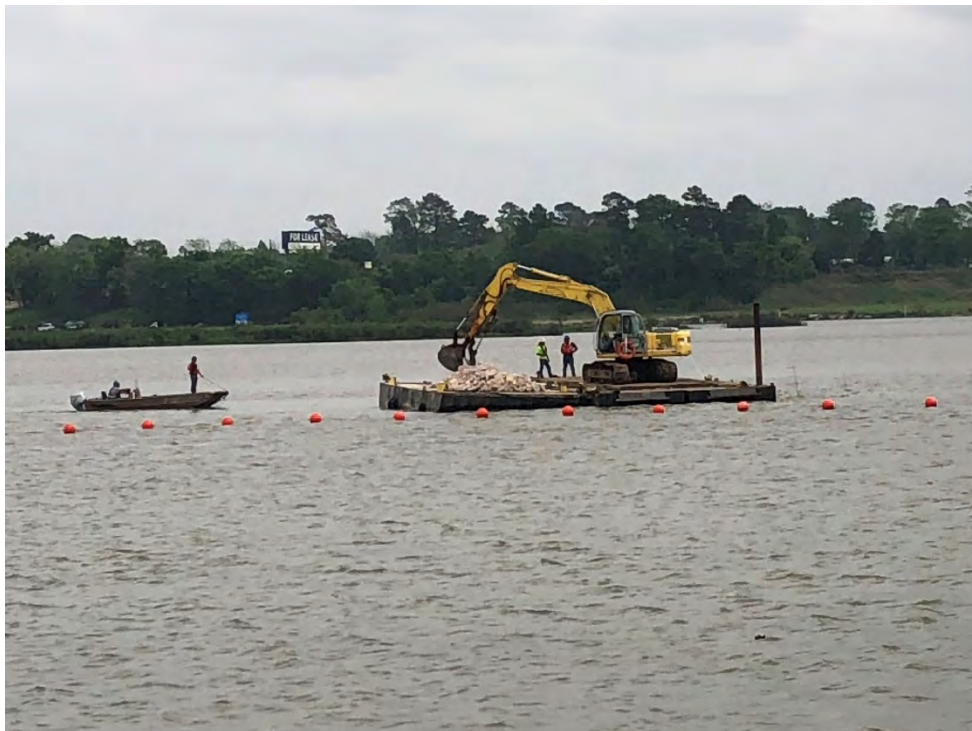
Photograph 2 – Rock being placed at Placement Area 3 with Dynamic Excavator.
