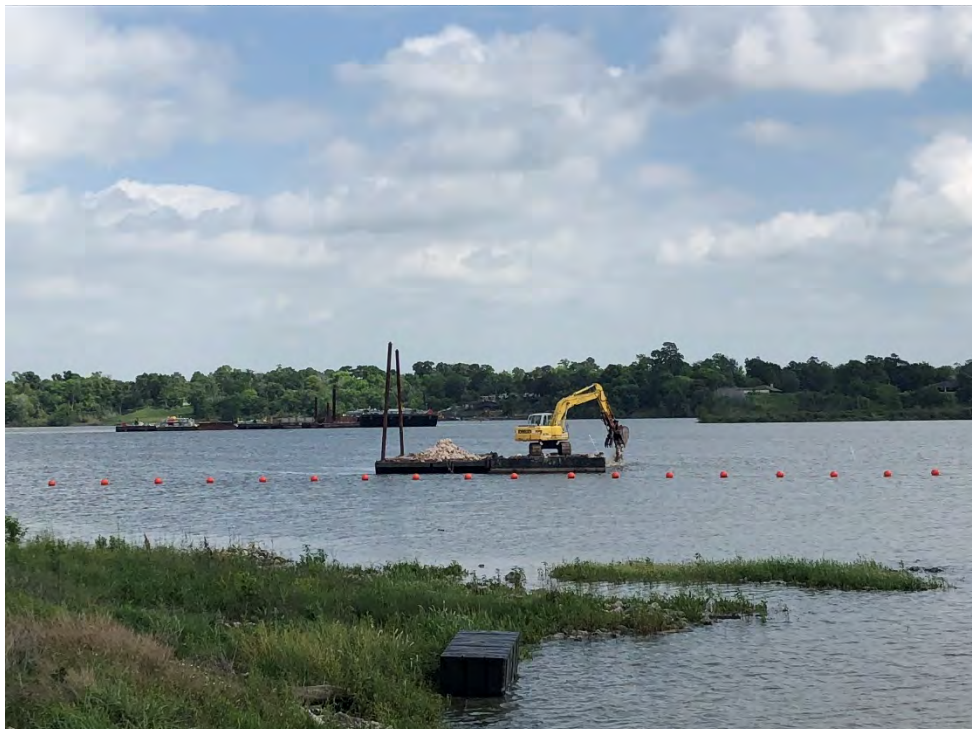
Photograph 4 – Rock being placed at Placement Area 2 with Dynamic Excavator.
