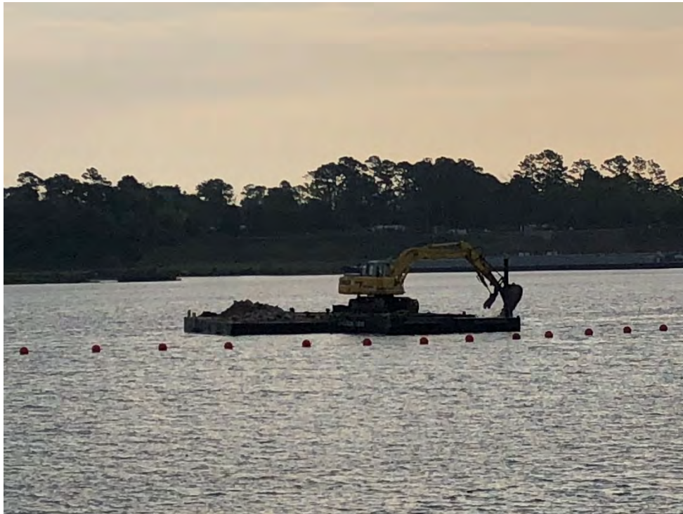
Photograph 1 – Rock being placed at Placement Area 3 with Dynamic Excavator.
