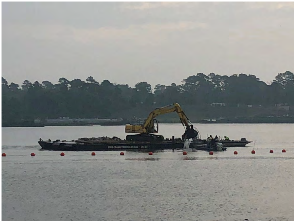
Photograph 2 – Rock placement corrections being conducted at Placement Areas with assistance from surveyors.
