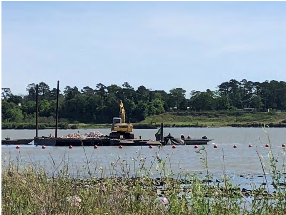
Photograph 3 – Geotextile fabric being placed at Placement Area 3.
