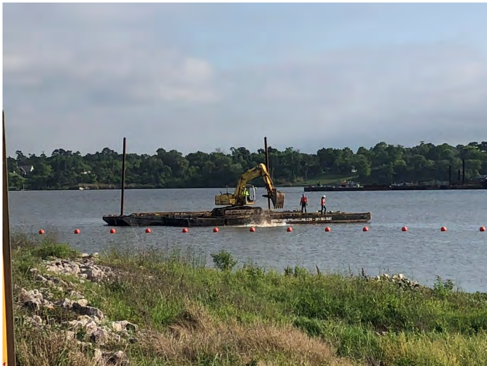
Photograph 2 – Remaining 10 tons of rock being placed at Placement Area 1.
