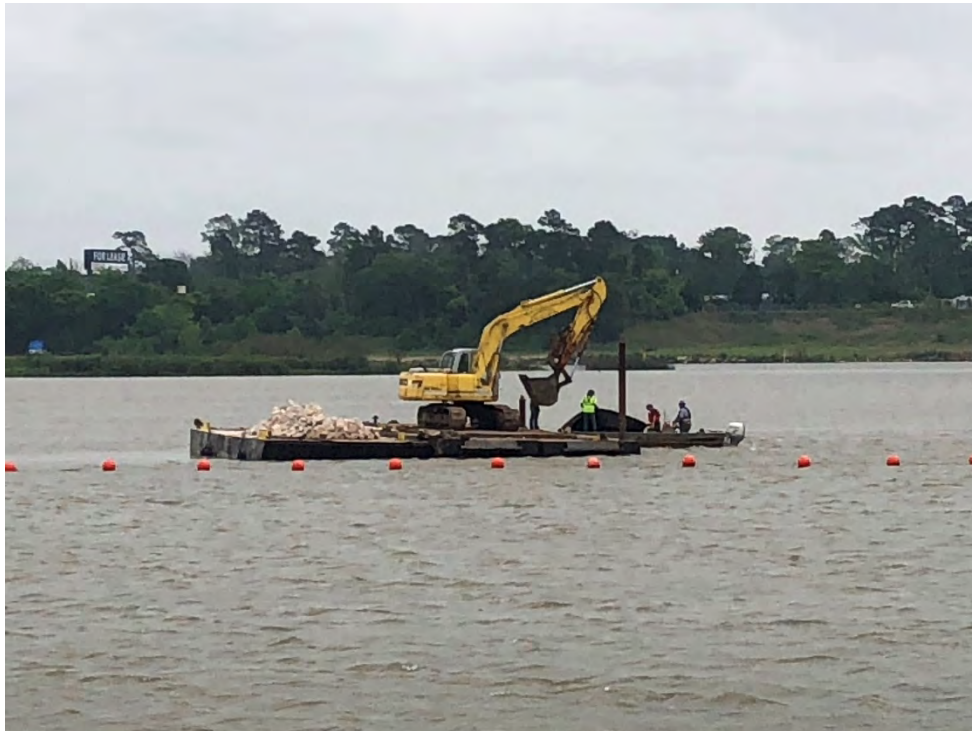
Photograph 3 – Placement of geotextile fabric being conducted at Placement Area 3.
