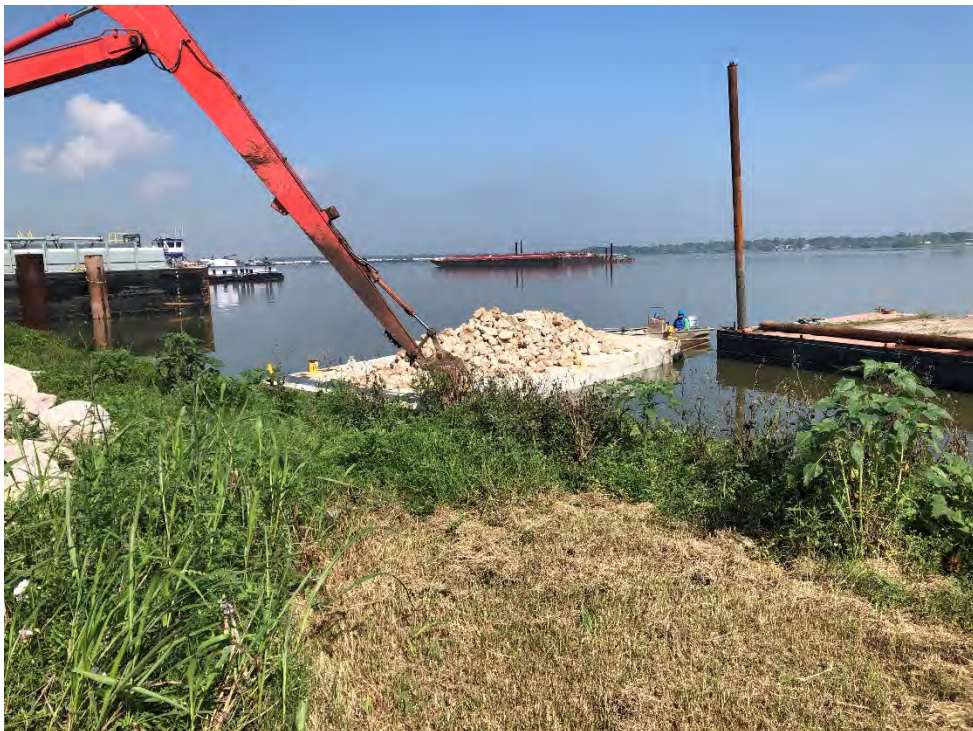
Photograph 2 – Barge loaded with rock at San Jacinto River Fleet property.
