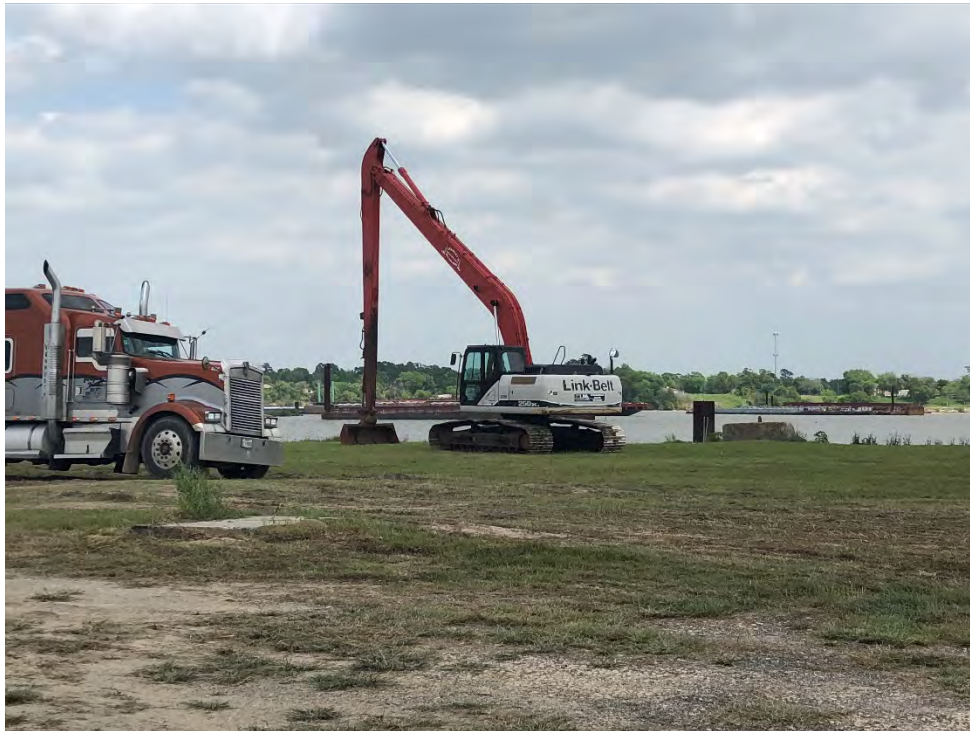
Photograph 2 – Crawley long-reach excavator at San Jacinto River Fleet property.
