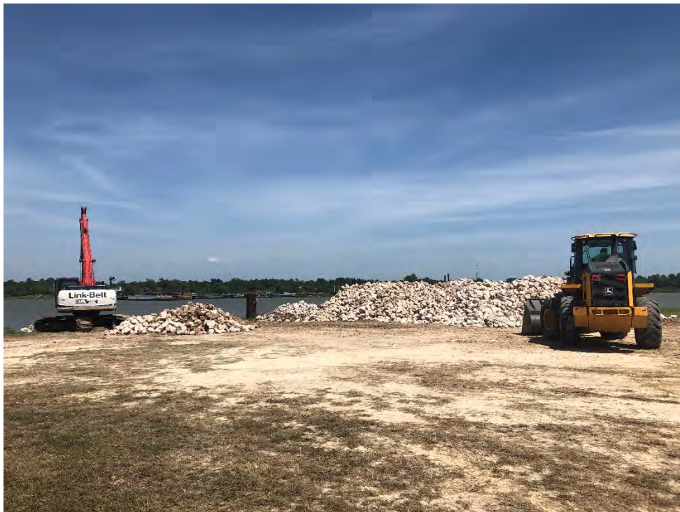
Photograph 4 – Stockpiled rock at San Jacinto River Fleet property.
