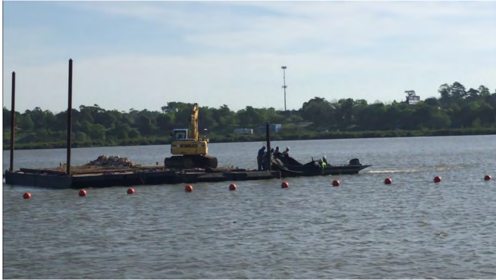
Photograph 3 – Placement of geotextile fabric being conducted at Placement Area 2.
