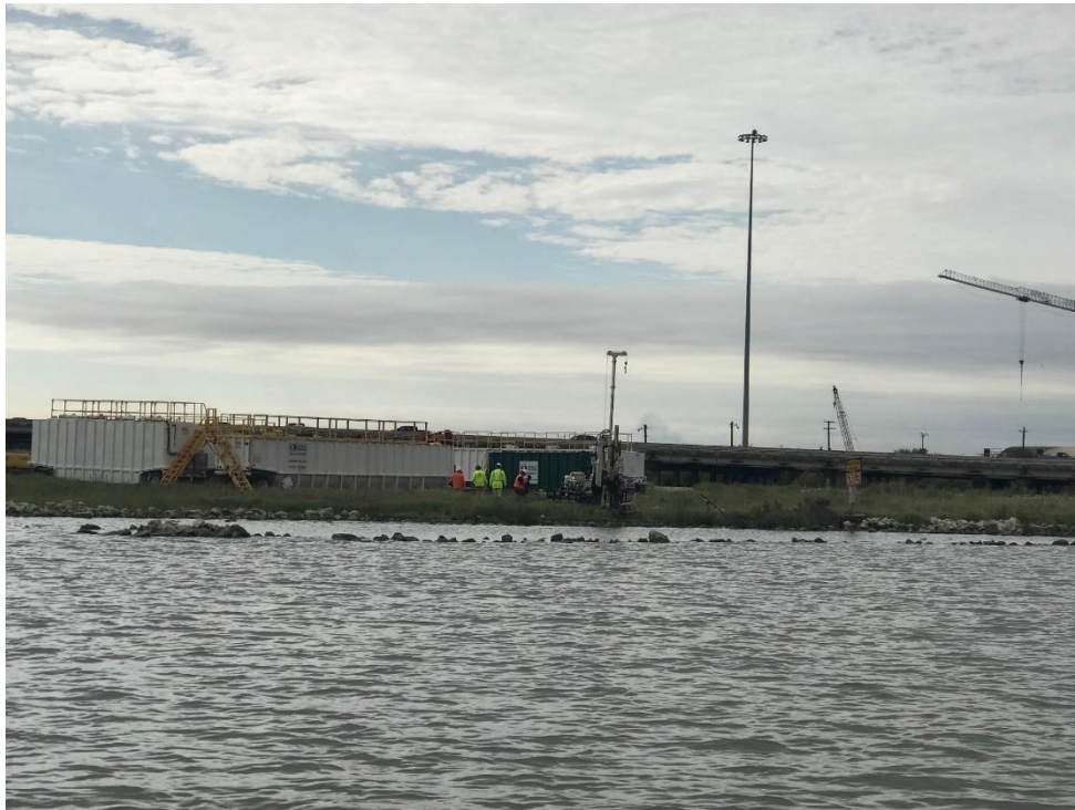
Photo 2 - View of North Impoundment from San Jacinto River.
