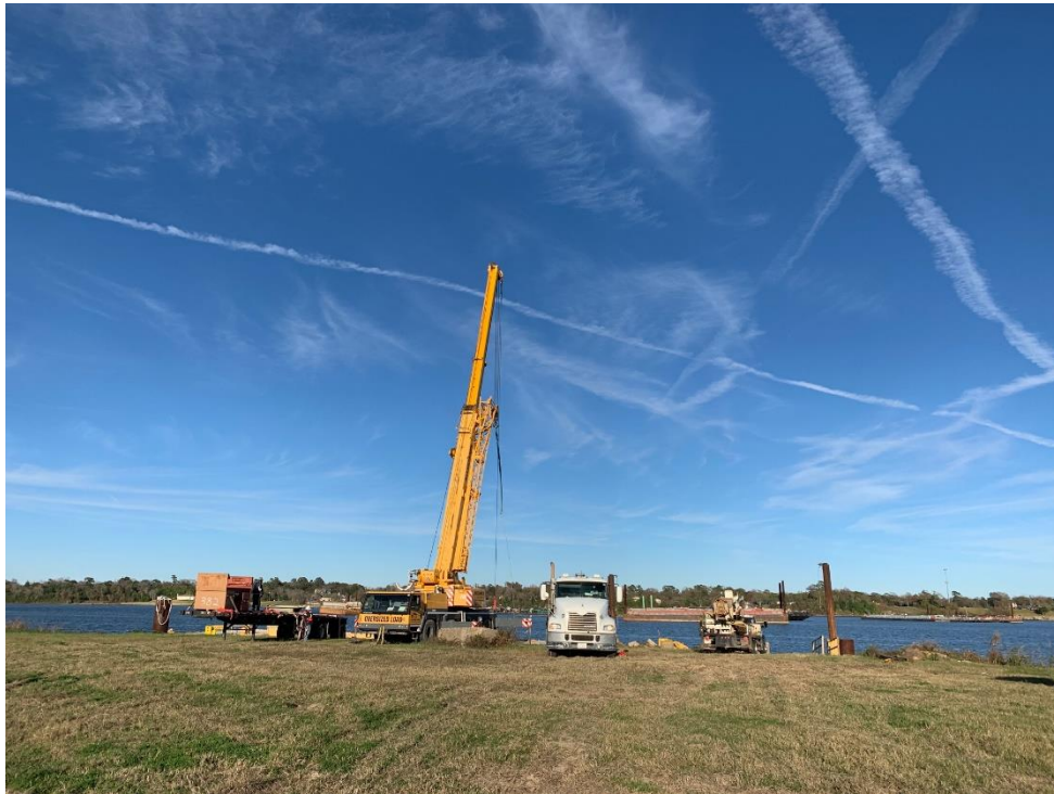
Photo 16 - Preparing transfer of drilling rig to barge.
