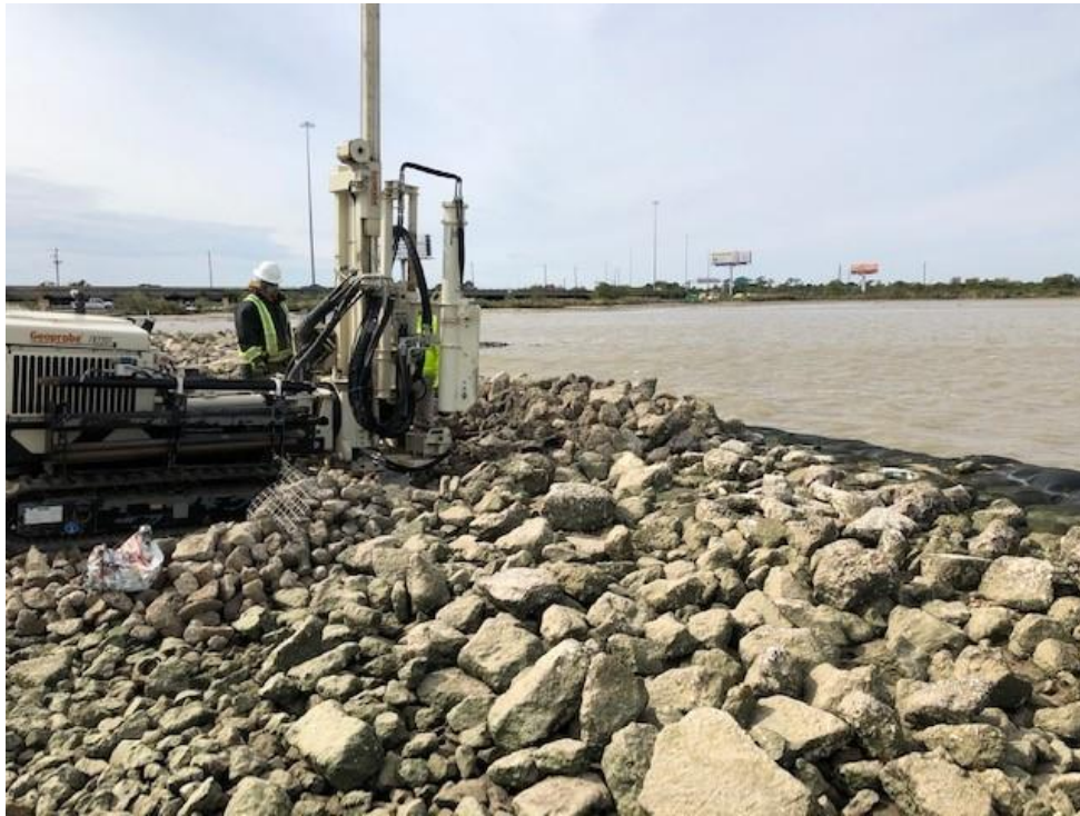
Photo 9 - Drill Crew collecting sample at location SJSB071.
