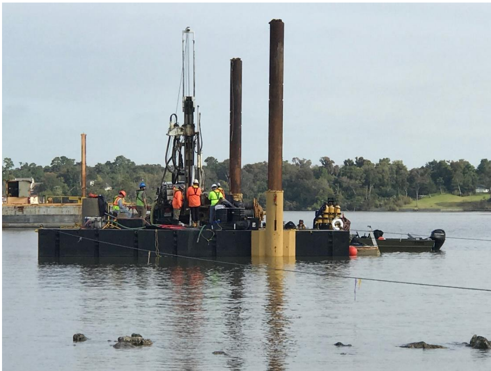
Photo 8 - Drill crew performing geotechnical sampling on barge, GHD oversight.
