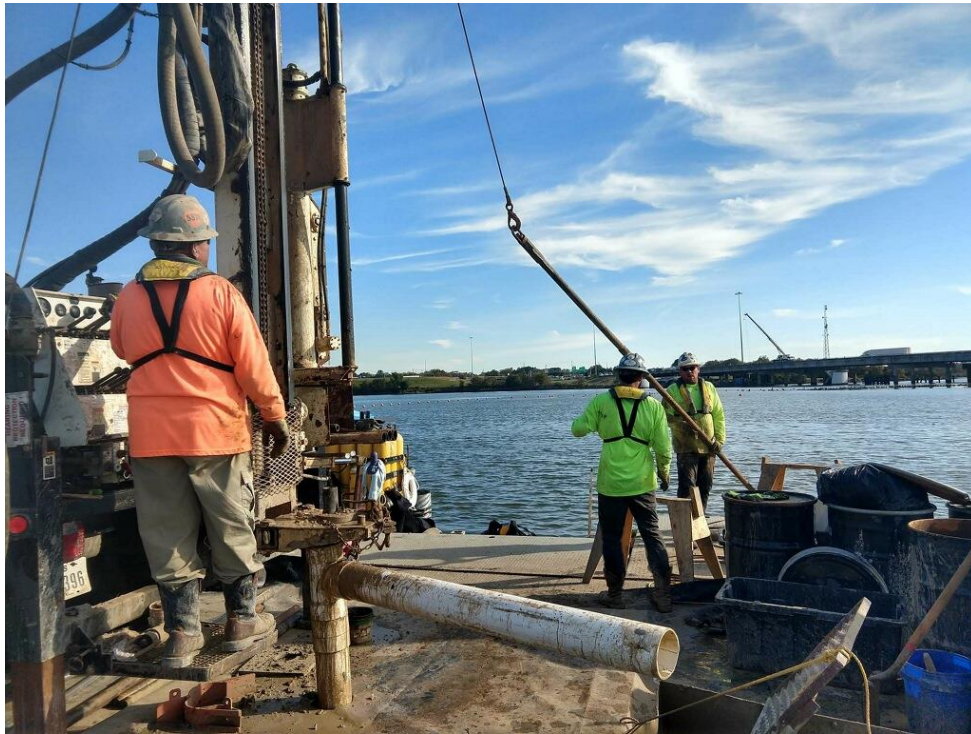
Photo 11 - Drill crew collecting samples from barge using rotary method.
