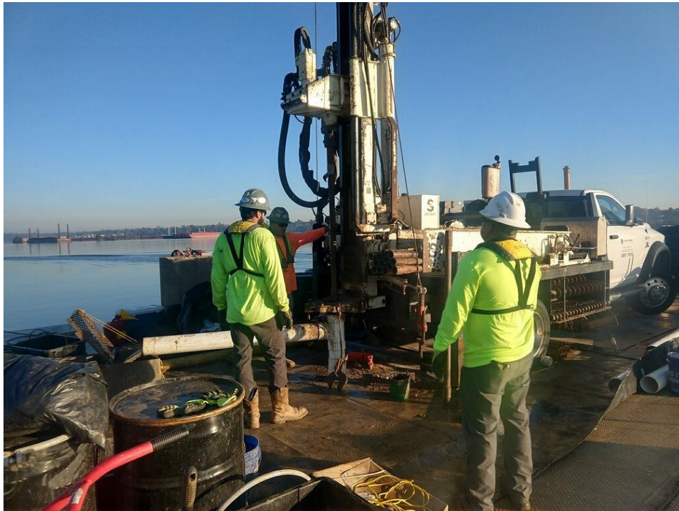
Photo 12 - Crew drilling borehole from barge using rotary method.
