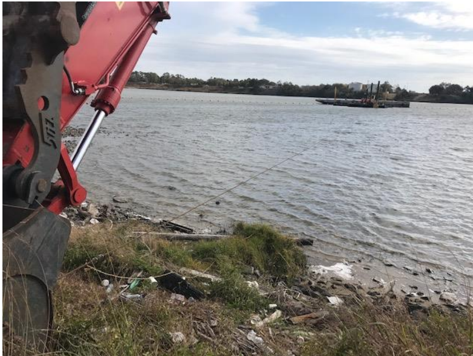
Photo 14 - View of barge anchored to excavator.
