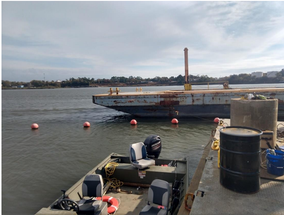
Photo 15 - View of spud barge anchoring drilling rig.
