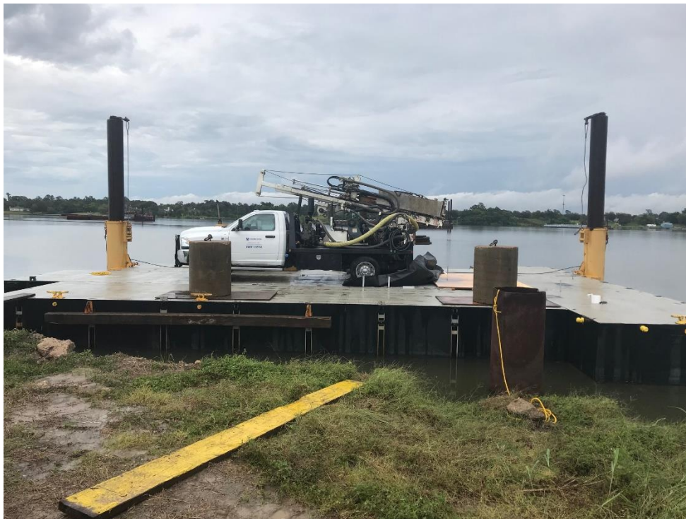
Photo 6 - View of drilling rig on barge.
