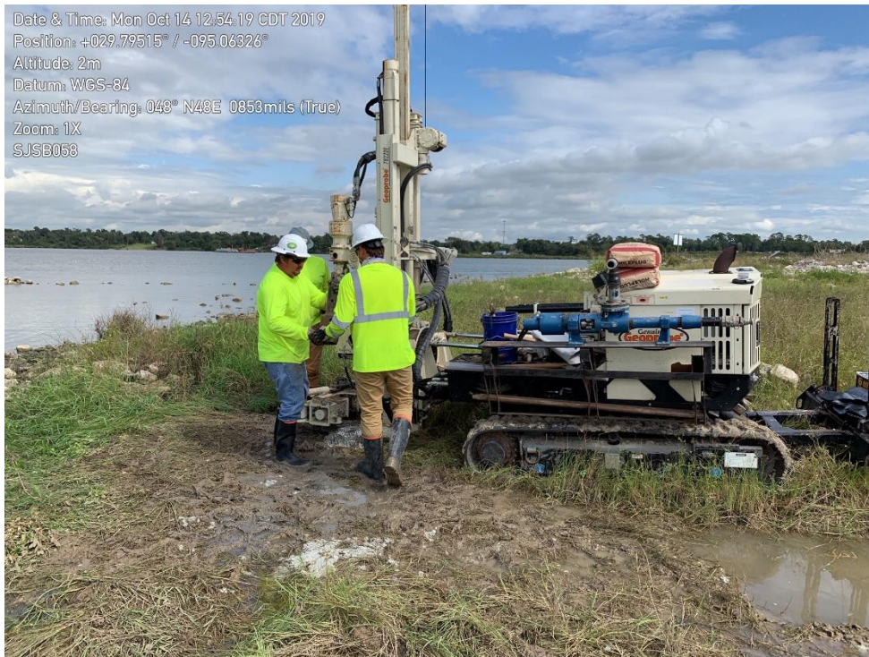
Photo 4 - Drill crew performing surface completion.
