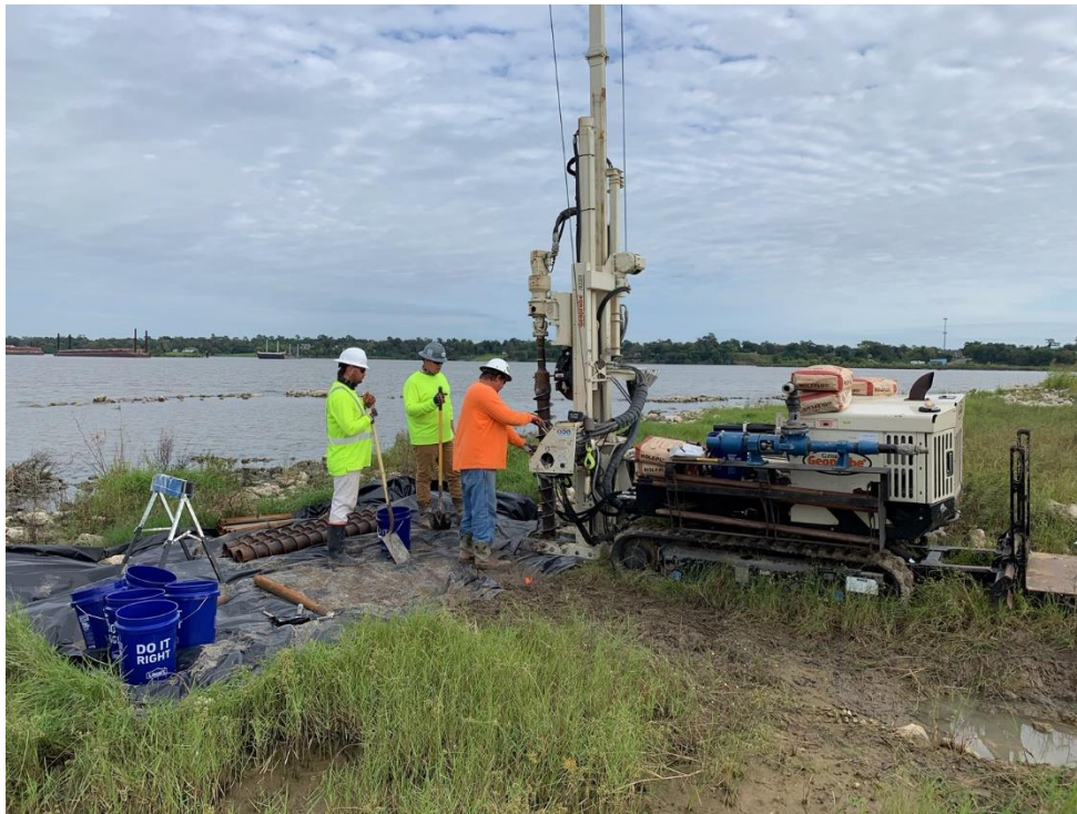
Photo 5 - Drill crew collecting samples using hollow-stem auger method.
