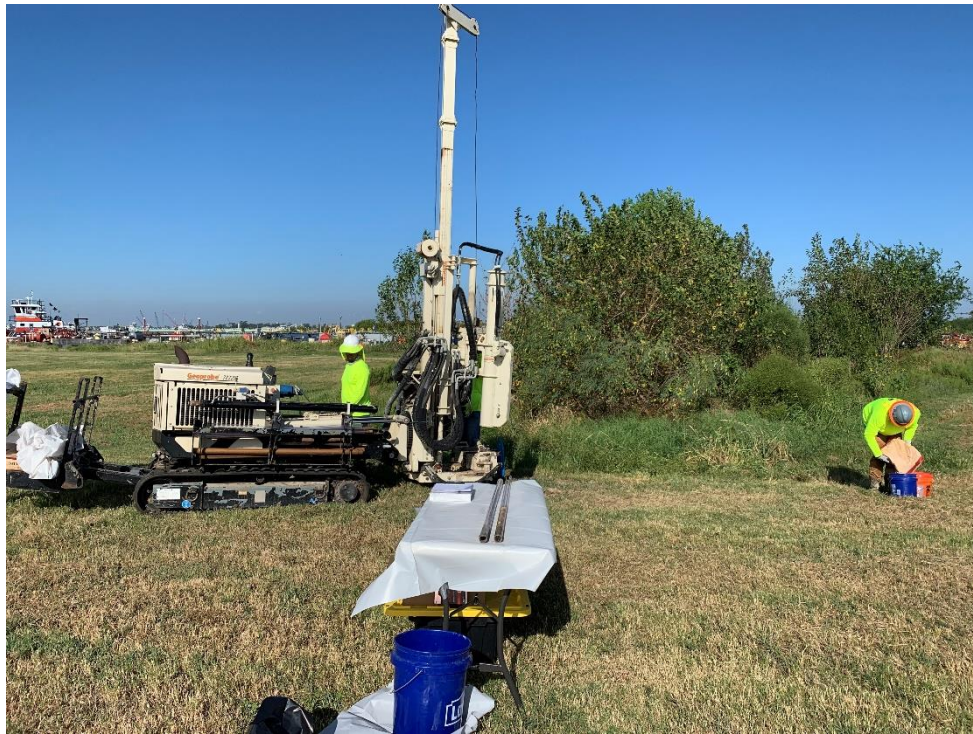
Photo 3 - Drill crew collecting samples at location SJGB029 using direct push technology.
