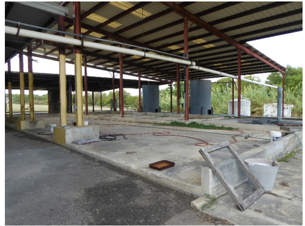
Covered Loading and Storage Area (Building A, east side)
