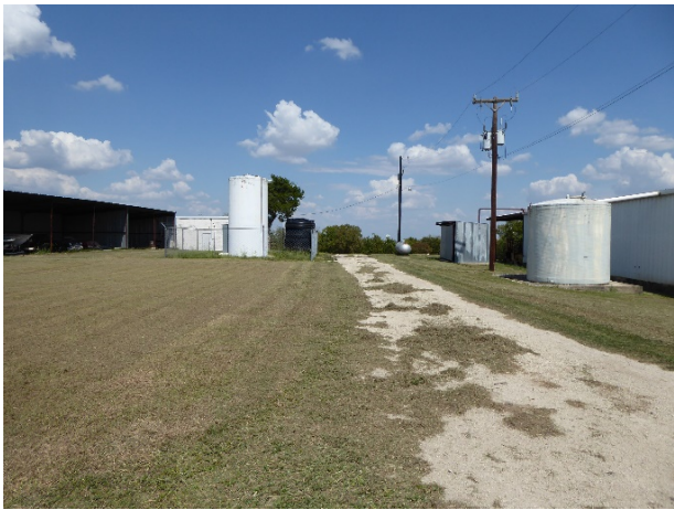
Internal Driveway on Site
