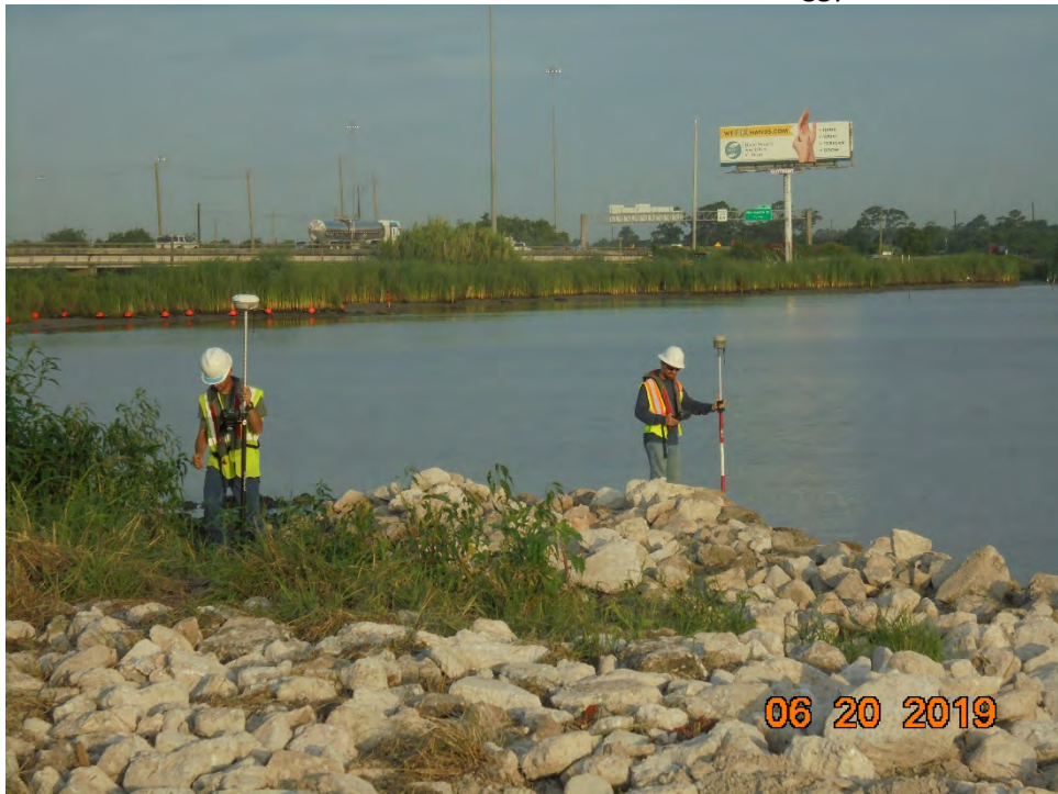
Photo 2 – Post-construction topographic surveying of the ACBM installation area
