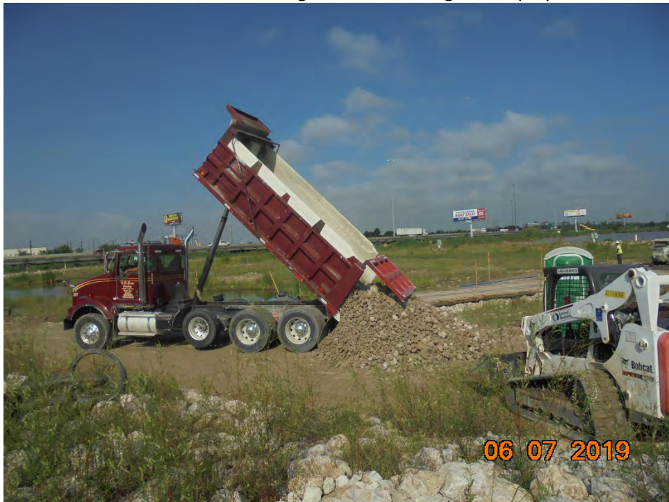
Photo 4 – Delivery of riprap near the grout pumping platform
