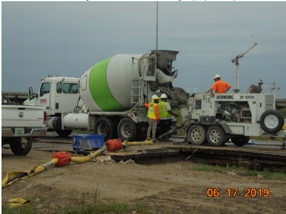
Photo 4 – Concrete grout being offloaded from delivery truck into grout pump
