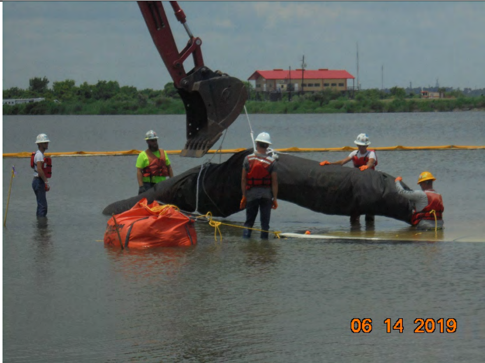
Photo 5 – Lowering of ACBM form 405 into the water for unrolling and positioning
