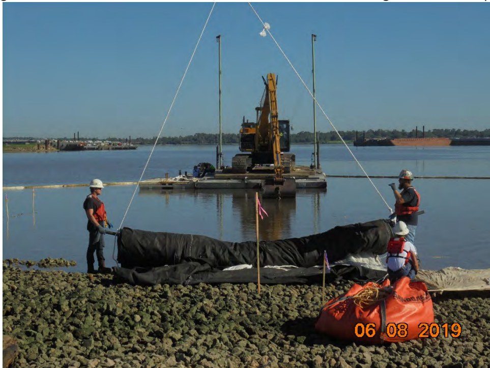
Photo 5 – Positioning of ACBM form 210 for unrolling
