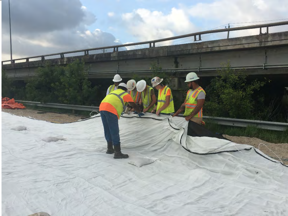
Photo 2 – Sewing of geotextile fabric to ACBM form during mattress assembly
