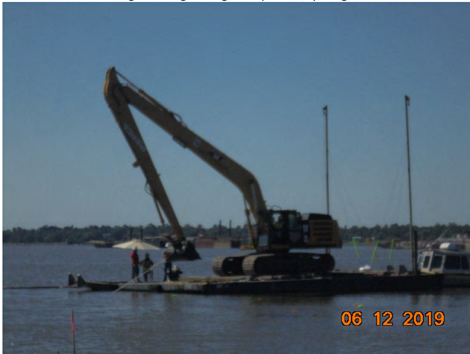
Photo 4 – Barge-mounted excavator assisting with the underwater unrolling of ACBM form 305
