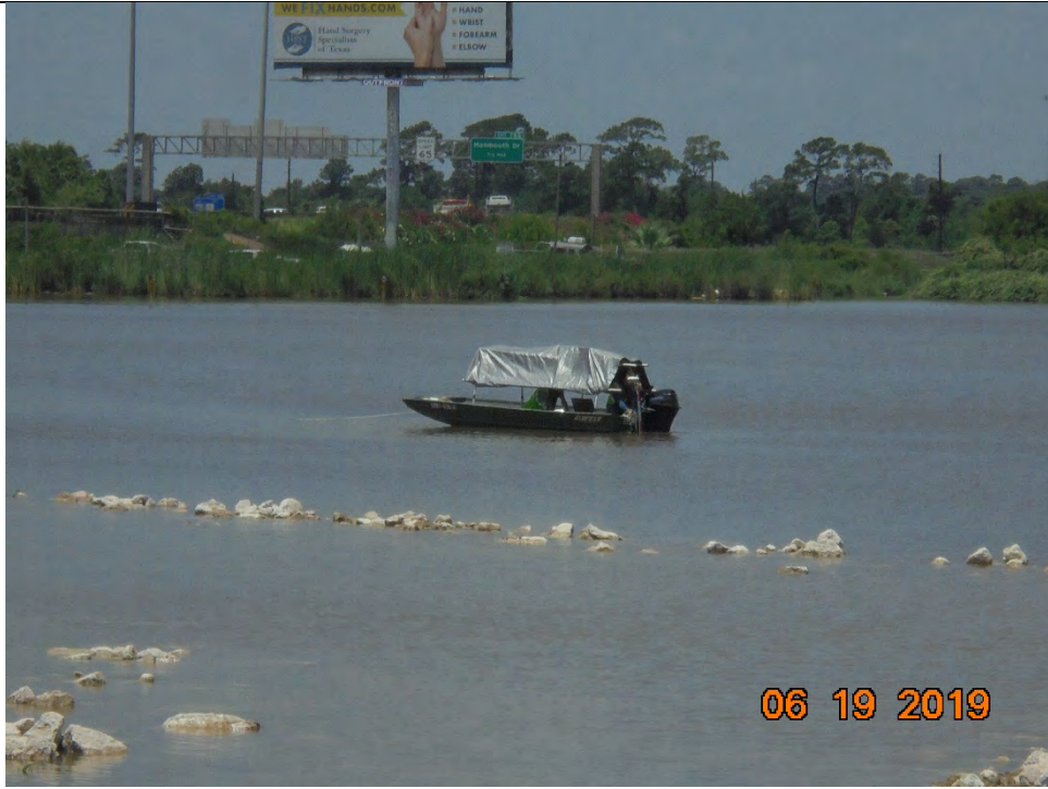
Photo 6 – Post-construction hydrographic surveying of the ACBM installation area
