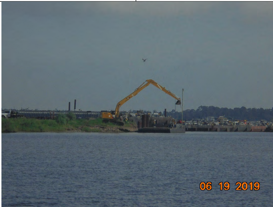
Photo 1 – Disassembly of spud barge components in preparation for demobilization
