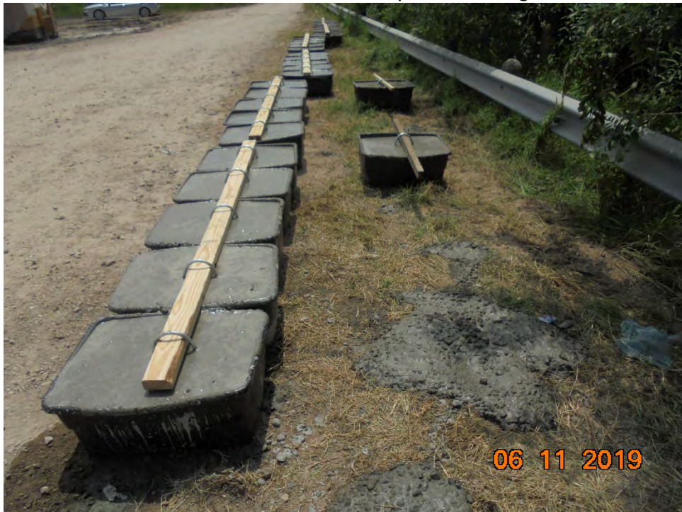
Photo 4 – Filled anchor forms with lifting eyes set in place
