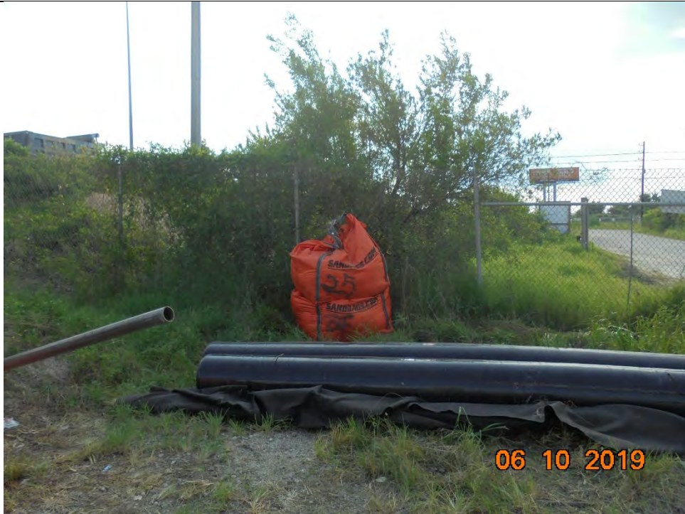
Photo 3 – Supersacks of sandbags placed in front of hole in security fence
