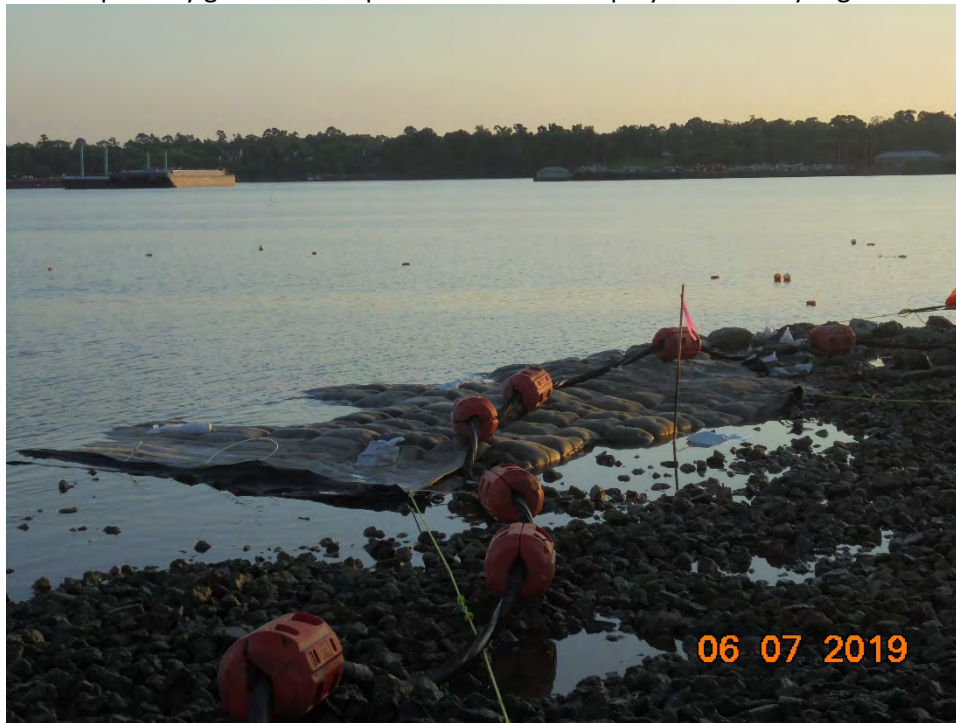
Photo 2 – Grouted ACBM panels visible during morning low tide
