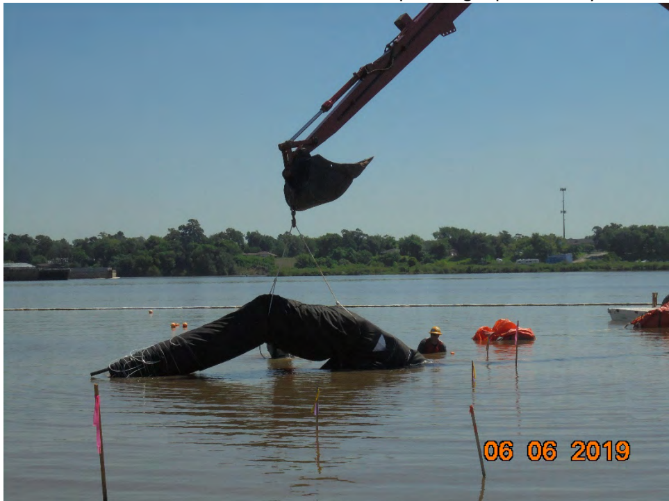
Photo 4 – ACBM form 207 being lowered into the water for positioning and unrolling
