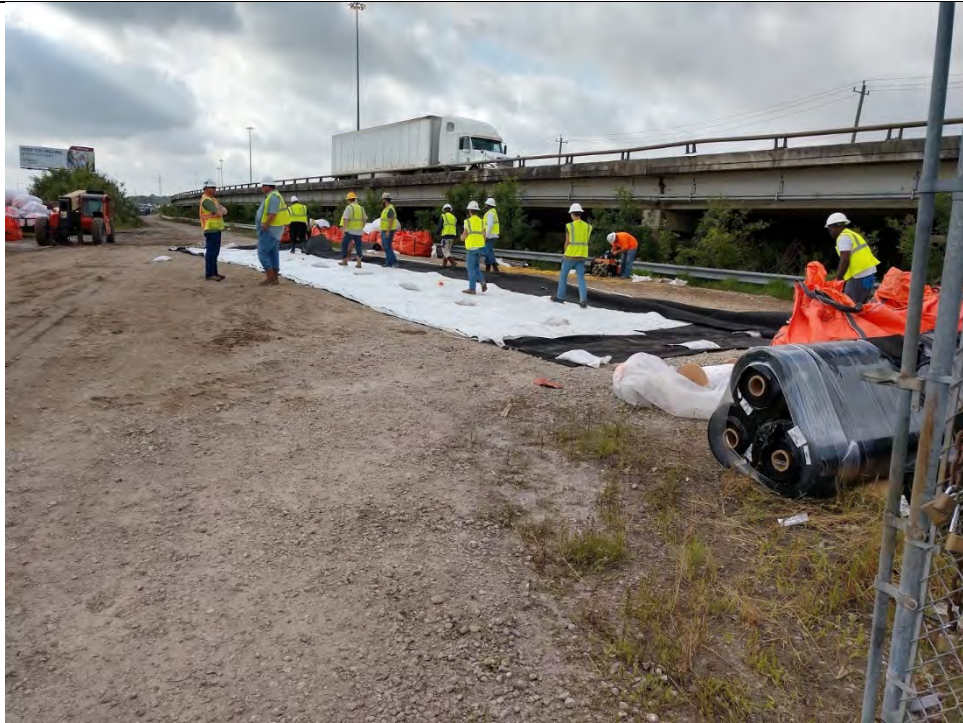
Photo 2 – ACBM mattress form assembly
