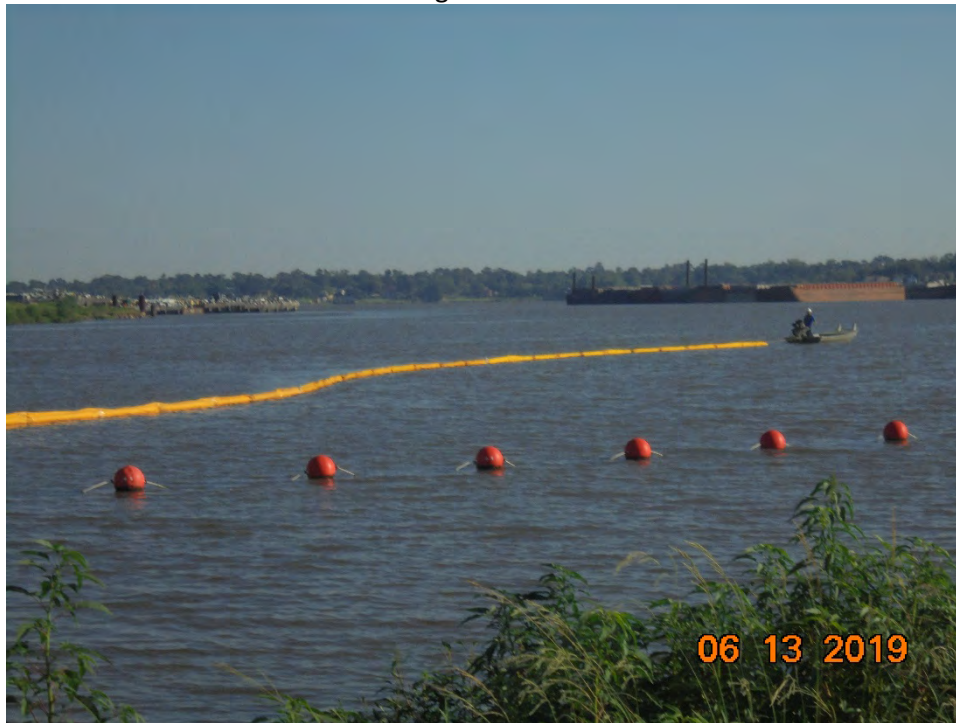
Photo 2 – Deployment of silt curtain around the ACBM installation work area
