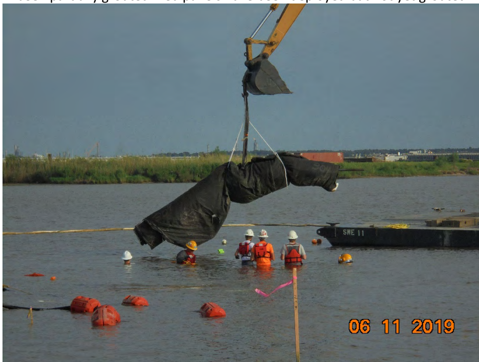
Photo 2 – ACBM form 304 being lowered into the water for positioning and unrolling
