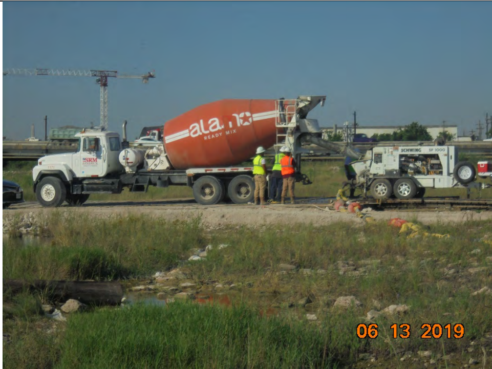
Photo 3 – Concrete grout being offloaded from delivery truck into the grout pump
