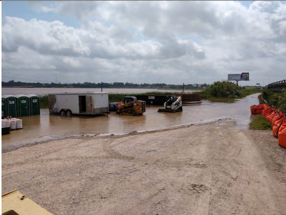
Photo 4 – Incoming tide at worksite.
