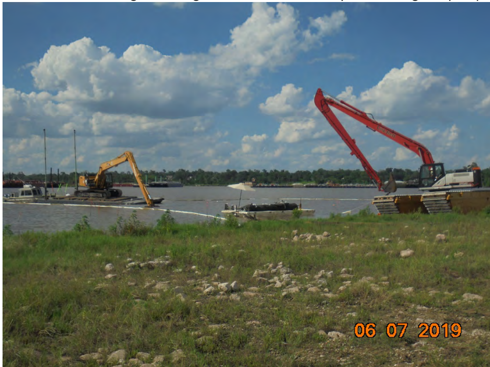
Photo 6 – Marsh buggy assisting with the positioning of ACBM form 209 during deployment
