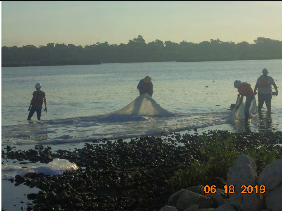
Photo 3 – Deployment of additional ACBM panel over gap between panels 209, 210, and 301
