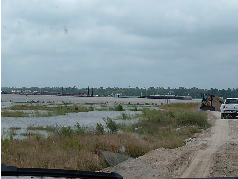
Photo 4 – Access road with incoming tide
