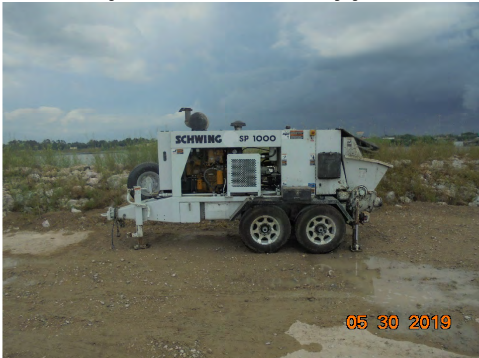
Photo 3 – CCI's grout pump staged near ACBM installation site
