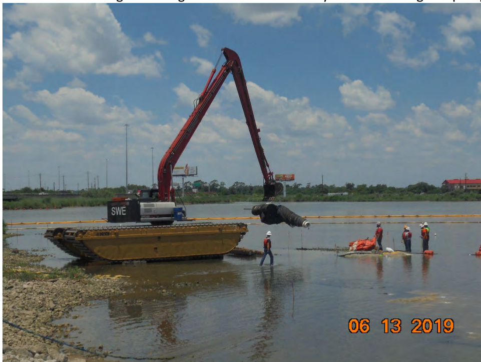
Photo 4 – Marsh buggy preparing to place ACBM form 401 into the water during deployment operations
