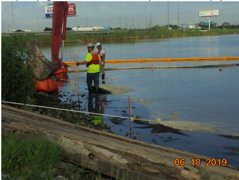
Photo 2 – Repositioning of ACBM forms 410 and 411 prior to grouting
