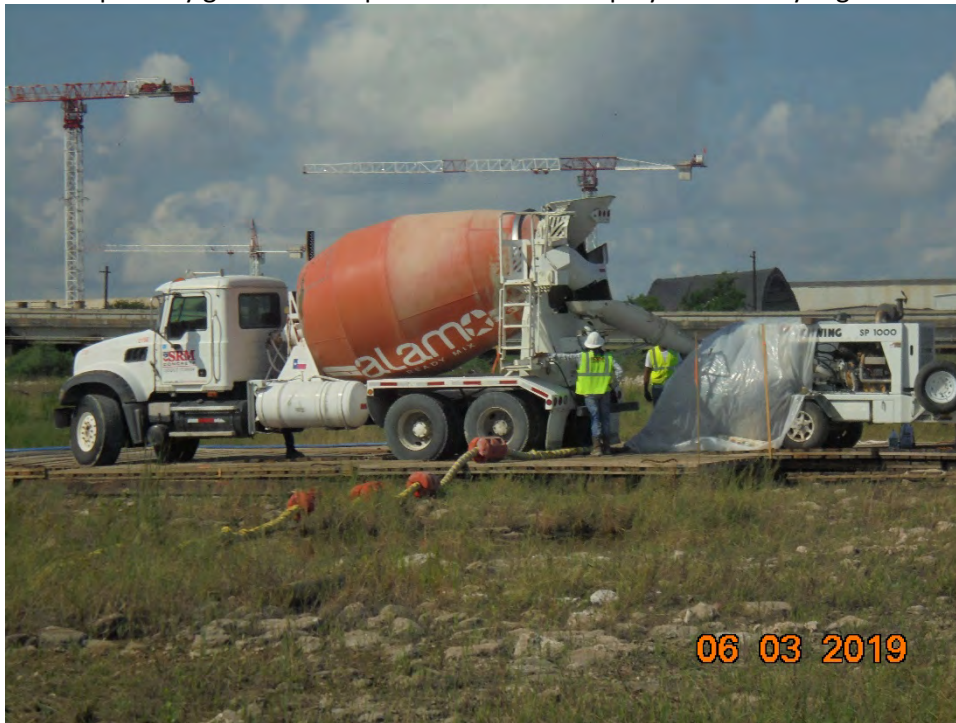
Photo 2 – Concrete being offloaded into grout pump during ACBM panel grouting
