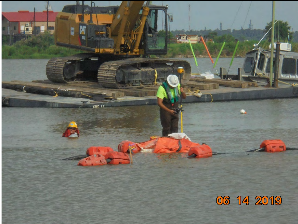
Photo 3 – Surveying of grouted extents of installed ACBM panels
