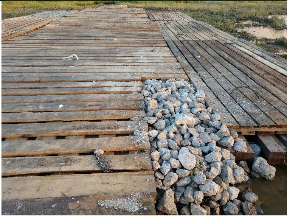
Photo 4 – Crane mats at installation site
