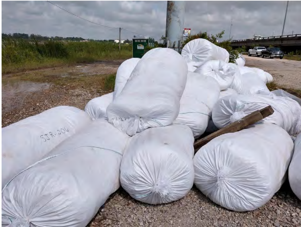
Photo 1 – Geotextile fabric rolls for ACBM.
