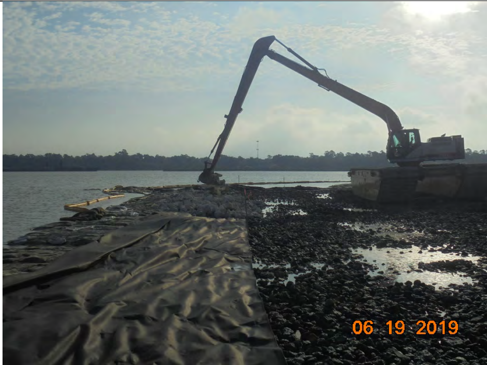
Photo 2 – Placement of riprap armor along the southern edge of installed ACBM
