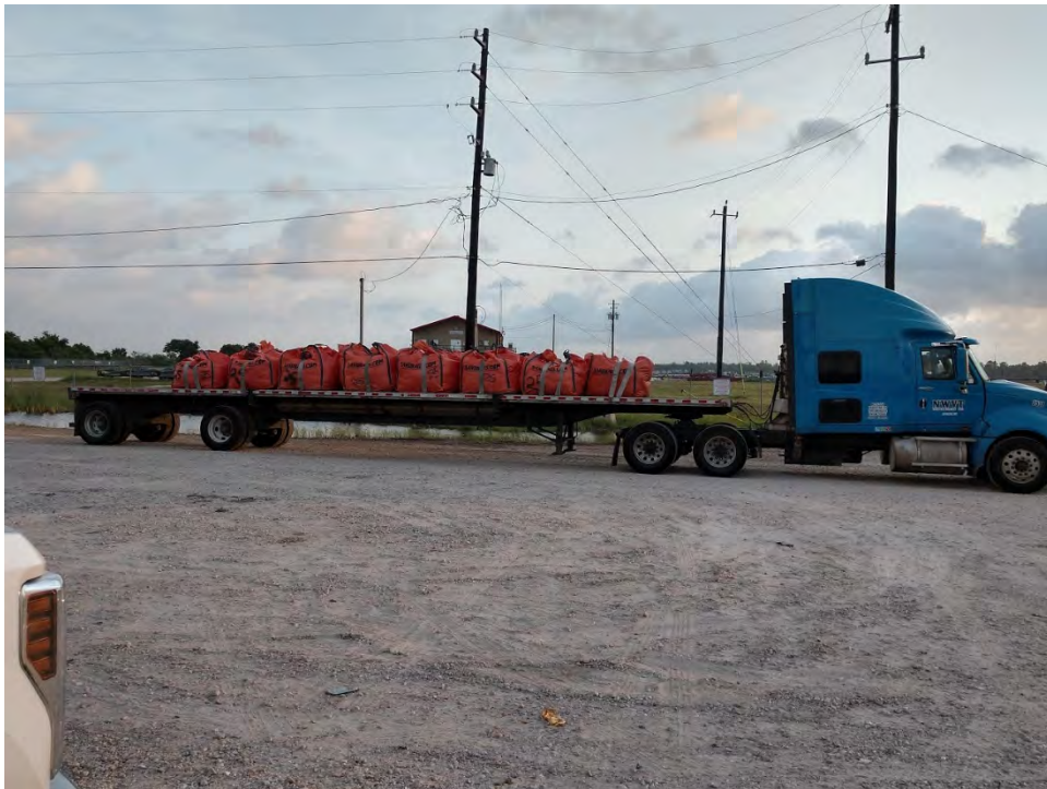
Photo 1 – Sand bags for ACBM construction.
