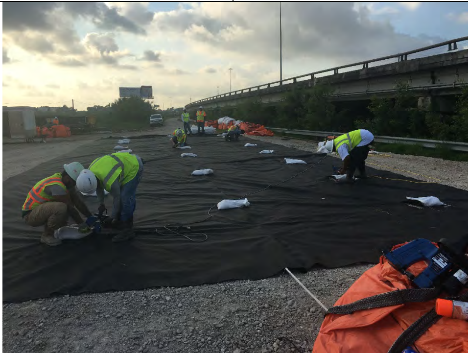
Photo 1 – Sewing of anchoring sandbags to geotextile fabric during ACBM mattress assembly
