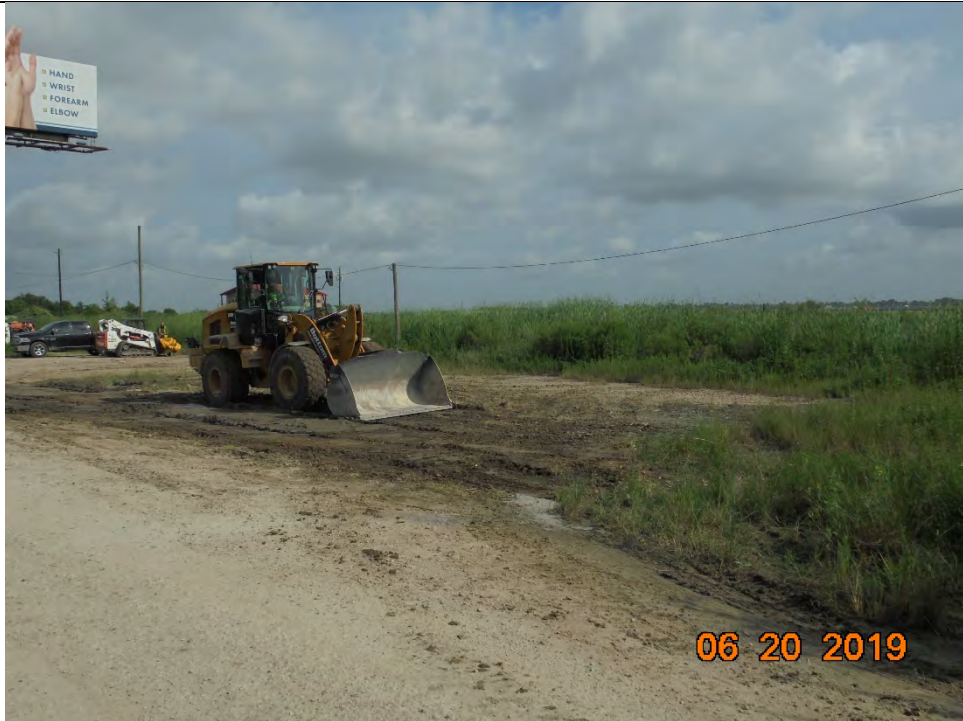
Photo 5 – Smoothing/backdragging of heavily trafficked northeastern portion of the staging area
