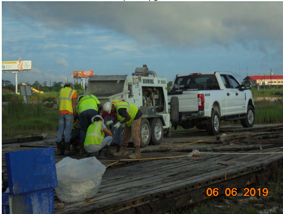
Photo 2 – Re-connection of discharge line to grout pump during morning setup activities
