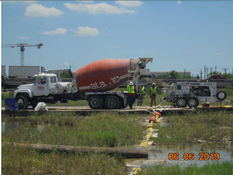
Photo 5 – Concrete grout being offloaded from delivery truck into the grout pump
