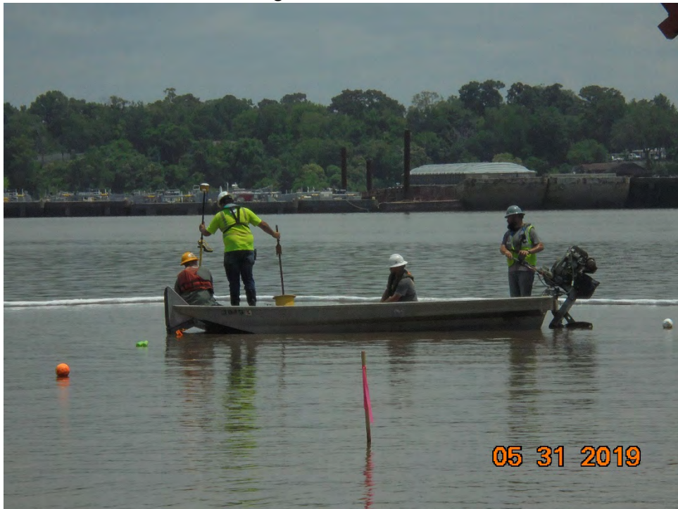
Photo 5 – GHD verifying position of unrolled ACBM form
