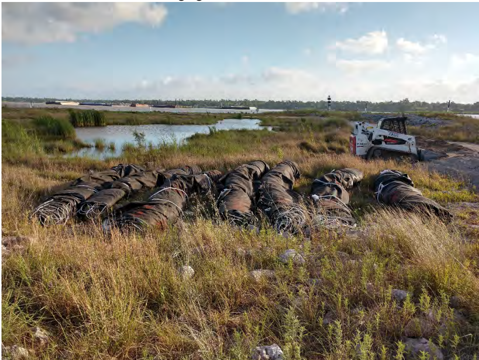
Photo 3 – Staging of ACBM near installation site
