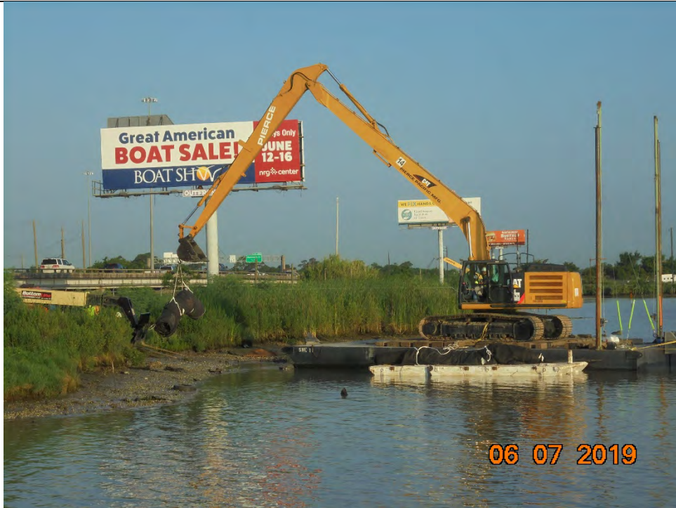
Photo 3 – ACBM form being loaded onto barge for deployment
