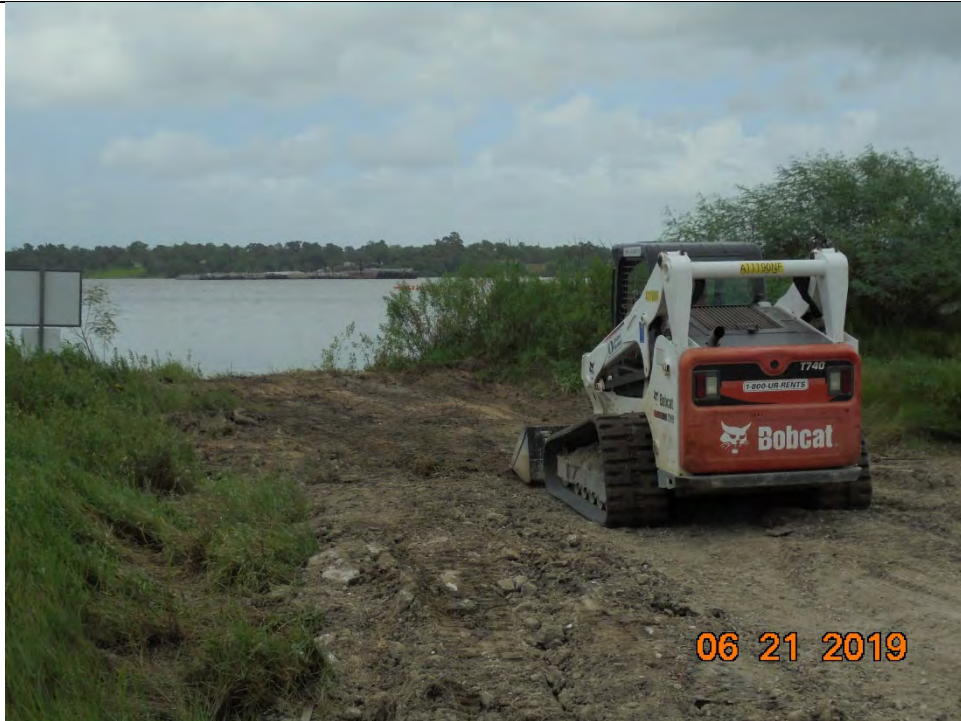
Photo 3 – Smoothing/backdragging of area previously used for barge-loading of materials
