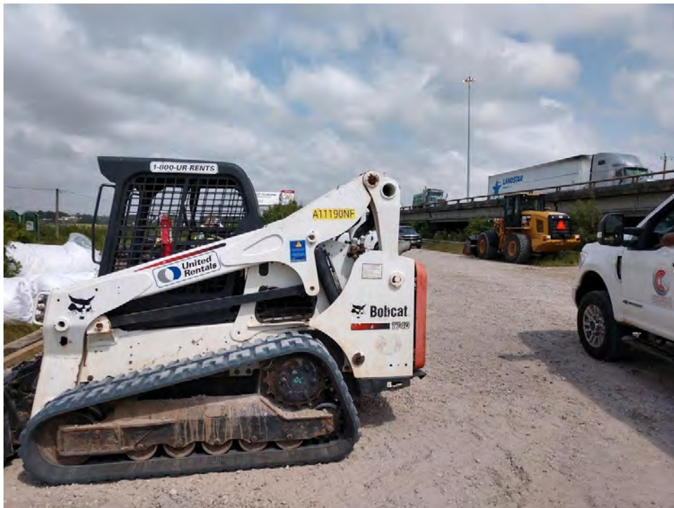
Photo 3 – Bobcat and Cat bulldozer.
