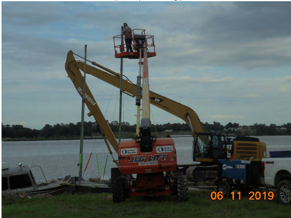
Photo 6 – Repairs to spud cable pulley being performed
