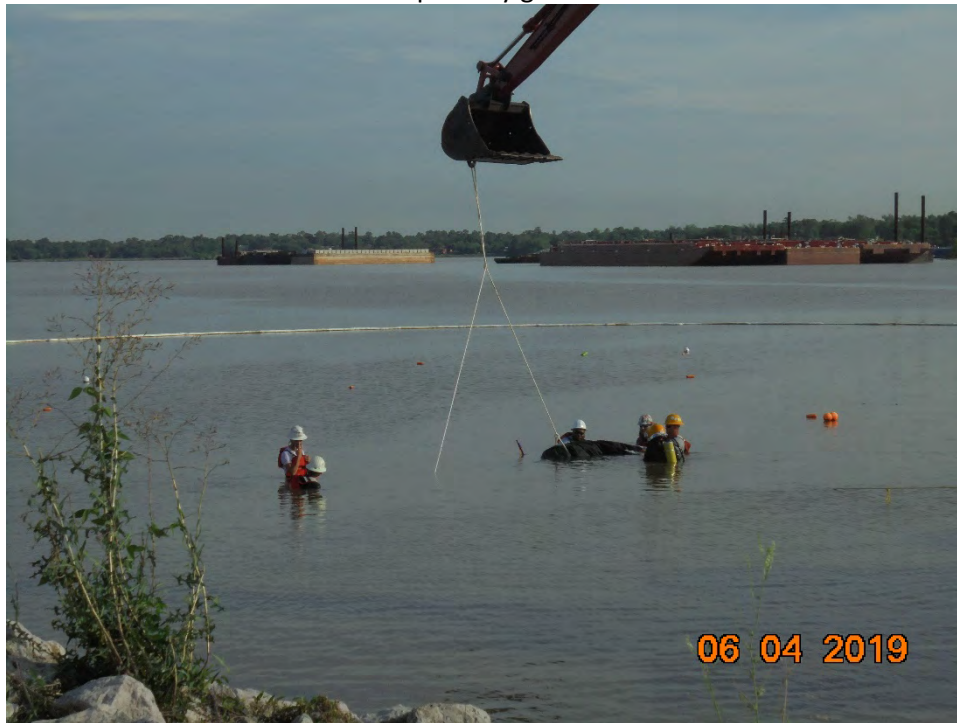
Photo 2 – Placement of ACBM form 205 in the water for unrolling and positioning
