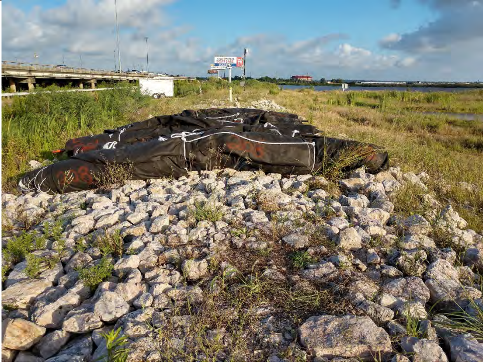
Photo 2 – Staging of ACBM near installation site
