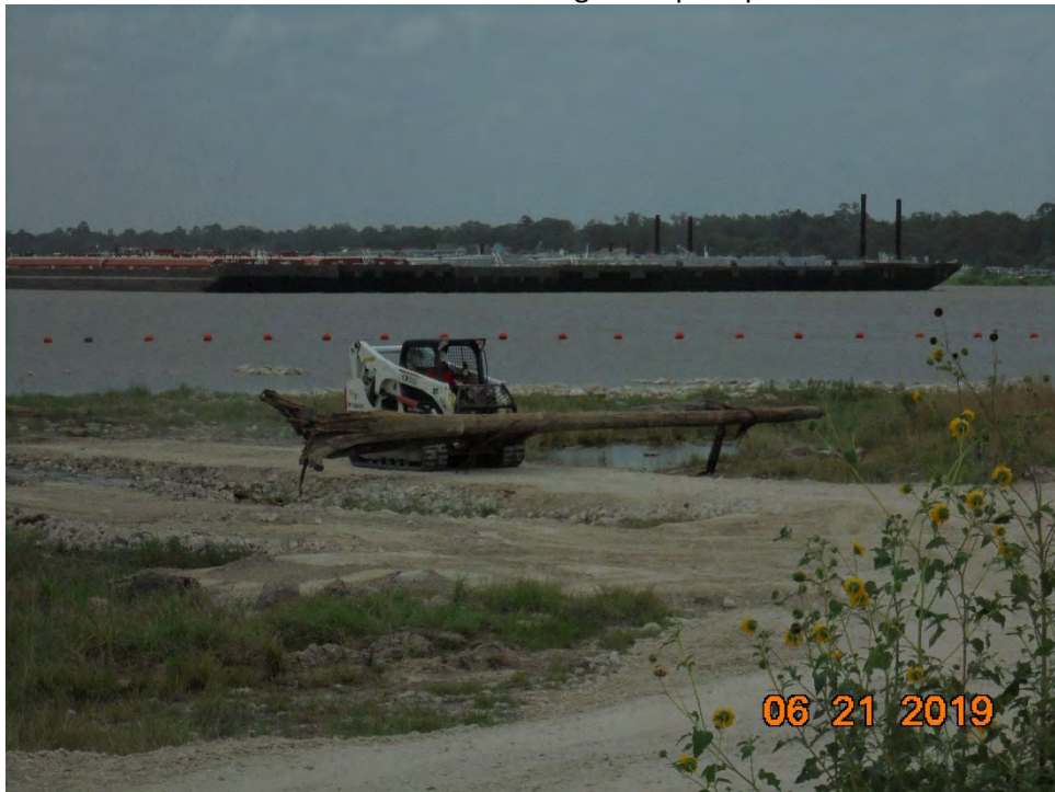
Photo 2 – Removal of logs near the shoreline of the ACBM installation area
