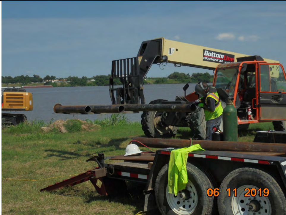
Photo 5 – Spud repairs being performed
