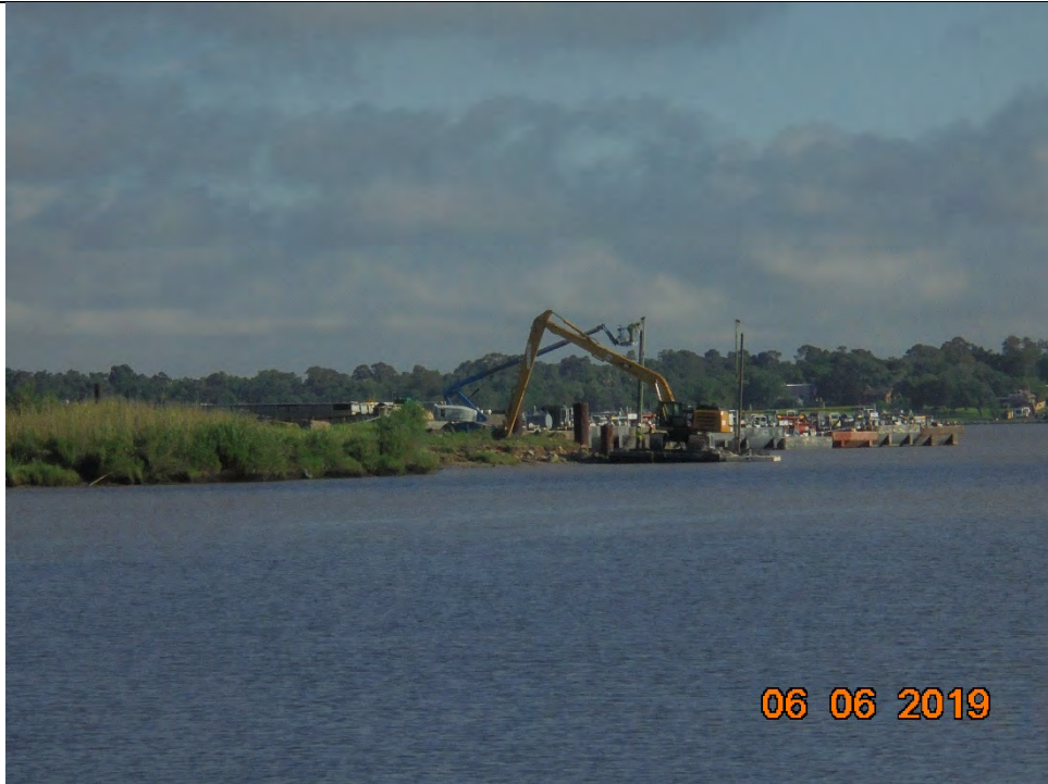
Photo 3 – Manlift-assisted maintenance of spud barge spud cable system
