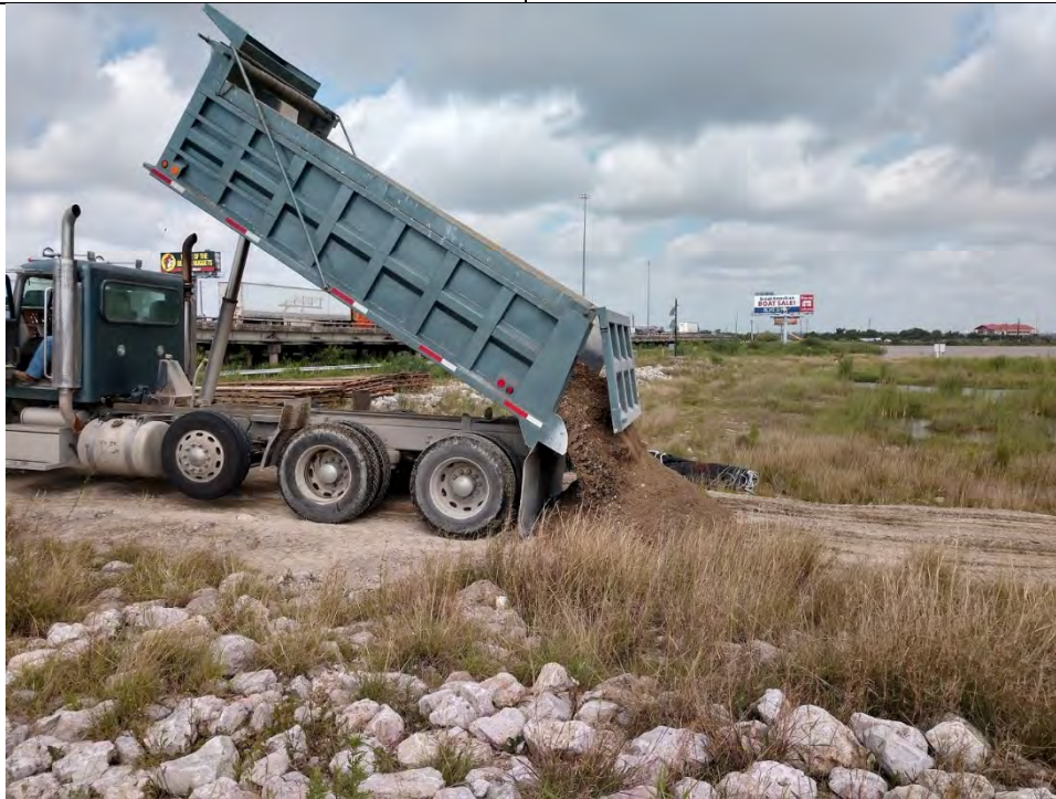
Photo 1 – Maintenance of construction access roadway
