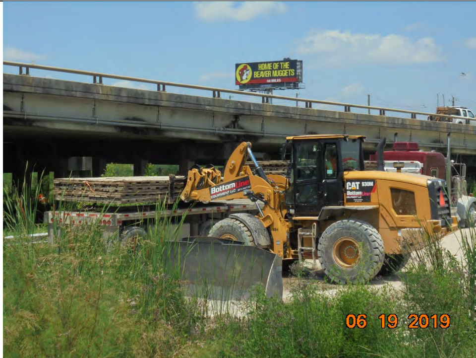
Photo 4 – Loading of board mats onto flatbed truck for removal from site
