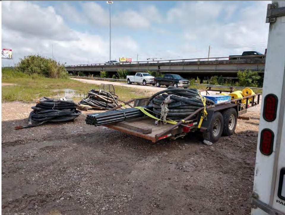
Photo 2 – Grouting hoses and roll-out pipes.
