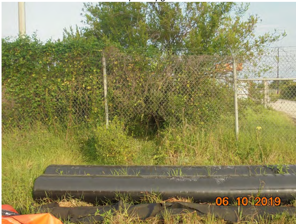
Photo 2 – Hole in security fence, observed during morning setup activities
