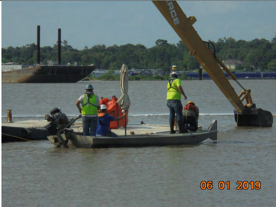
Photo 4 – GHD and CCI verifying position of ACBM panel
