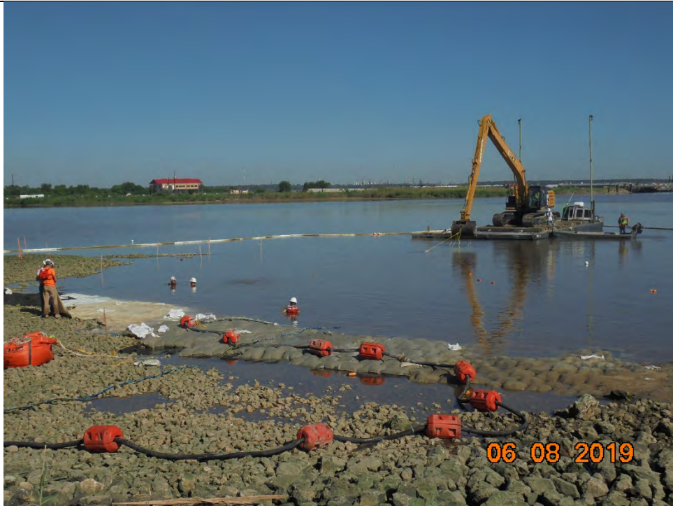
Photo 6 – Barge-mounted excavator assisting with the unrolling of ACBM form 210
