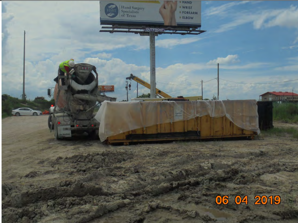
Photo 5 – Concrete truck being washed out into designated onsite roll off box
