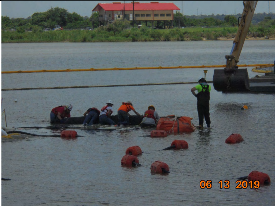
Photo 5 – Unrolling of ACBM form 401 during deployment operations
