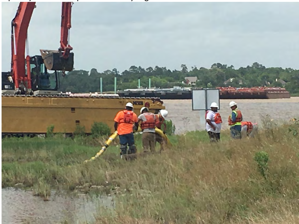
Photo 5 – Assembly of grout pump hoses near ACBM installation site
