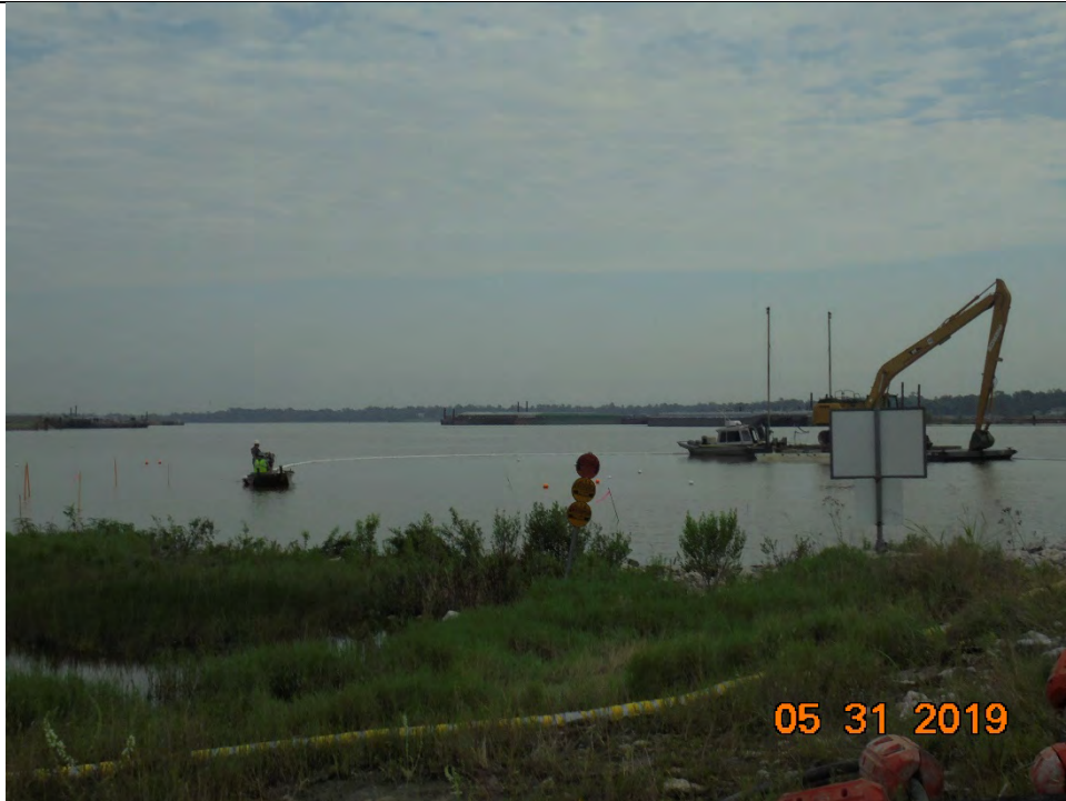
Photo 2 – Deployment of sorbent boom around ACBM installation work area
