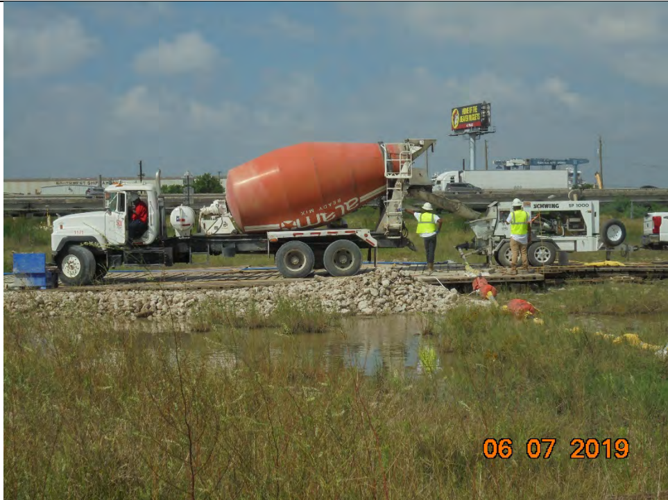
Photo 5 – Concrete grout being offloaded from delivery truck into grout pump
