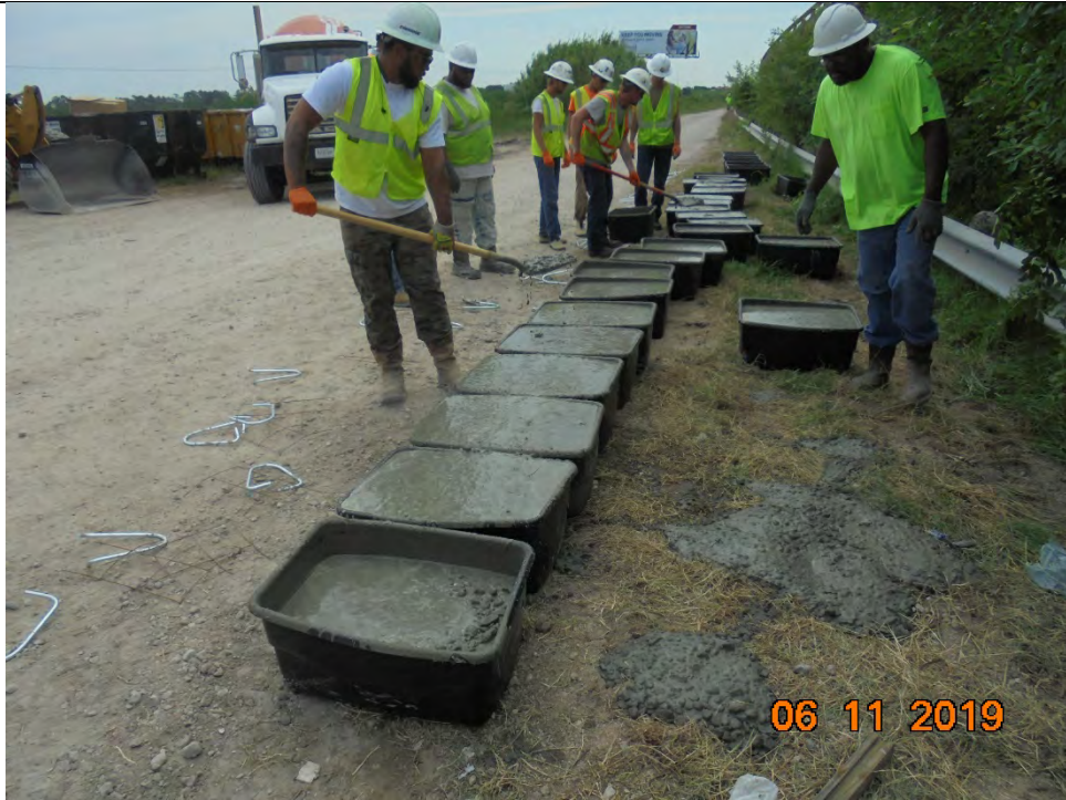
Photo 3 – Forms for concrete buoy anchors being filled
