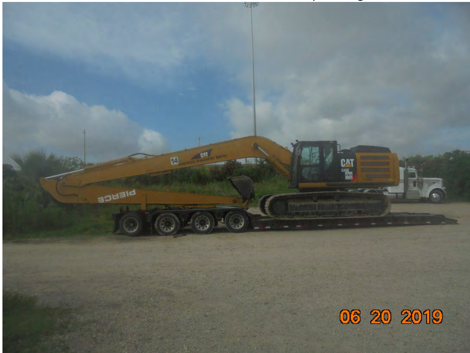
Photo 4 – Demobilization of SWE's long-reach excavator
