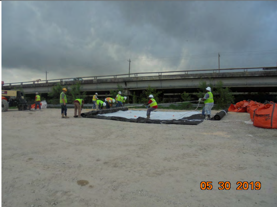
Photo 2 – Rolling of assembled ACBM mattress for staging at installation site
