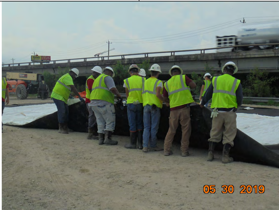
Photo 1 – Sewing of geotextile fabric to ACBM form during mattress assembly
