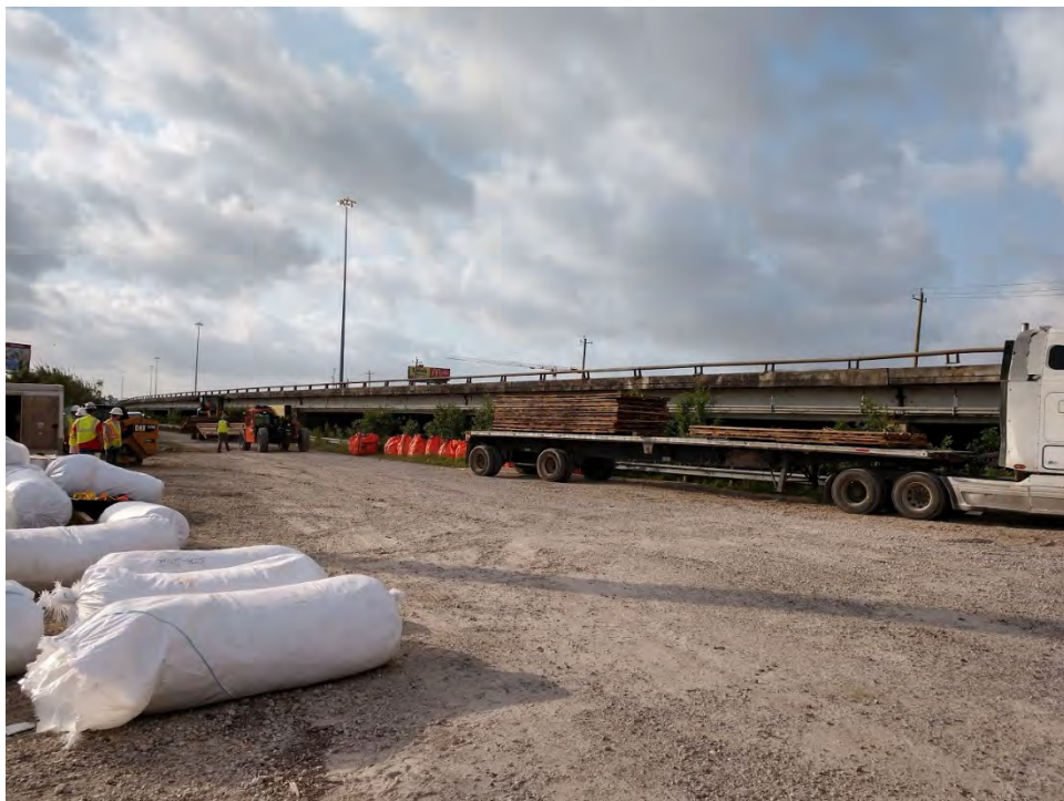
Photo 3 – Timber crane mats
