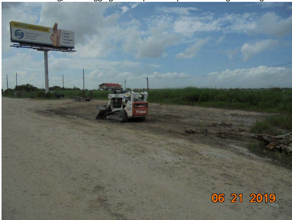
Photo 4 – Smoothing/backdragging of the northeastern corner of staging area
