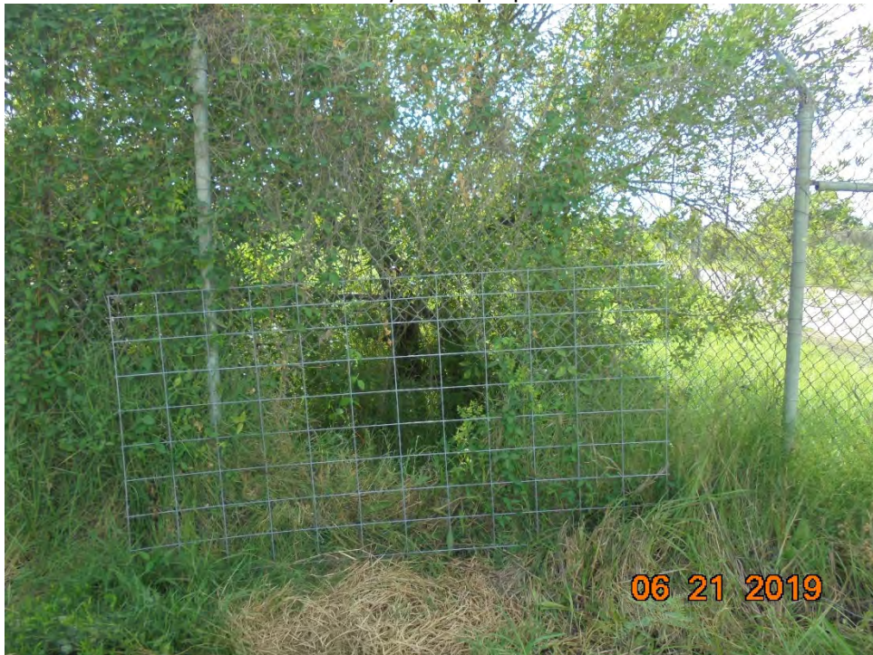
Photo 6 – Temporary wire-mesh patch installed over the hole in the security fence
