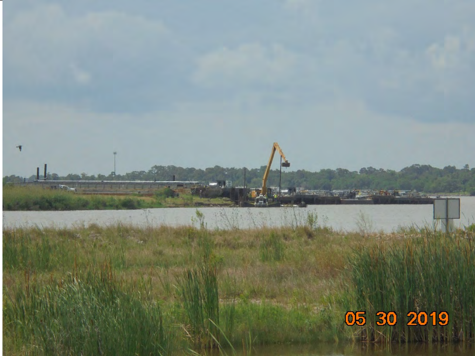
Photo 4 – Longer spuds being installed on SWE spud barge
