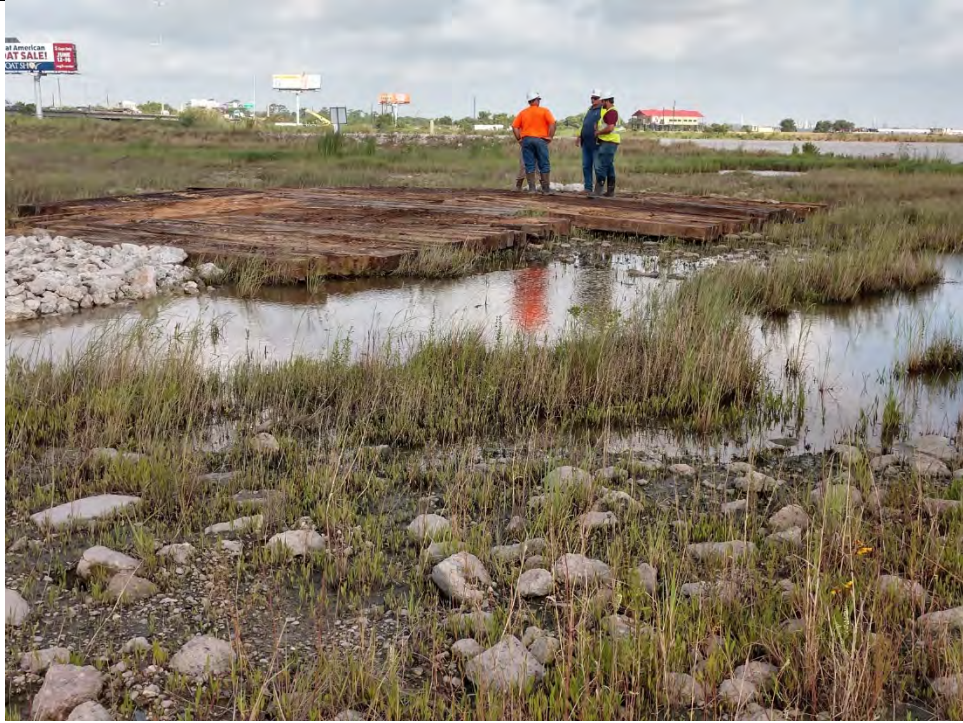
Photo 4 – Grout pump staging area.
