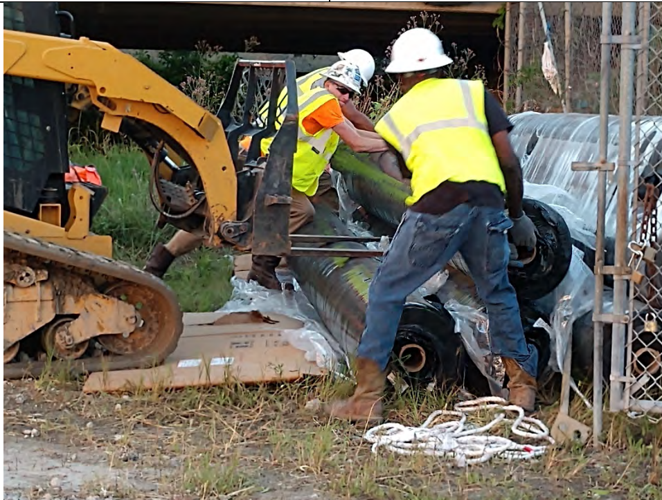
Photo 1 – Ongoing ACBM assembly
