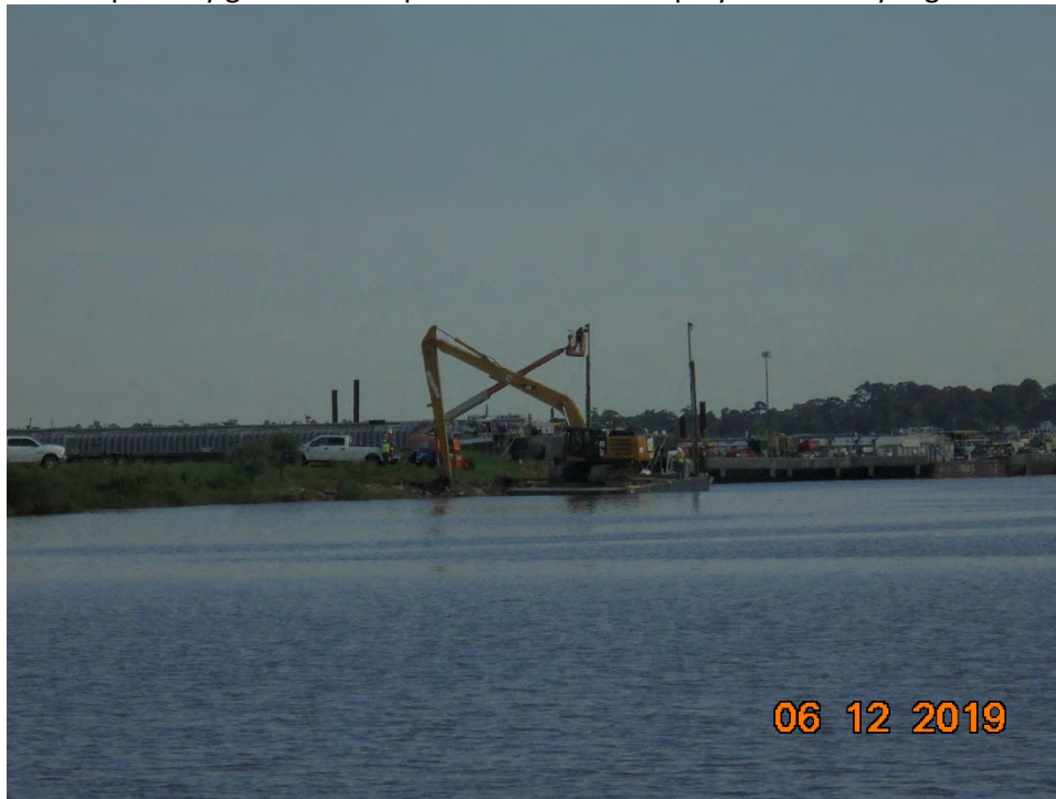
Photo 2 – Repairs to spud barge's spud cable pulley being performed
