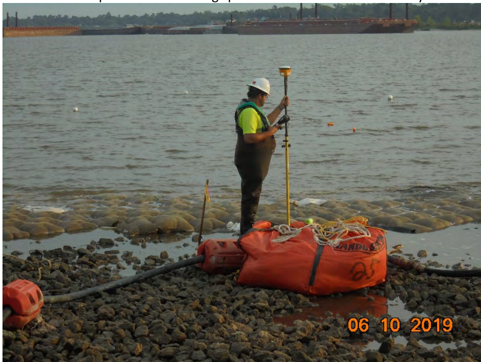
Photo 4 – Surveying of grouted boundaries of installed ACBM
