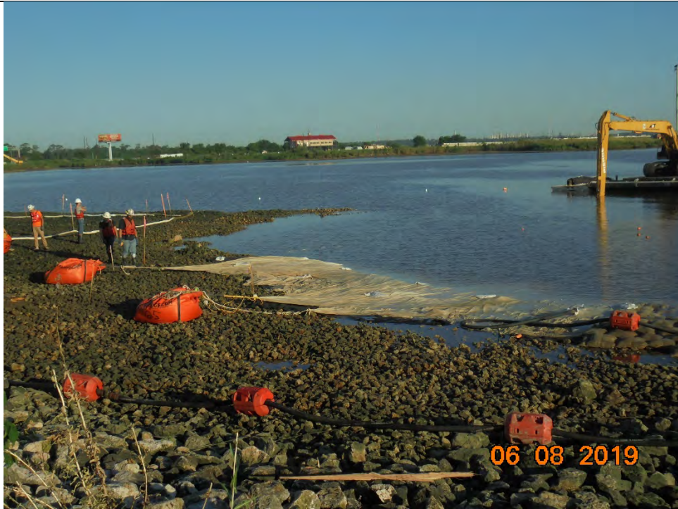
Photo 2 – Deployed ACBM forms 208 and 209 prior to the start of grouting operations
