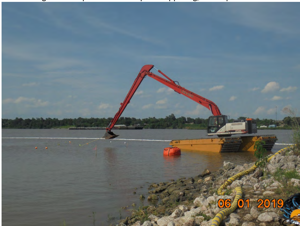
Photo 3 – SWE marsh buggy assisting with panel re-positioning after completion of zippering
