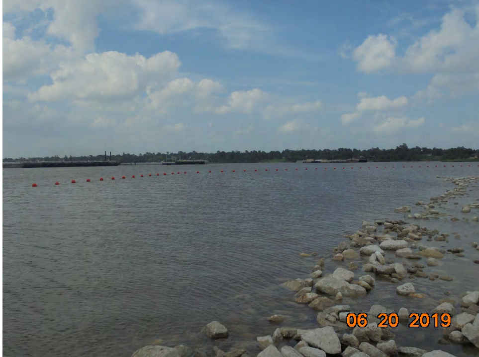
Photo 6 – Western-most portion of realigned perimeter buoys
