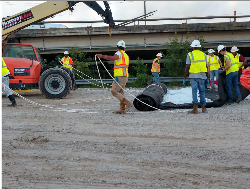
Photo 1 – Completion of ACBM form assembly
