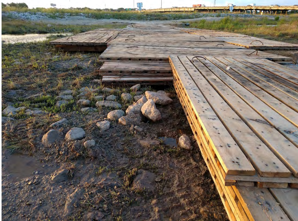
Photo 5 – Crane mats at installation site
