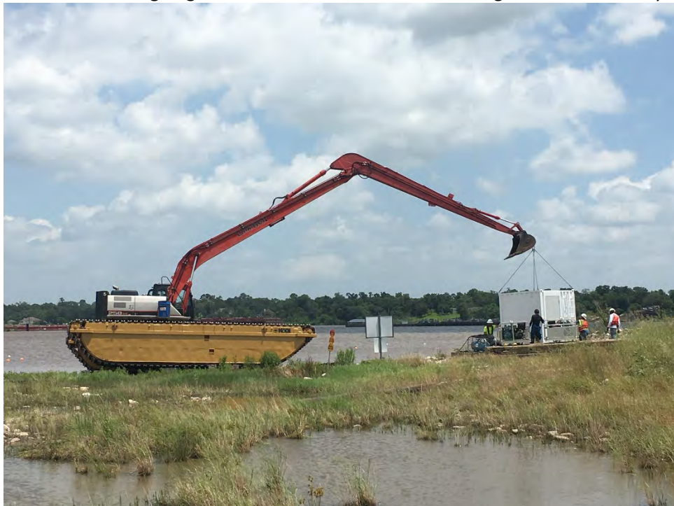
Photo 3 – Placement of dive equipment adjacent to ACBM installation site
