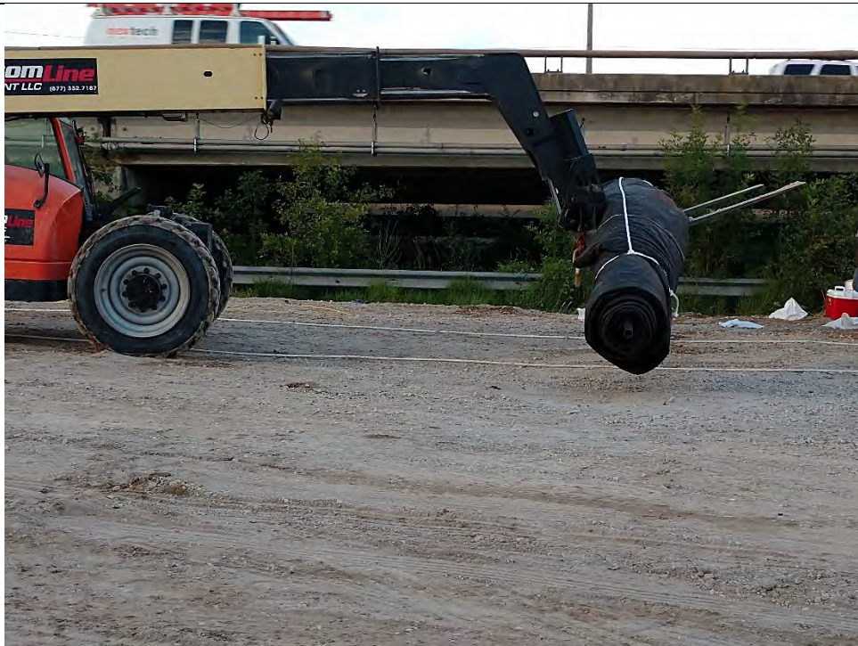
Photo 2 – Completed ACBM form assembly being moved to installation staging location
