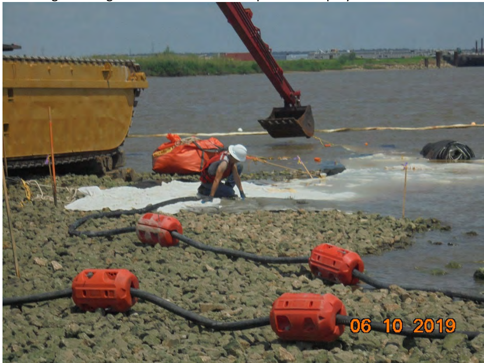
Photo 6 –Pumping of grout into ACBM form 301
