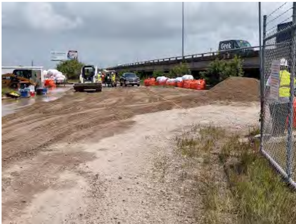
Photo 5 – Completion of laydown area maintenance
