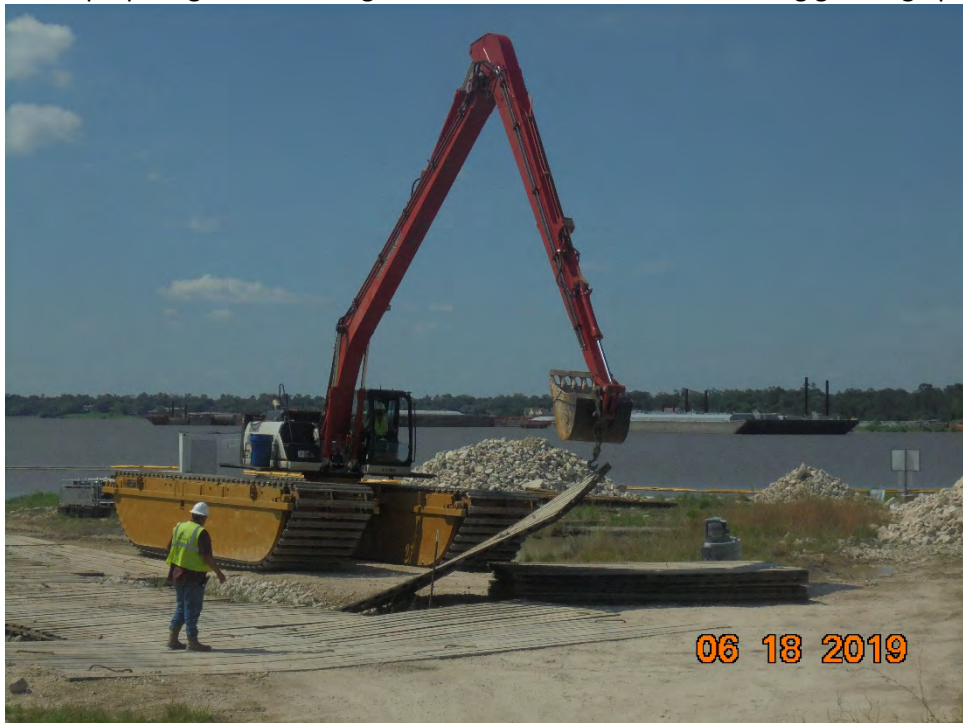
Photo 5 – Removal of board mats from the grout pumping pad
