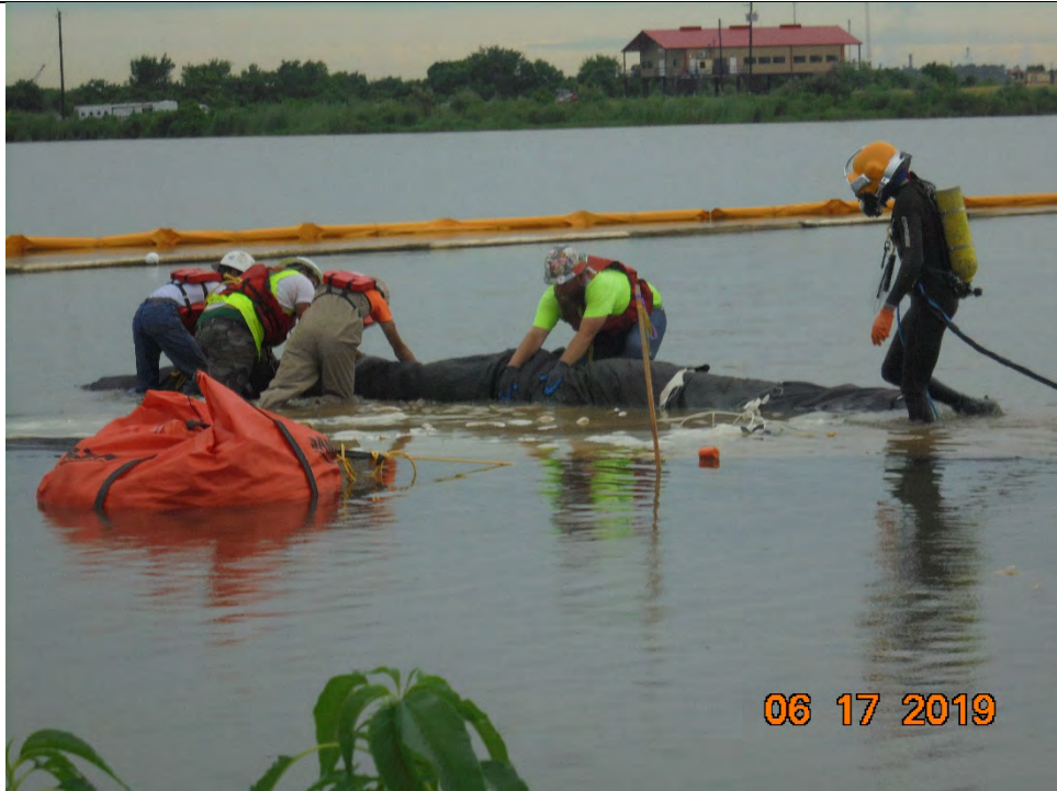
Photo 3 – Unrolling of ACBM form 407 during deployment operations
