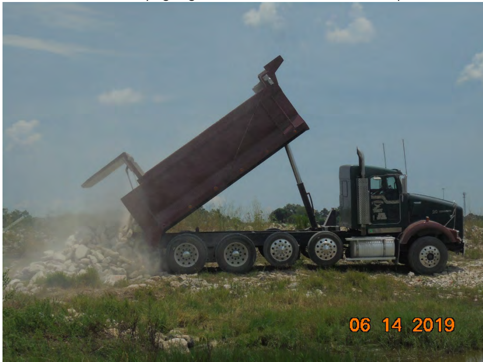
Photo 4 – Delivery of riprap for ACBM armoring
