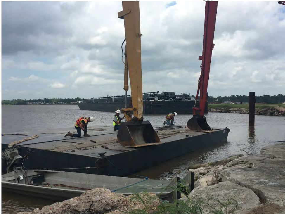
Photo 5 – Assembly of SWE spud barge
