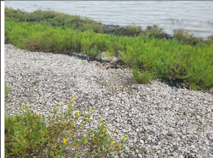
19 – South Inner Dike, viewing exposed geofabric
