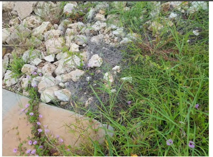
20 – Drainage channel, viewing slight erosion and vegetation on Northwest corner
