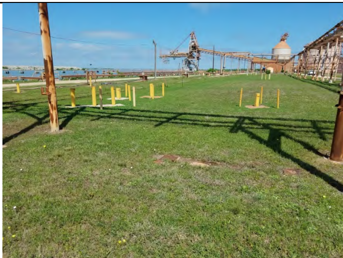
21 – View South to North, monitoring wells and recovery wells
