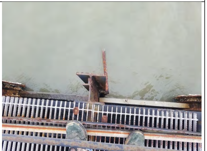
24 – South Decant Structure, viewing corrosion of angle iron
