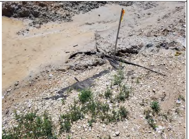
4 – North Inner Dike, viewing exposed geofabric
