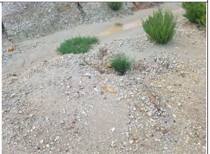
4 – North Inner Dike, viewing minor erosion
