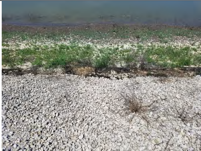
19 – South Inner Dike, viewing exposed geomembrane
