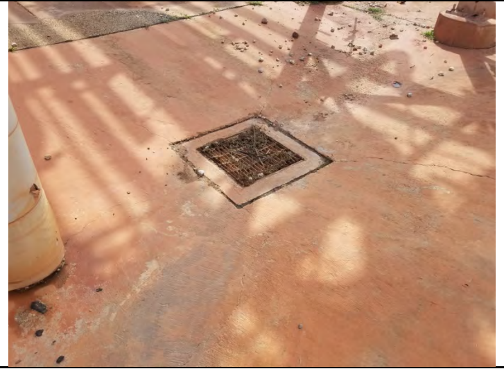
2 – R301, storm sewer drain
