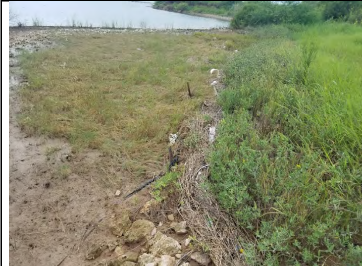
15 – Slope from cap to channel, viewing deteriorated silt fence
