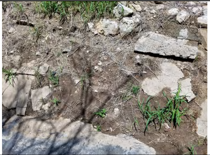
10 – Drainage channel, viewing deterioration of old channel
