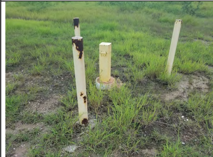
21 – O/W Separator, viewing monitoring well
