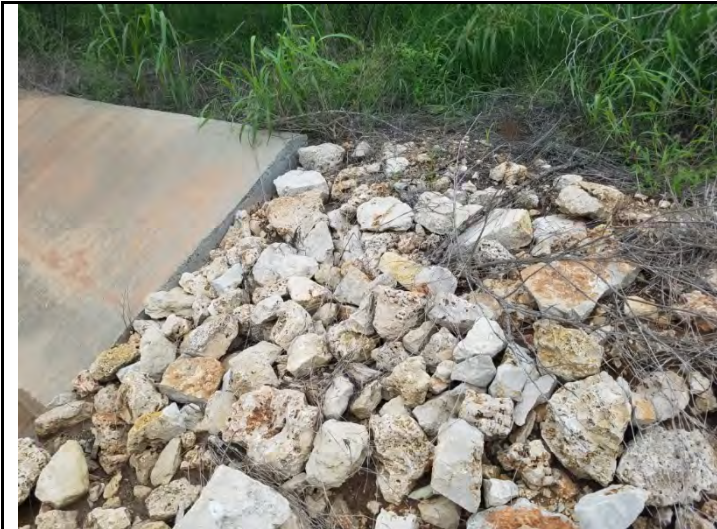
19 – Drainage channel, viewing slight erosion on Southwest corner
