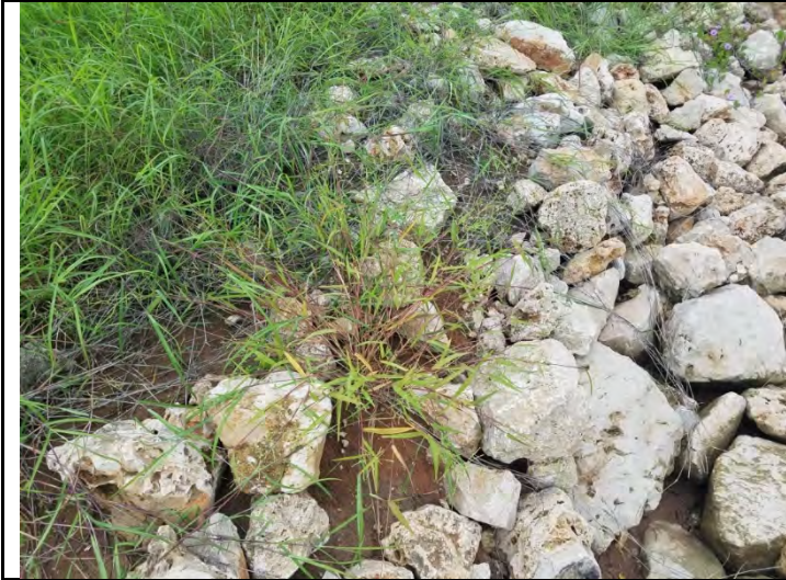
13 – Drainage channel, viewing some slight movement and buildup of sediment
