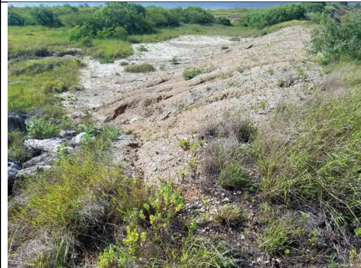
33 – East CPA Outer Dike, viewing erosion
