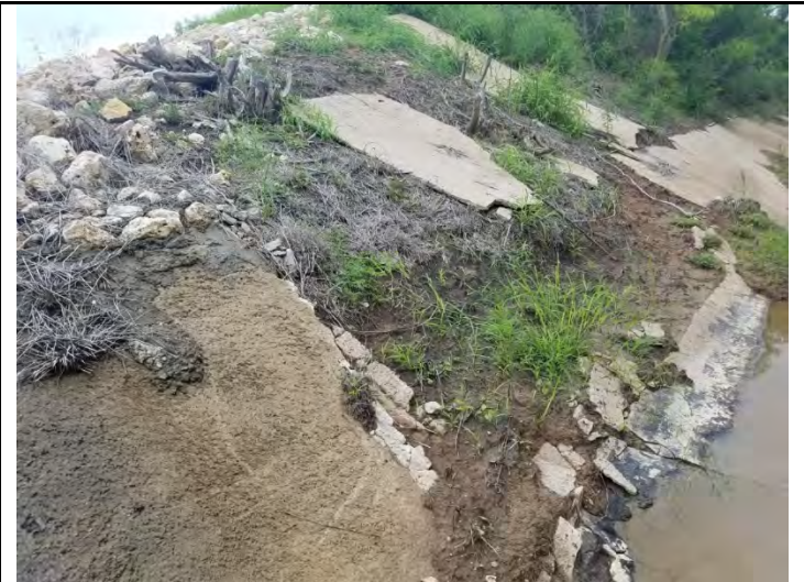
8 – Drainage channel, viewing deterioration of old channel
