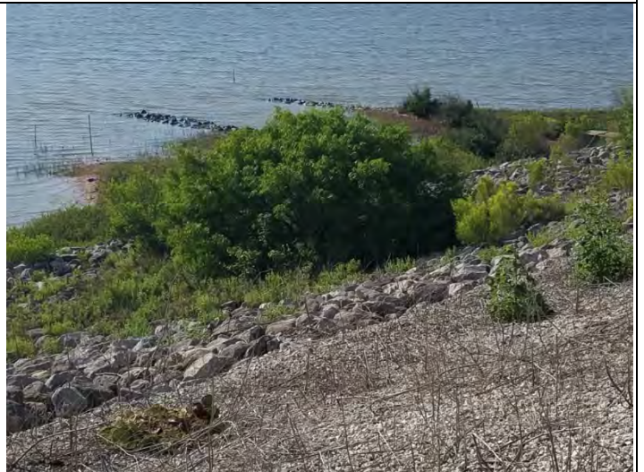
12 –East Outer Dike - vegetation at the bottom of the gravel protection and in the armor
