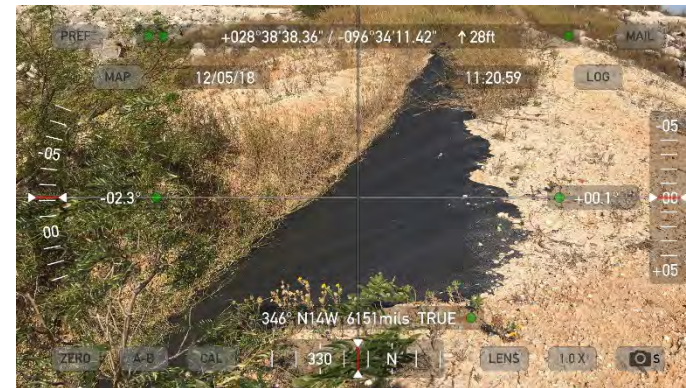
Port CDF Erosion/Exposed FML at East Water Stop - Interior
