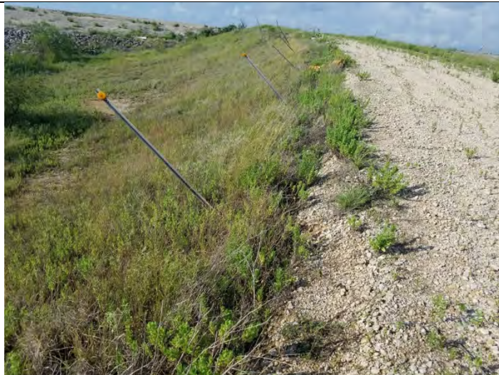
3 – North Ramp, viewing washout and cracking
