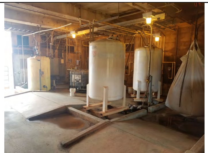
16 – R301, viewing system – carbon canisters
