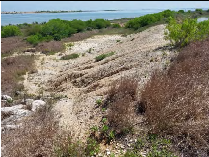
33 – East CPA Outer Dike, viewing erosion
