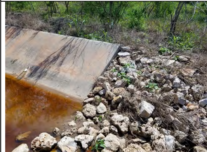
23 – Drainage channel, viewing slight erosion on Southwest corner
