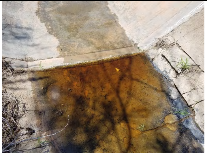
8 – Drainage Channel, viewing seam between old and new channel
