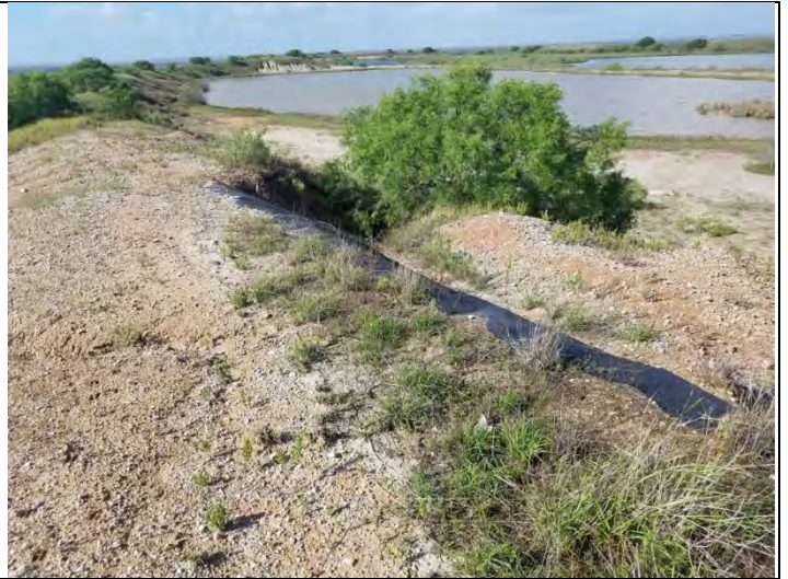
32 – East CPA Inner Dike, viewing erosion and exposure of liner
