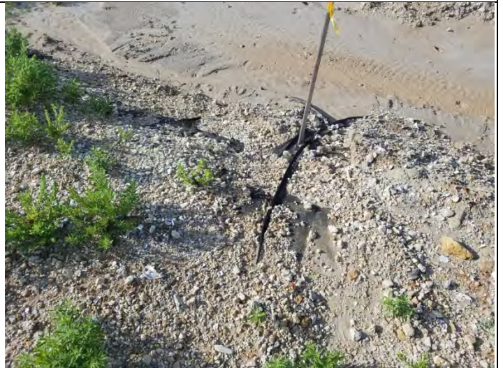
4 – North Inner Dike, viewing exposed geofabric
