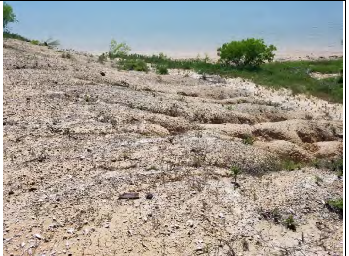
34 – West CPA Outer Dike, viewing erosion
