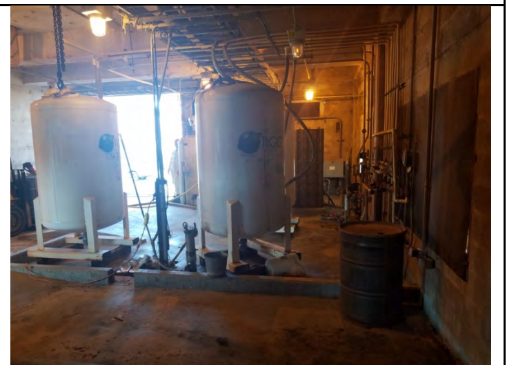
18 – R301, viewing system – carbon canisters
