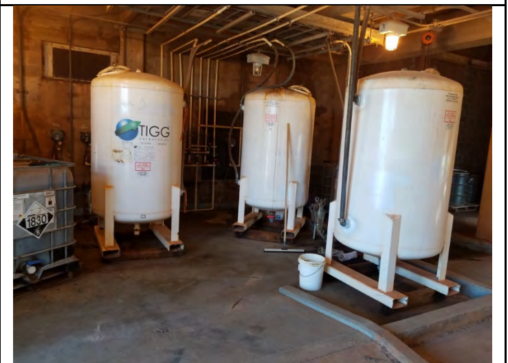
18 – R301, viewing system – carbon canisters
