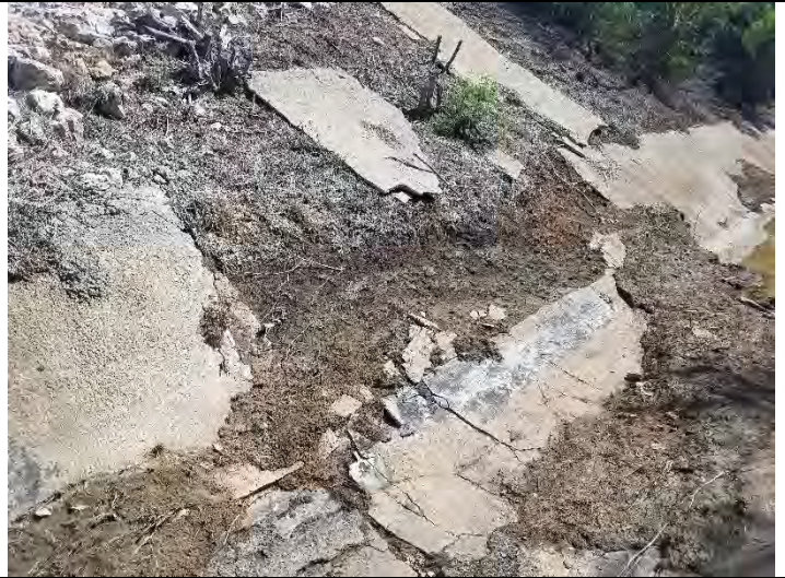
10 – Drainage channel, viewing deterioration of old channel
