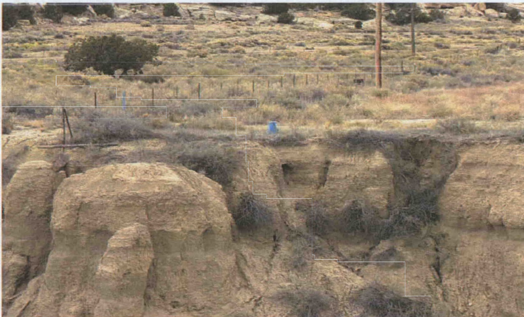
Photograph 4: North view across Pipeline Arroyo, shows the close proximity of Well GW-3 (north side) to the severely eroded and sloughed embankment, prohibiting sampling due to safety concerns.
