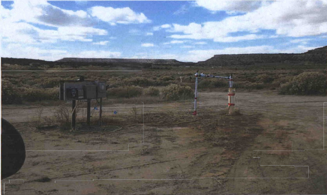
Photograph 7: North view across the northwest ground water remedial action area, that shows the Zone 3 ground water extraction wells.
