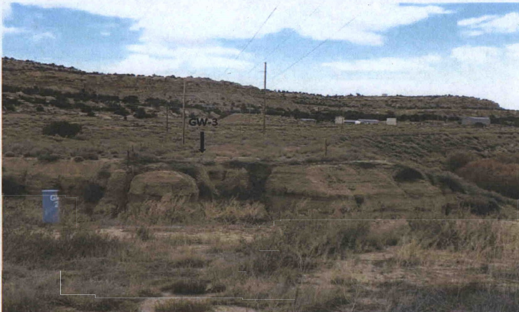
Photograph 3: North view across Pipeline Arroyo, shows the close proximity of Wells GW-2 (south side) and GW-3 (north side) to the severely eroded and sloughed embankments.
