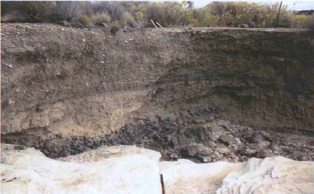
Photograph 6: Southeast view of a bend in Pipeline Arroyo at the “Nick Point”, that shows the continual undercutting and erosion of the embankment.
