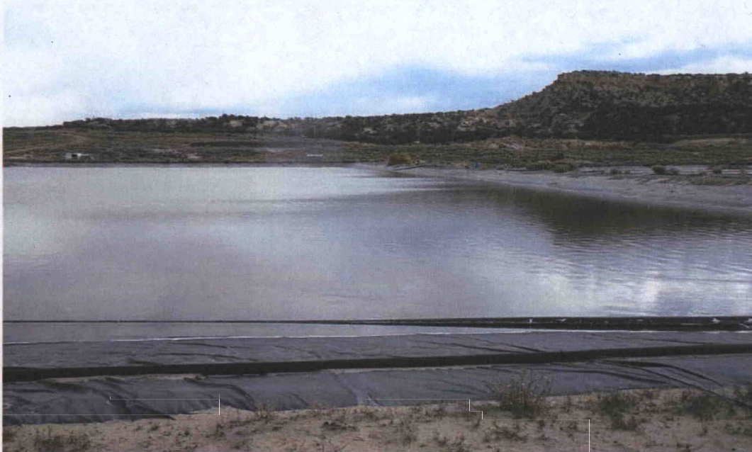
Photograph 2: Southeast view across the lined evaporation ponds on the south cell. Ponds contain mostly supplemental water from the facility supply well, and less than 5 percent from ground water extraction.
