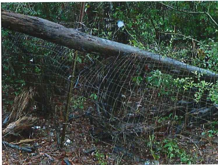
Border fence near UA-10 with damage from a fallen tree
