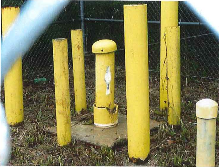
Well DA-02, with faded label and missing cover lock, well secured with locked plug
