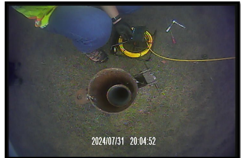
PS10A – well within stick up, camera equipment
