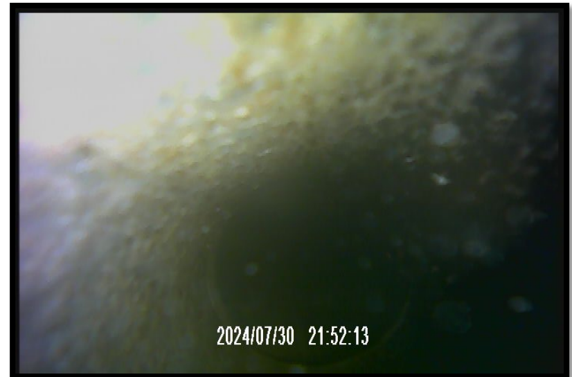
PSCD – reduced clarity, joint
