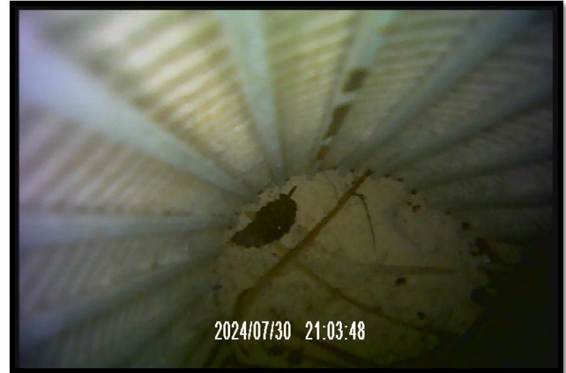
COP1 – bottom of well, clean screen
