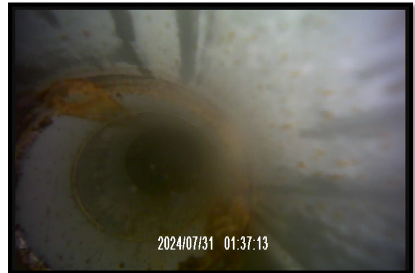
MW402S – some rusting on joint below water table
