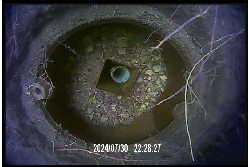
PS105D – well within flush mount
