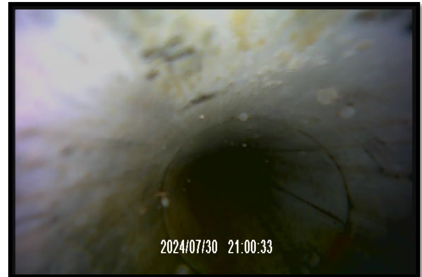
COP1 – joint beneath water table
