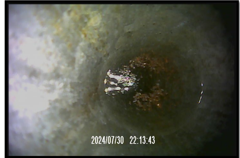
PS105S – water table above rusty joint
