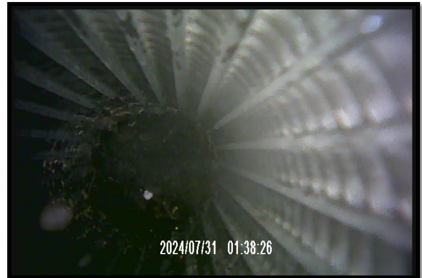
MW402S – screen in good condition
