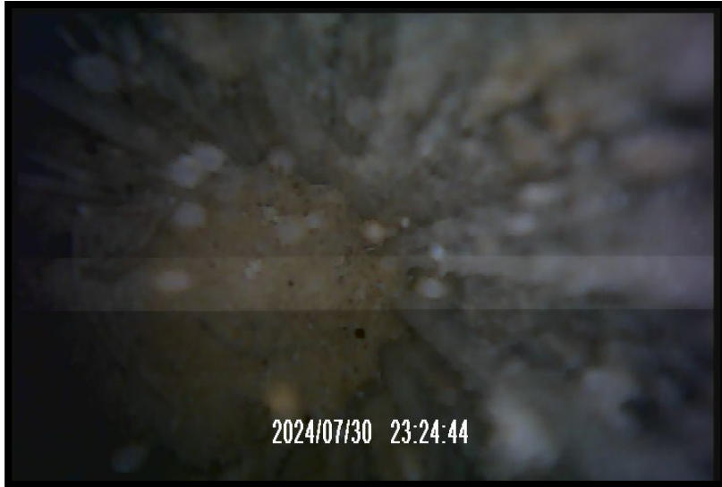
PS106 – bottom of screen, reduced clarity, calcite buildup still prevalent
