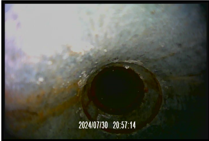
COP1 – casing and joint
