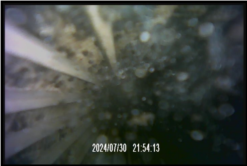
PSCD – screen has buildup near top
