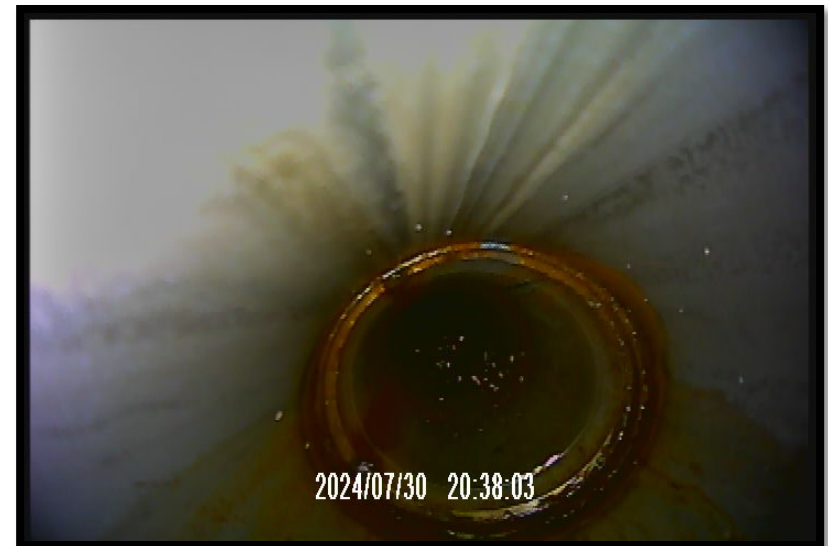
MW401S – joint / water table
