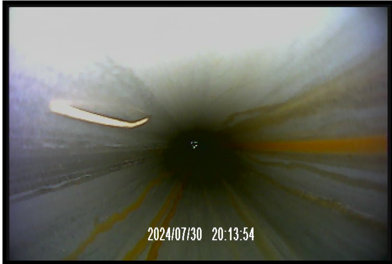
MW401D – Casing in good condition
