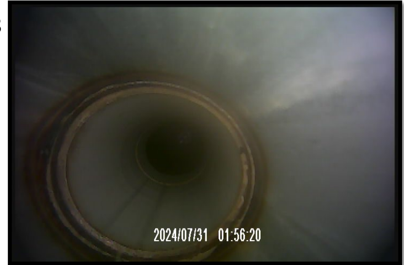
MW402D – joint in good condition
