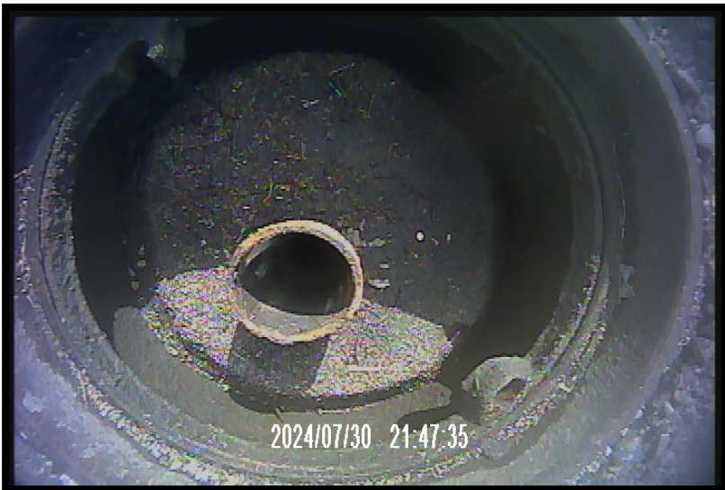
PSCD – Well within flush mount
