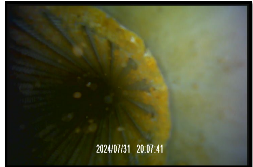
PS10A – off center, top of screen, rust
