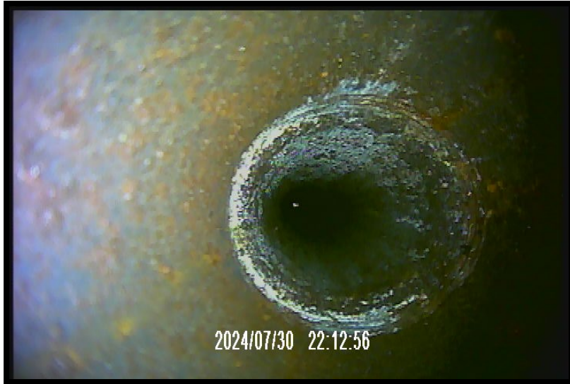
PS105S – joint with rust
