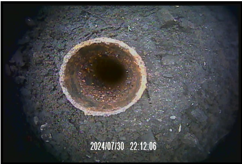
PS105S – rusty well within flush mount
