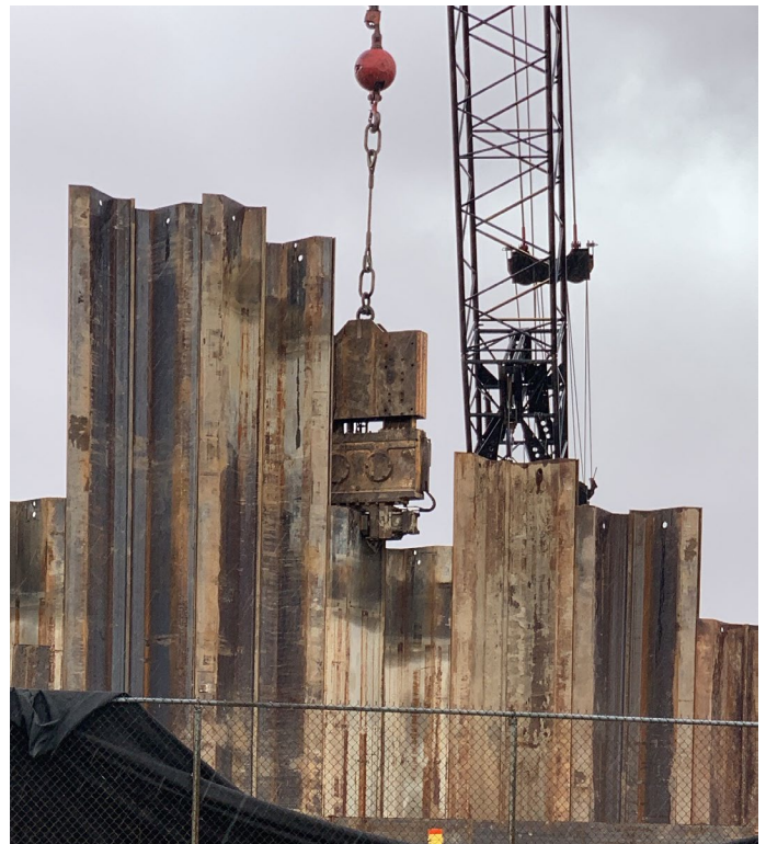
Photo of a vibratory hammer used to install sheet piles.
