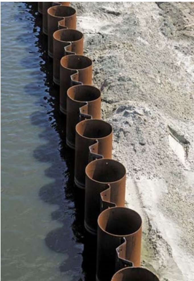
Photo of a sheet wall that looks similar to the one that will be installed at the Velsicol Site.
