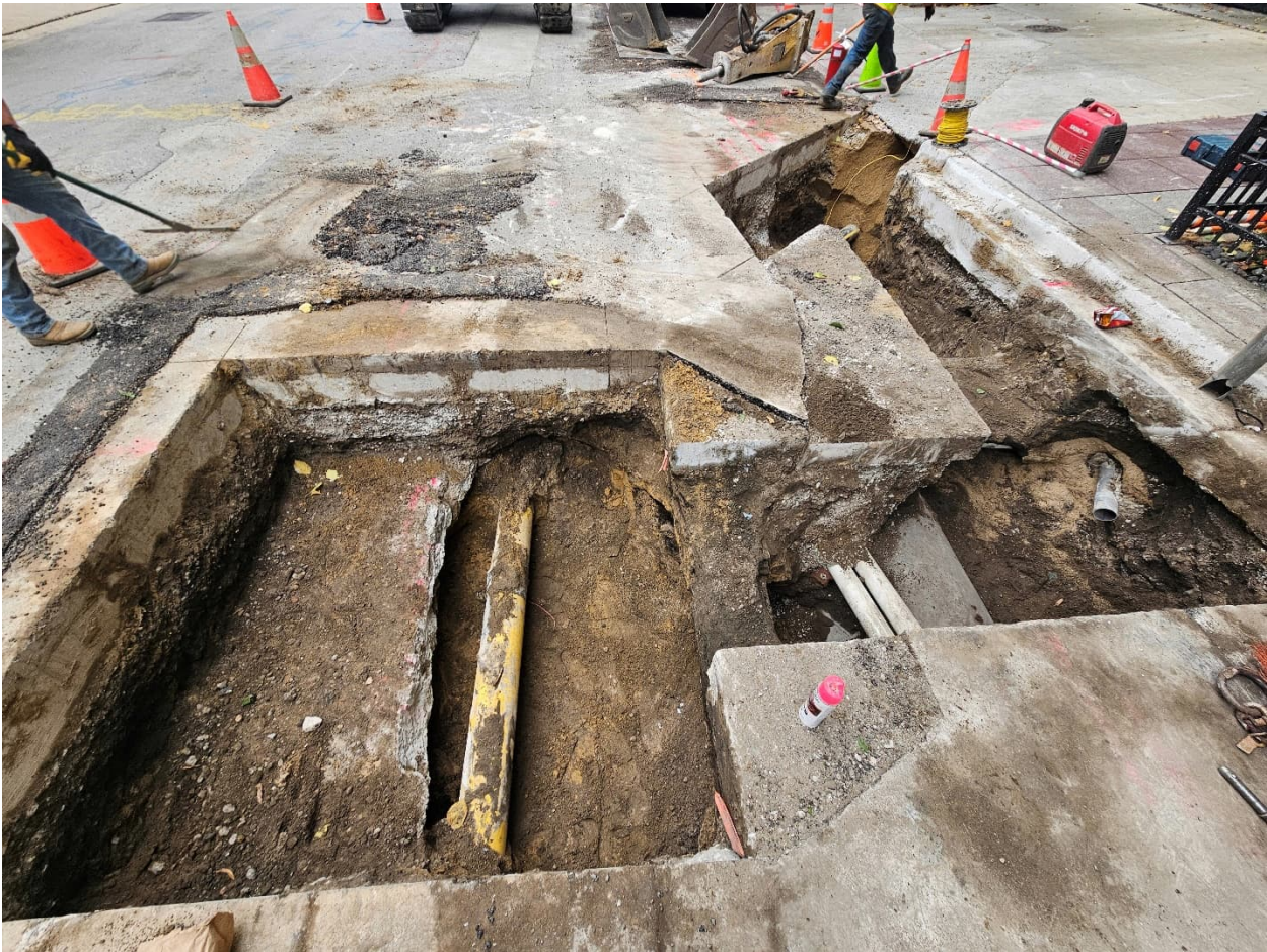
PICTURE 1: VIEW OF EXCAVATION FACING EAST, WESTERN END OF EXCAVATION.
