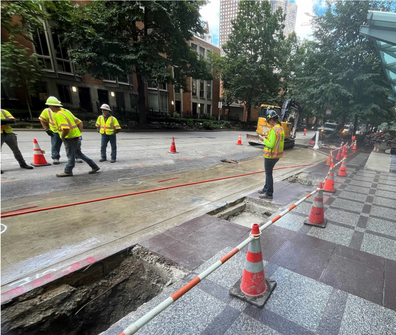
PICTURE 5: VIEW OF EXCAVATION ON SIDEWALK INFRONT OF 415 E NORTH WATER STREET CONDOS, FACING NORTHEAST.
