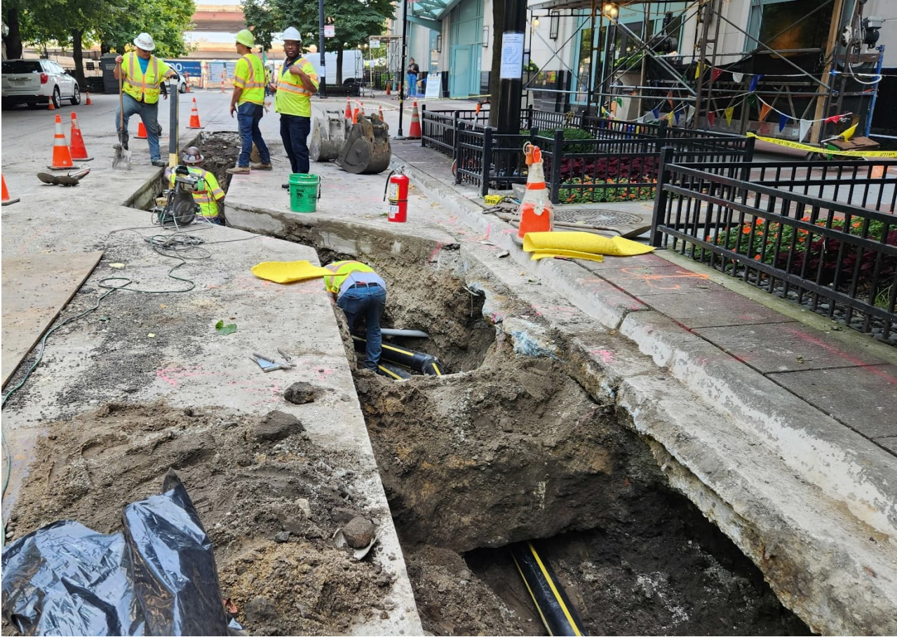
PICTURE 3: VIEW OF EXCAVATION RUNNING EAST TOWARDS 400 LSD
