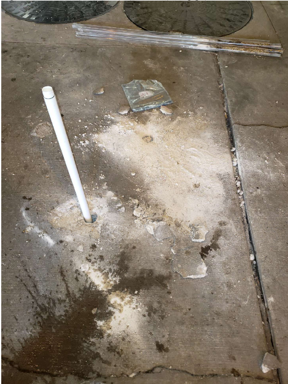
Figure 2: Holes B (BX) (middle) and B' (with pipe)
