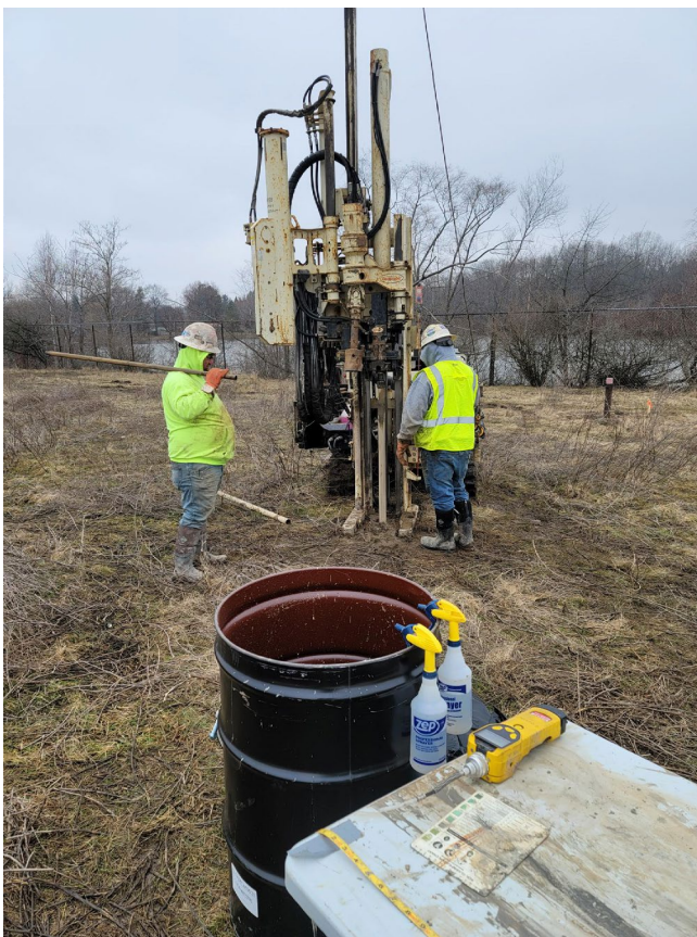
Workers drilling a soil boring from the MW-19 area.
