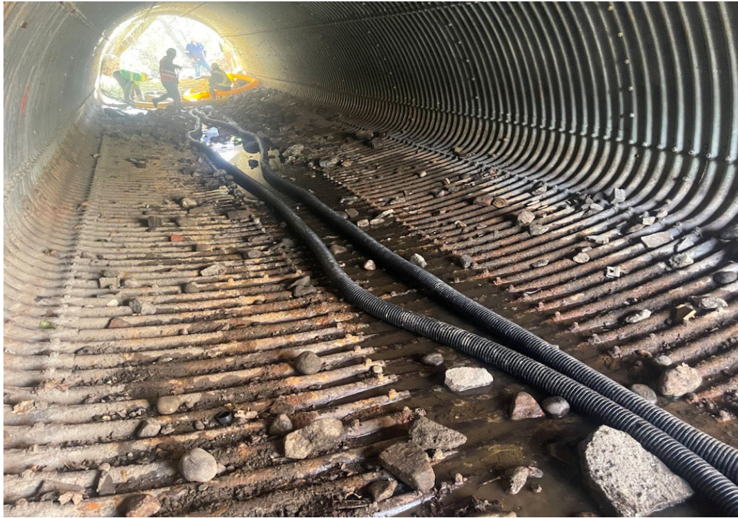
Photograph: 9 Description: Culvert C4 after cleaning. Date: 11/16/2023 Location: C4
