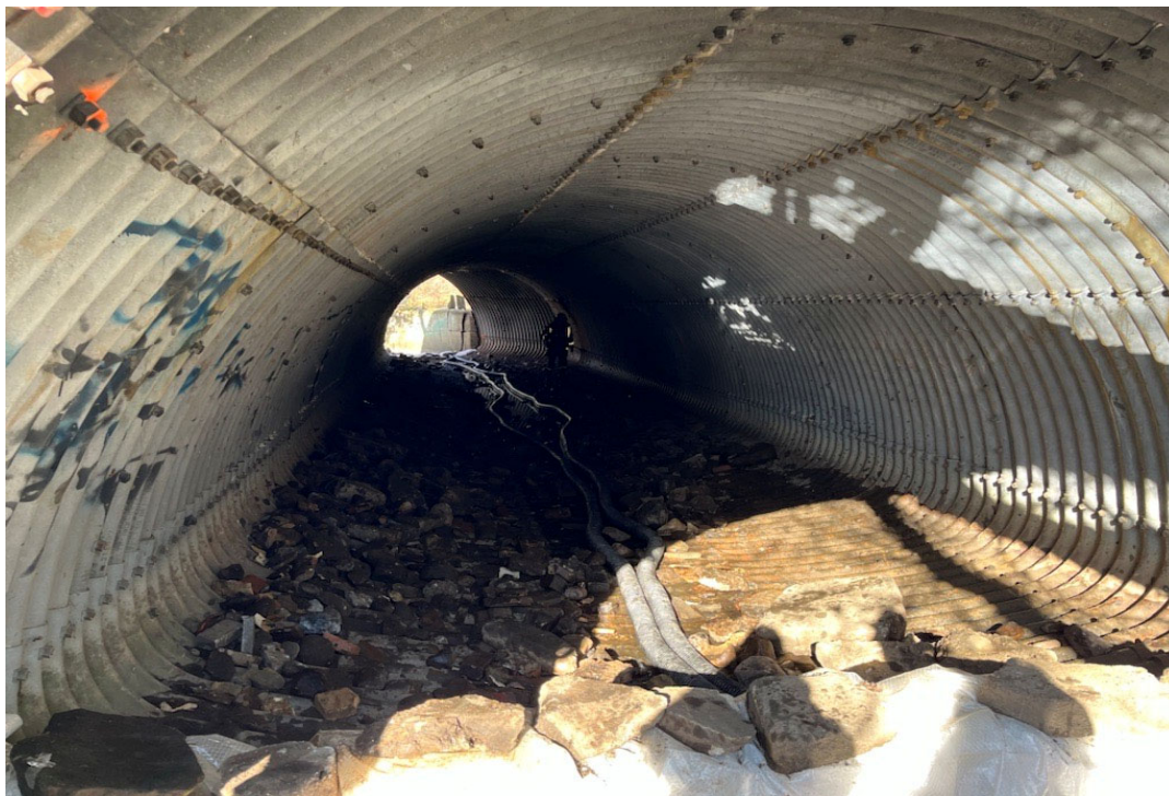
Photograph: 10 Description: Culvert C4 after cleaning. Date: 11/16/23 Location: C4
