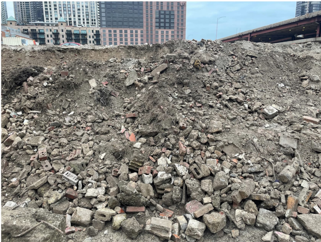
PICTURE 2: VIEW OF SIDE TRENCH 4 AND EXCAVATION SPOIL MATERIAL COMPOSITION - 400 N LSD LOOKING NORTH
