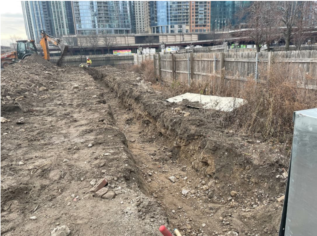
PICTURE 5: VIEW OF TRENCHES 9, 10 AND 11 - 400 N LSD LOOKING SOUTH
