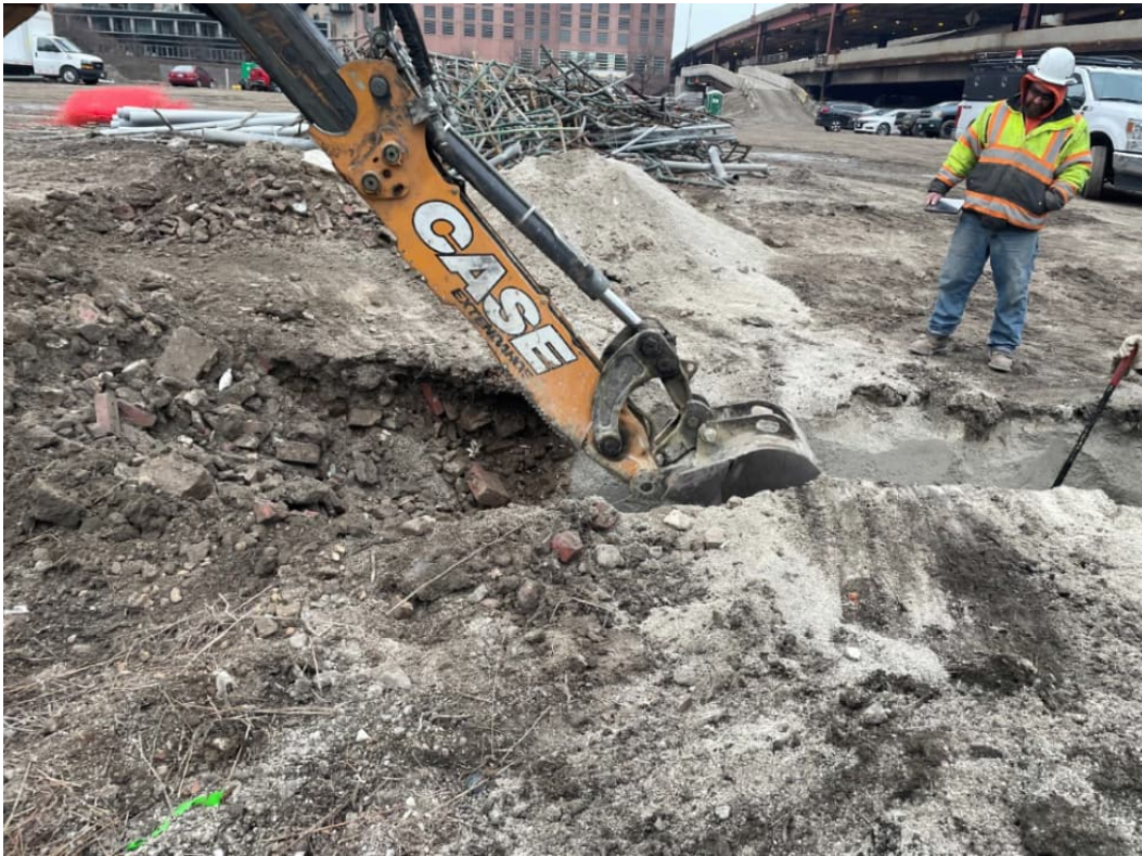
PICTURE 2: VIEW OF SIDE TRENCH 4 AND EXCAVATION SPOIL MATERIAL COMPOSITION - 400 N LSD LOOKING NORTH
