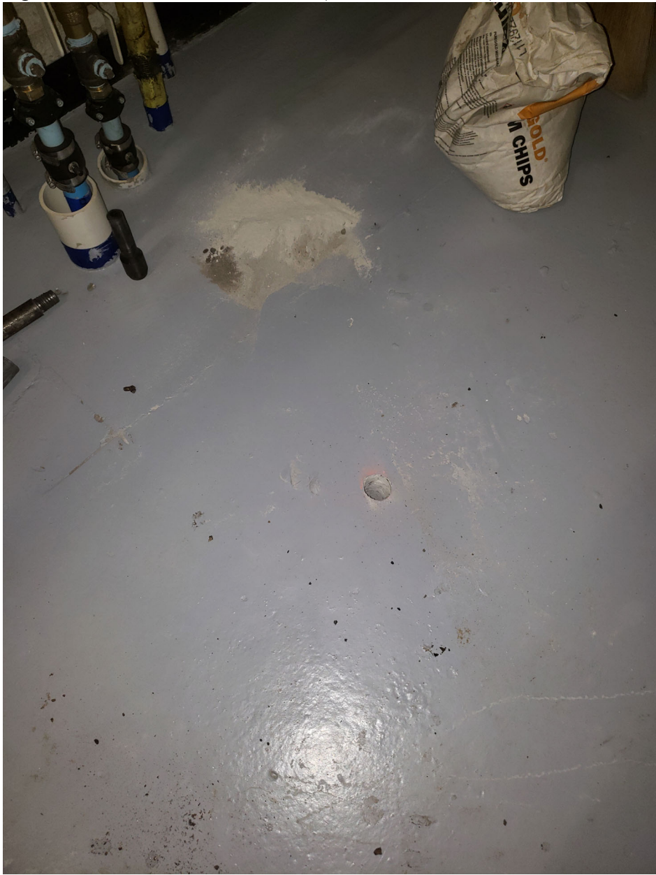
Figure 2: Generator room borehole (north to lower left)
