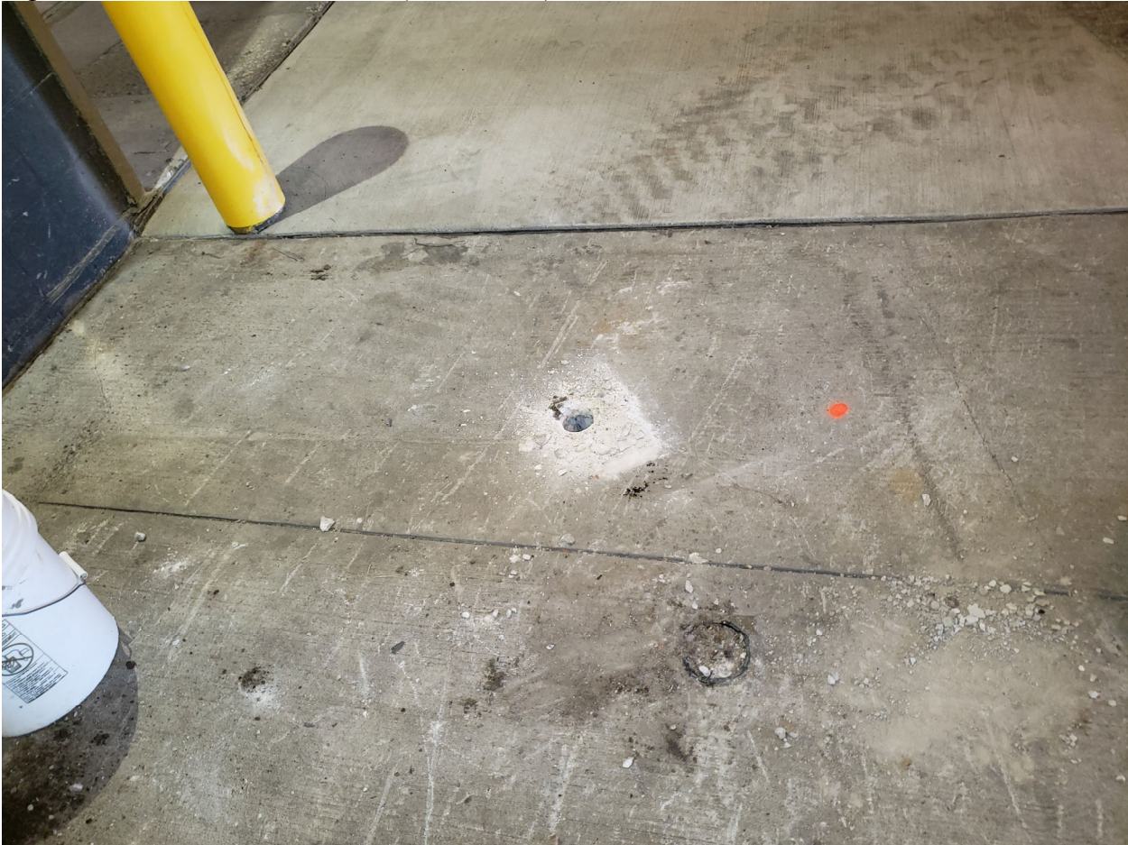
Figure 3: West sidewalk borehole (north to left)
