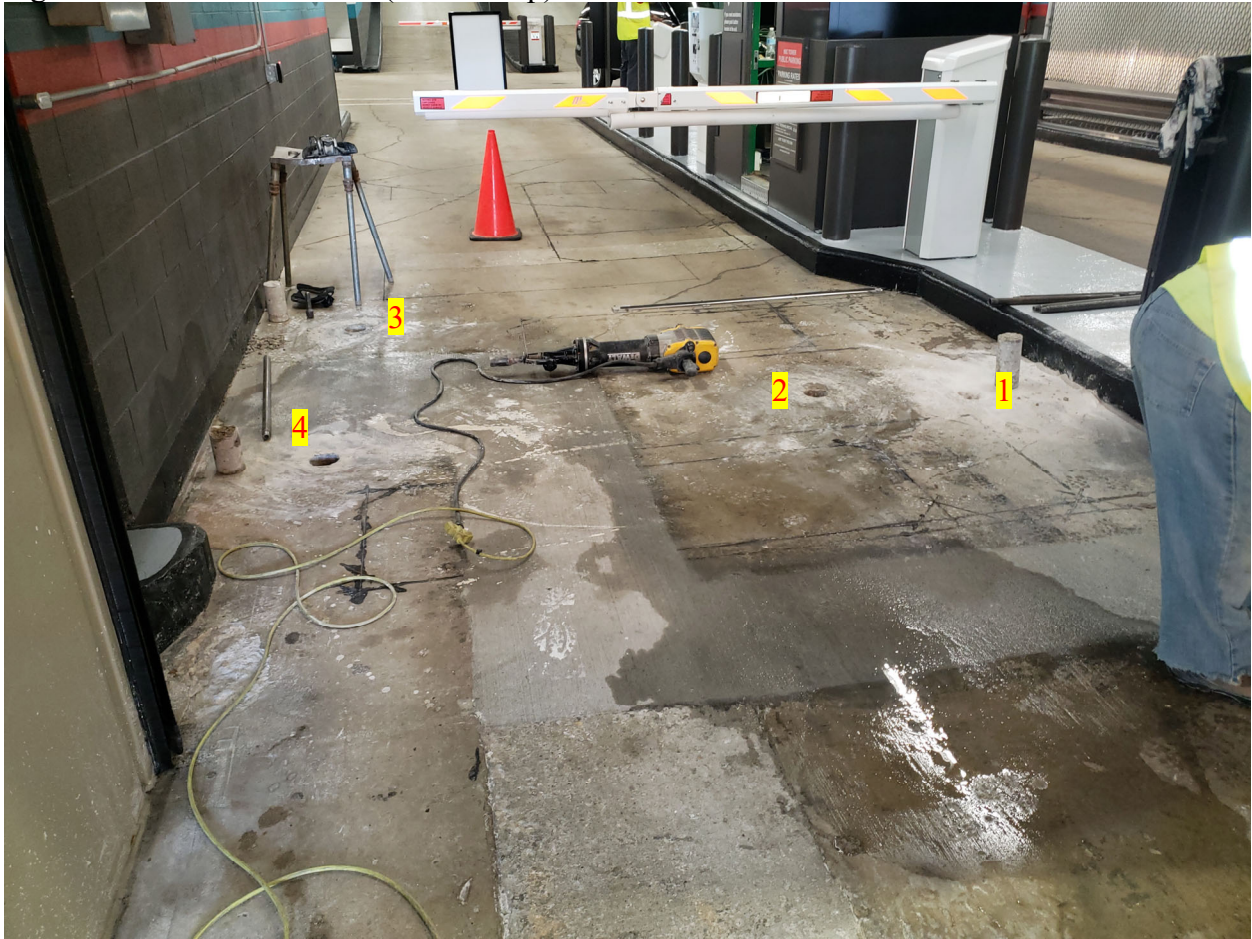
Figure 5: Exit lane boreholes (north to top)
