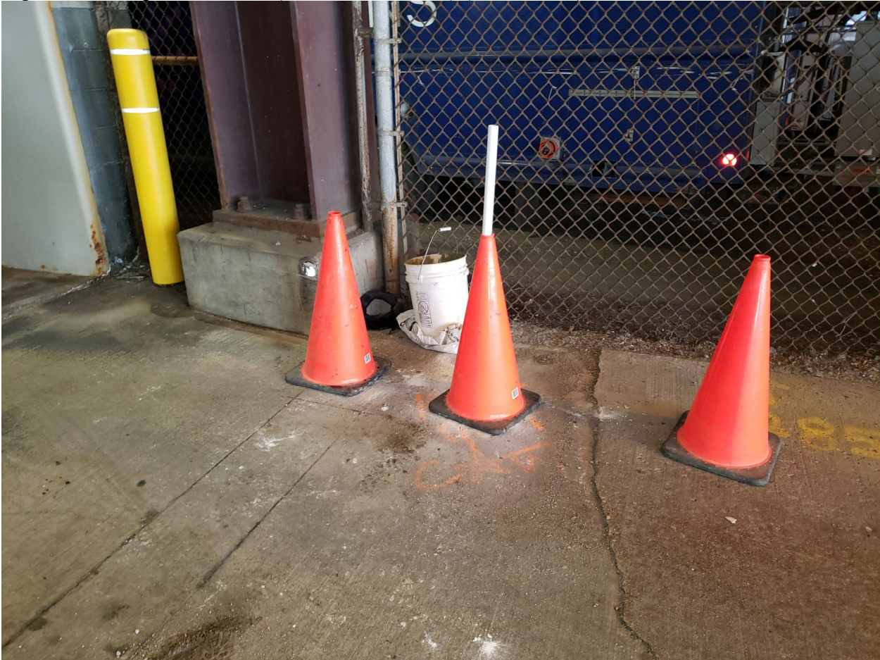
Figure 6: East apron borehole (under middle cone) (north to left)
