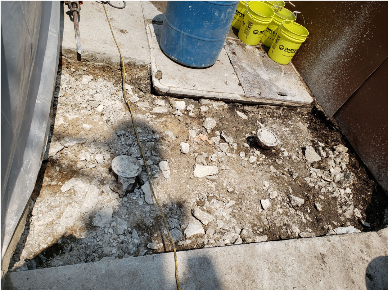
Figure 2: Area 1 and 1 B (north is to the top of the photograph)
