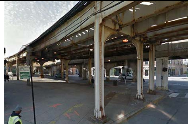
RPM-SB-15 boring location, facing southwest
