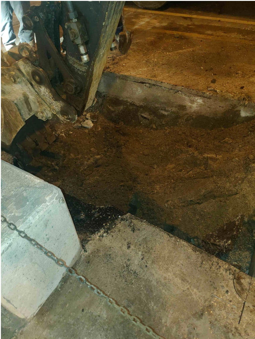
PICTURE 1: SOUTHWEST-FACING VIEW OF EXCAVATION AT 435 N LOWER MICHIGAN AVE.
