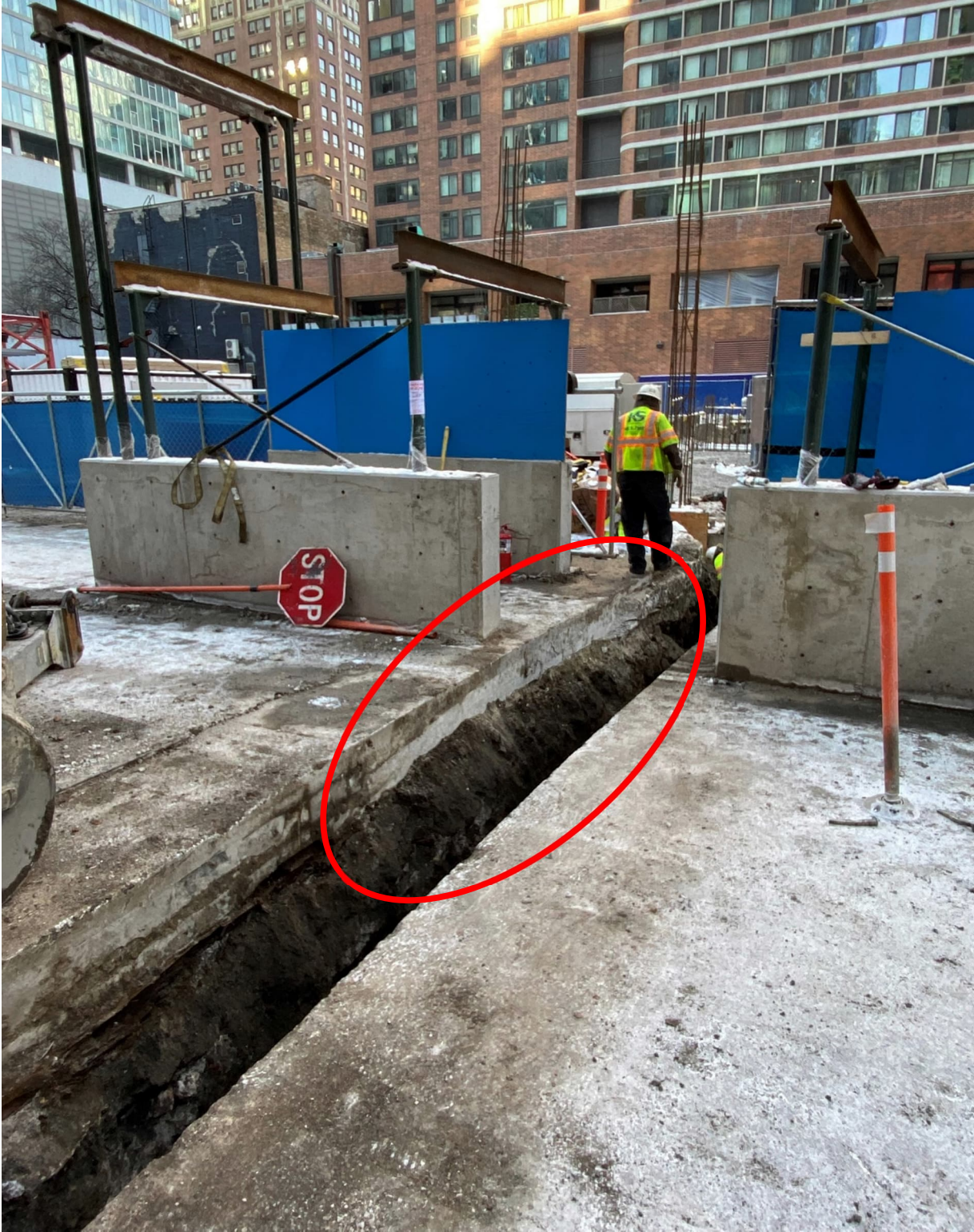
PICTURE 3: NORTH-FACING VIEW OF COMPLETED EXCAVATION OF SECTION 4 AT 210-225 E. GRAND AVE.
