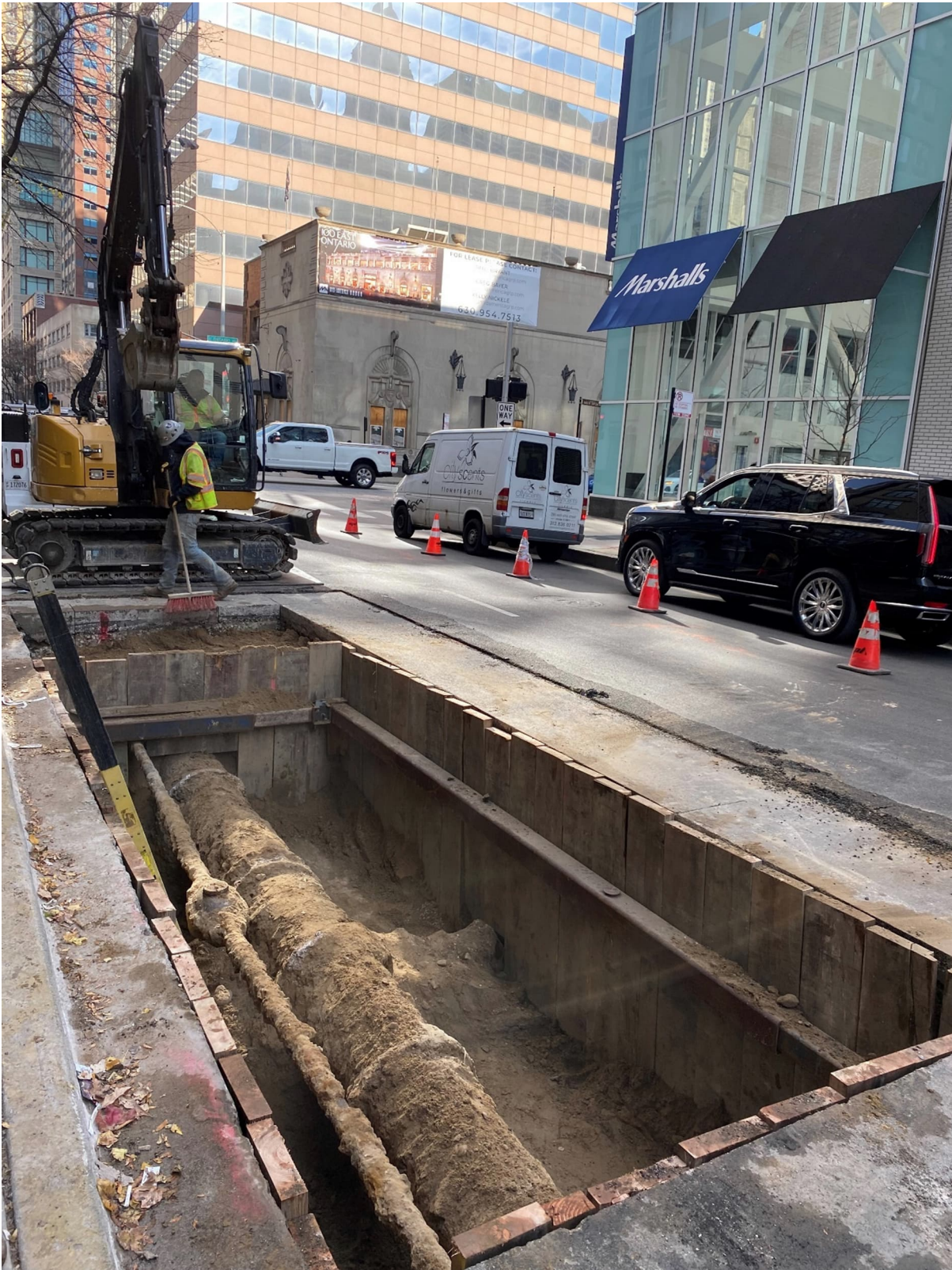
PICTURE 1: VIEW OF THE COMPLETED EXCAVATION AT 612-621 N. RUSH ST.
