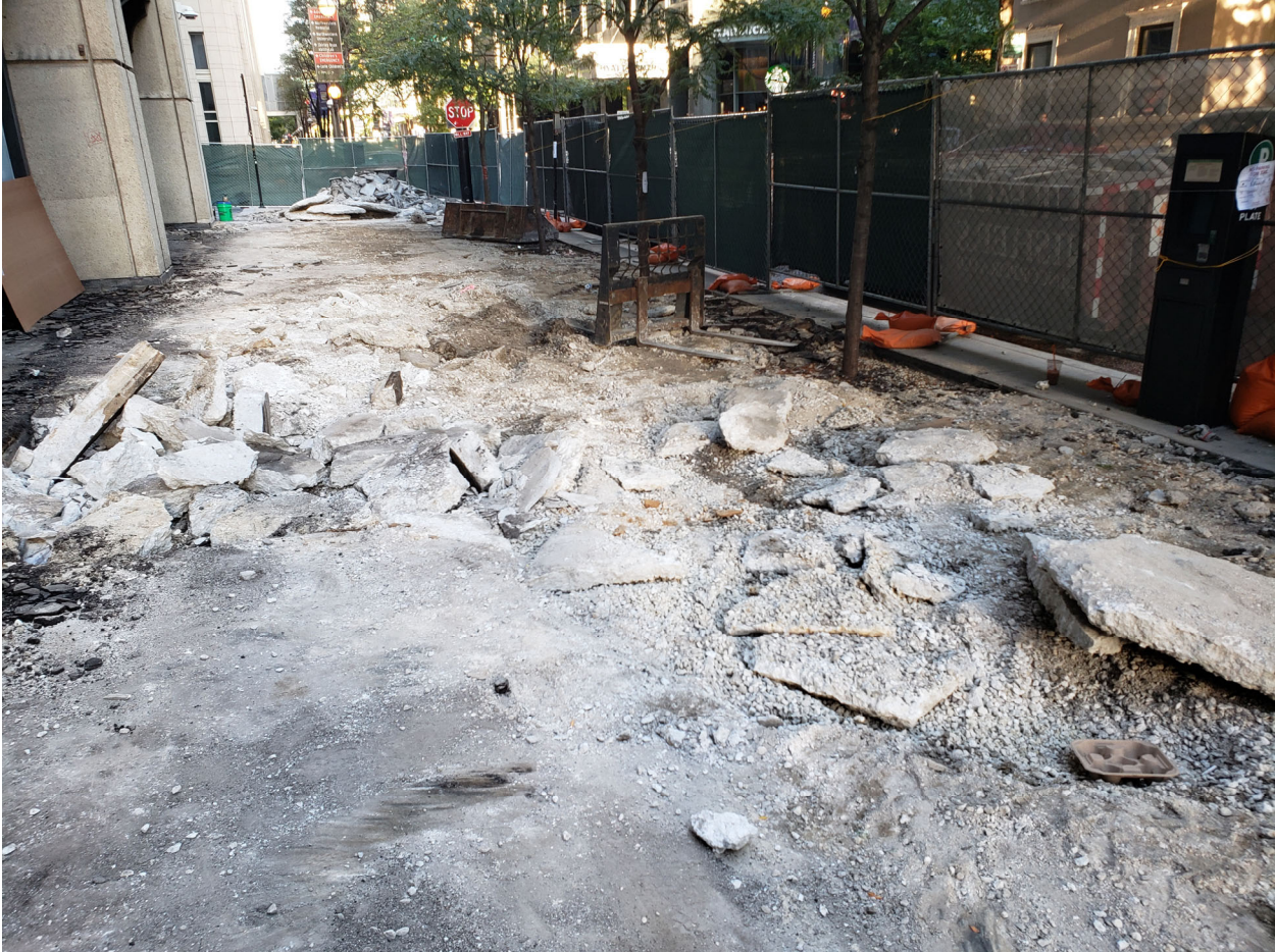
Figure: Area E-Broken, looking east
