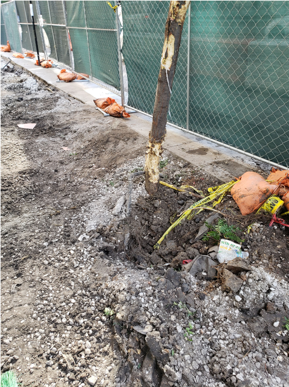
Figure: Tree 4, partially excavated around
