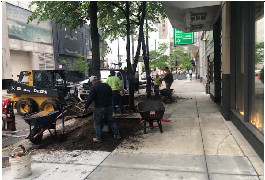
Photo 3: Looking south as Planter Area #3 is excavated after screening. 5/28/21
