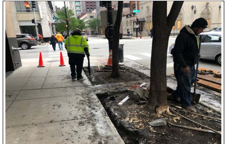
Photo 4: Looking North as Planter Area #5 is screened after concrete removal. 5/28/21
