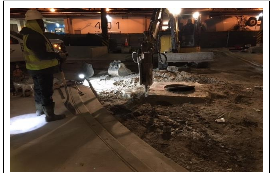
Photo 2: 1/14/2021 – Core Holes in extra concrete near manhole pad
