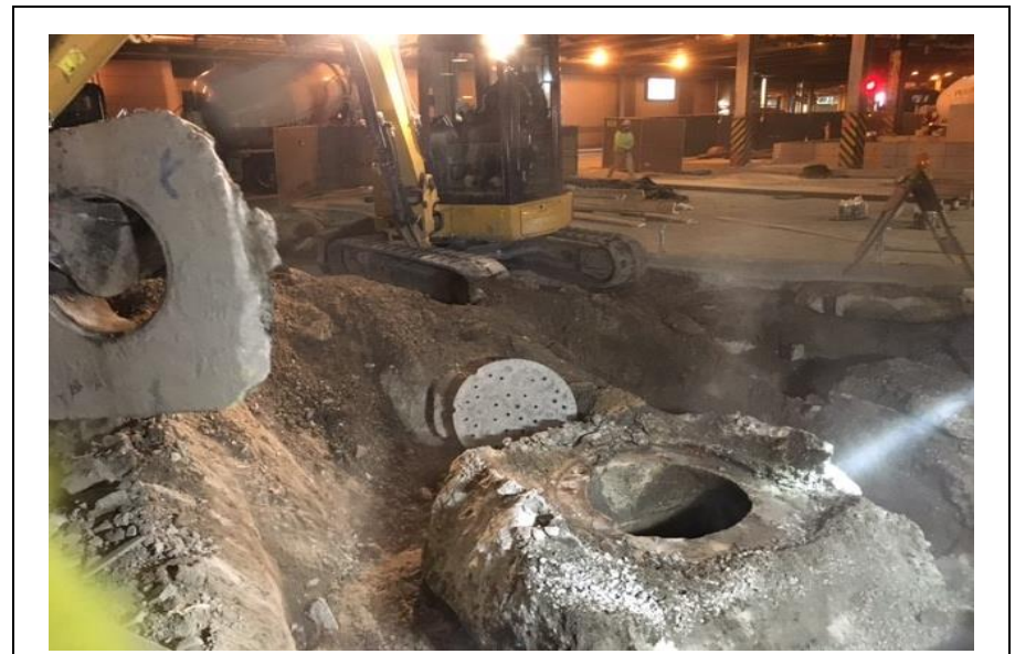
Photo 4: 1/14/2021 – Manhole Pad ready to be backfilled
