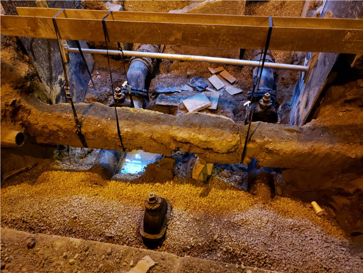
Figure 9: Water connection area, looking west, showing partially reburied utilities
