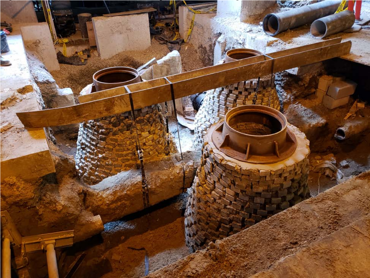
Figure 10: Water connection area, looking northwest, showing new vault construction
