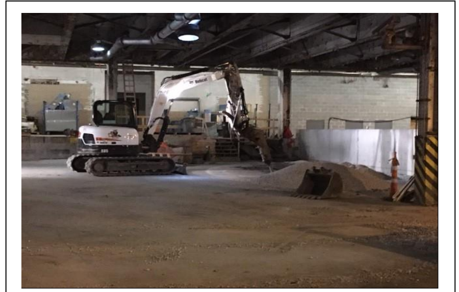
Photo 2: 12/24/2020 – Core Holes in Pavement using Jackhammer attachment
