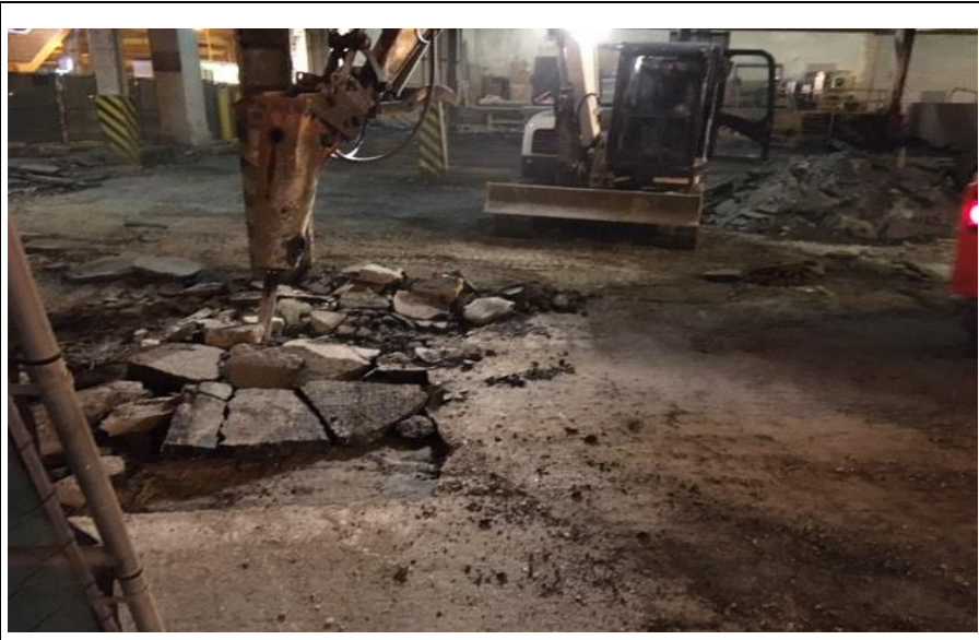
Photo 5: 12/29/2020 – RStrom hammered holes on Asphalt
