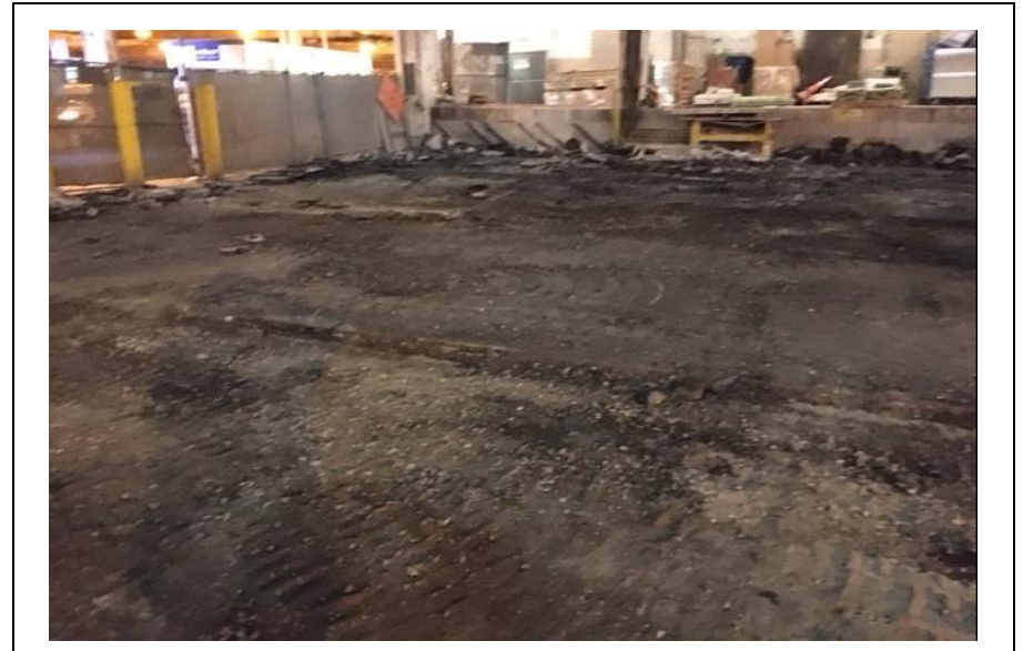
Photo 4: 12/28/2020 – 2 nd (underlying) Asphalt still present on Northern Half
