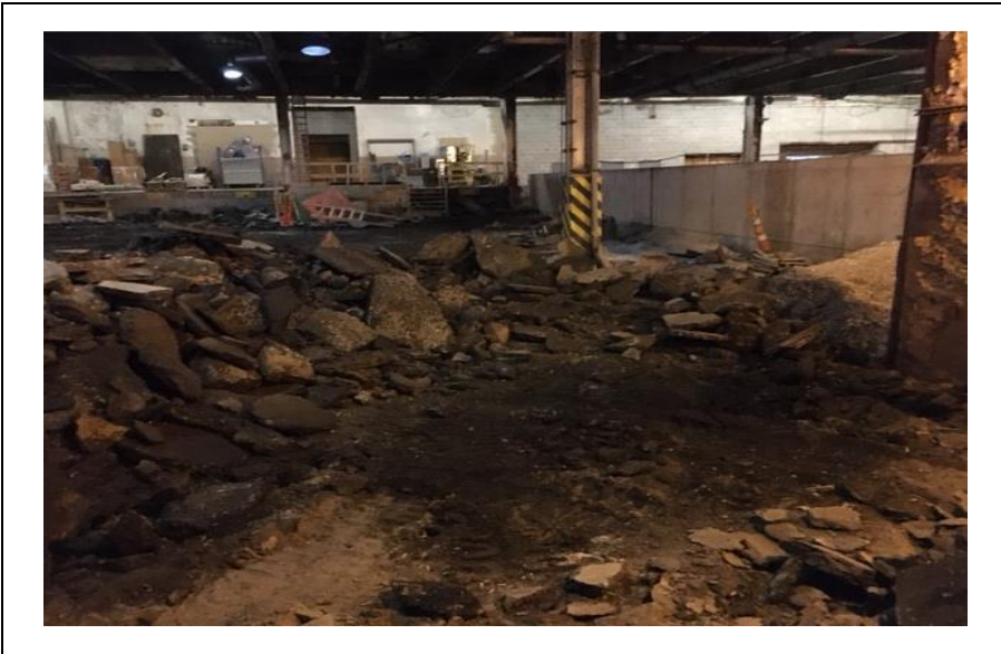
Photo 3: 12/28/2020 – Asphalt Removed from Southern Half of Work Area
