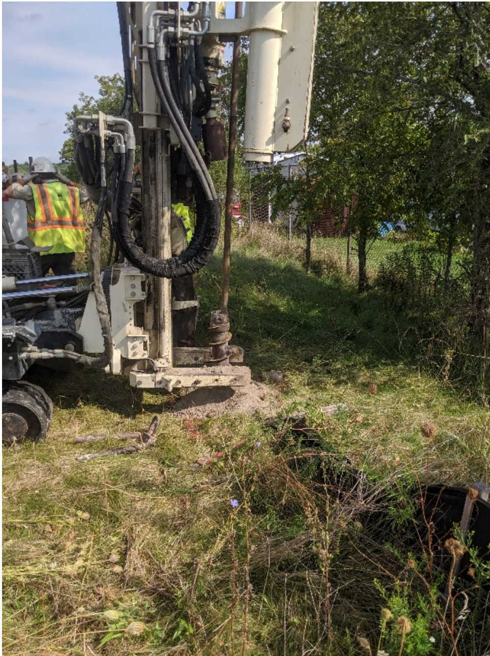
Photograph 5: CPZ-26 drilling activities (09-11-2019)
