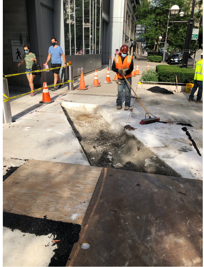
Looking west at sidewalk excavation in front of exit ramp.
