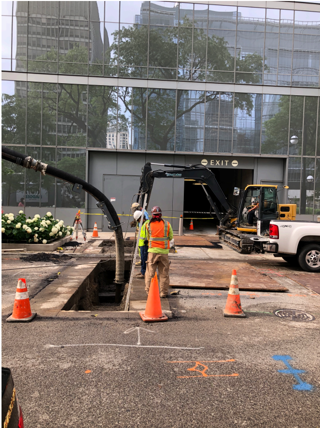
Looking south at excavation and 355 E. Erie St. building.
