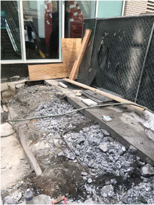
Sidewalk excavation area south of vault.
