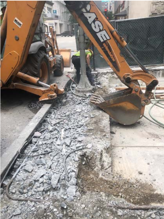
Western excavation area along N Rush St.
