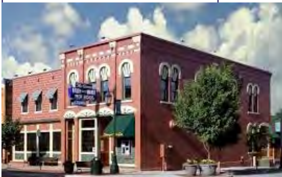
The Corner Bar in Rockford. https://www.tripadvisor.com/LocationPhotoDirectLink-g42646-d520665-i44220291-Corner_Bar-Rockford_Kent_County_Michigan.html .
