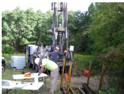
Contractors use a Geoprobe to collect soil samples on the Wolverine site.
