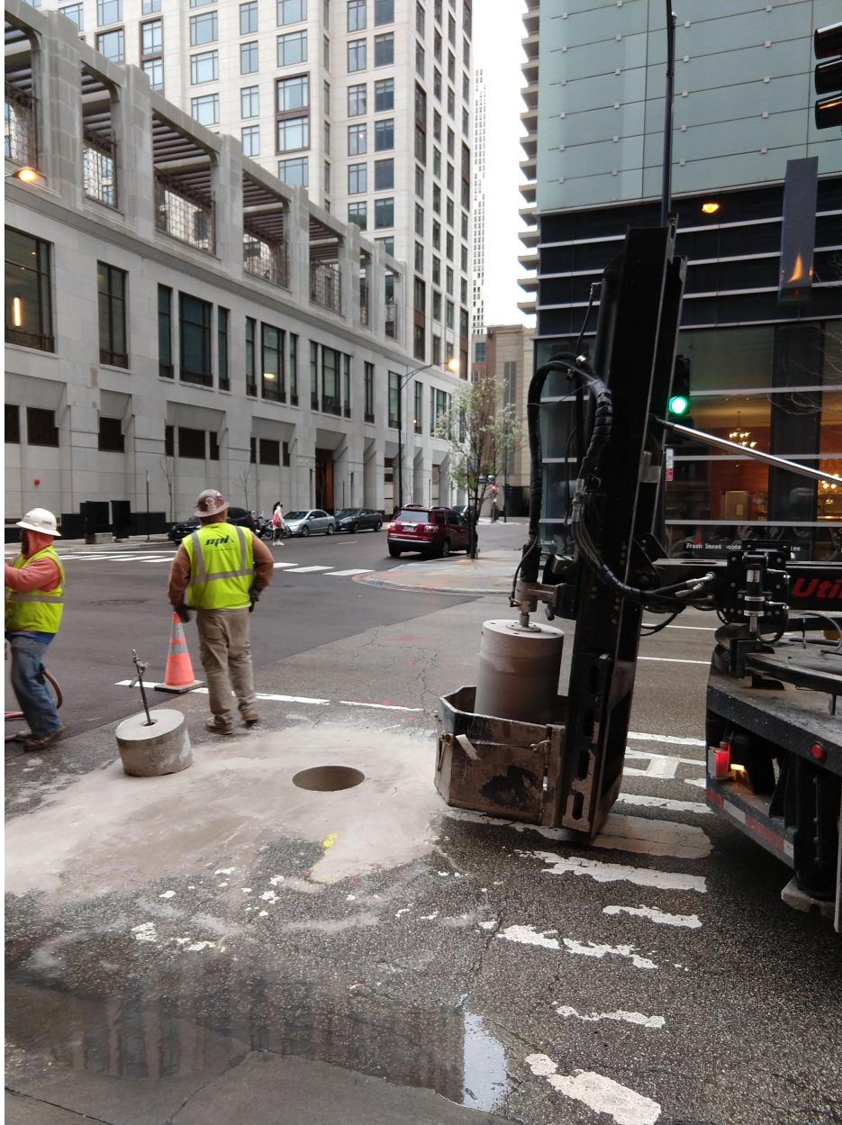
PICTURE 2: VIEW OF THE WEST KEYHOLE OPENINGS NEAR INTERSECTION OF PESHTIGO CT. THE THIRD KEYHOLE OPENING IS LOCATED APPROXIMATELY EIGHT FEET WEST (RIGHT IN THE PICTURE) OF THE KEYHOLE SHOWN ABOVE.
