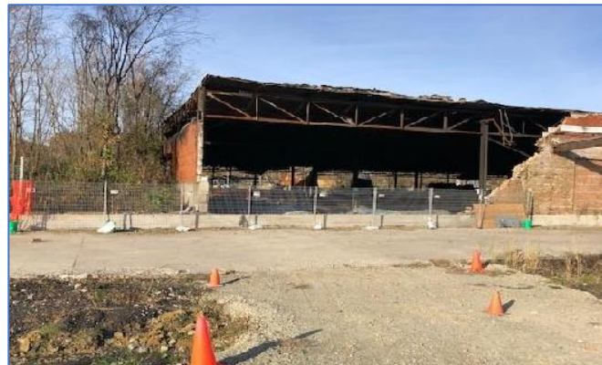
Fencing on the east side of the warehouse
