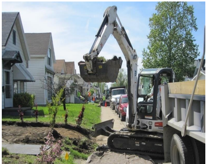
Figure 3: Typical excavation of contaminated soil.
