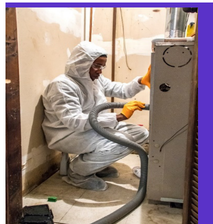
Interior dust cleaning.
