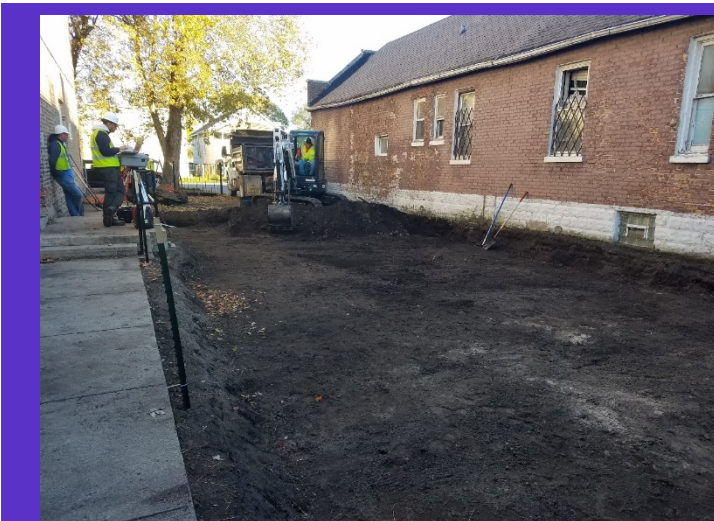
Clean fill replaces contaminated soil from yard.
