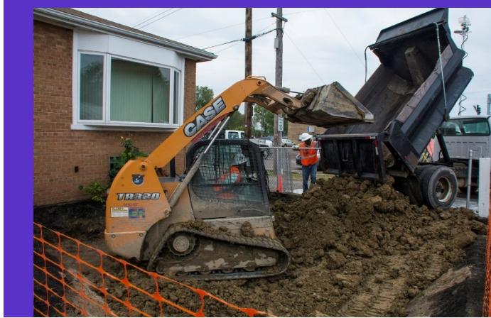
Soil being removed from yard.
